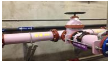
Reclaimed Water Supply Pipe at Howard County Fort Meade Reclaimed Water Pumping Station
