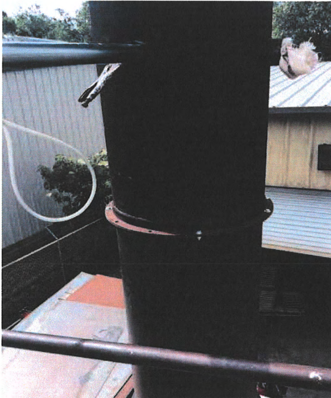
Photograph of Stack
