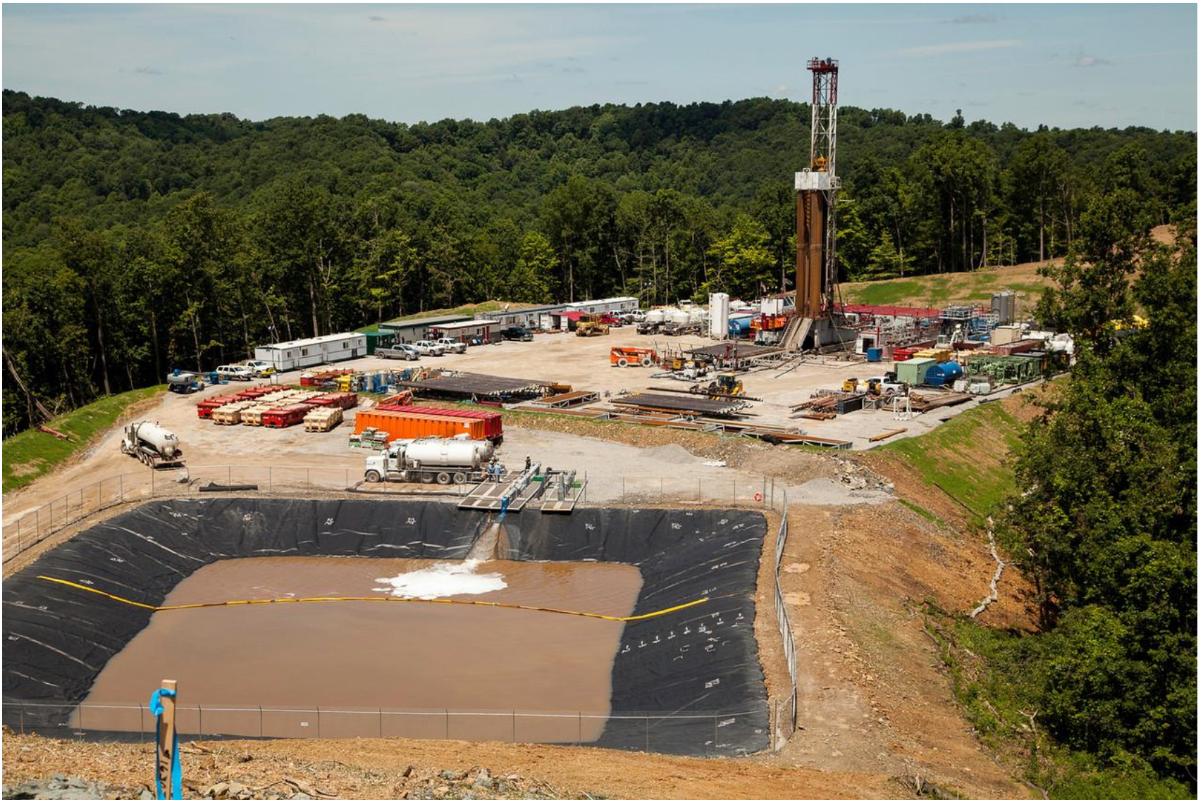
View of drill site from top of hill
