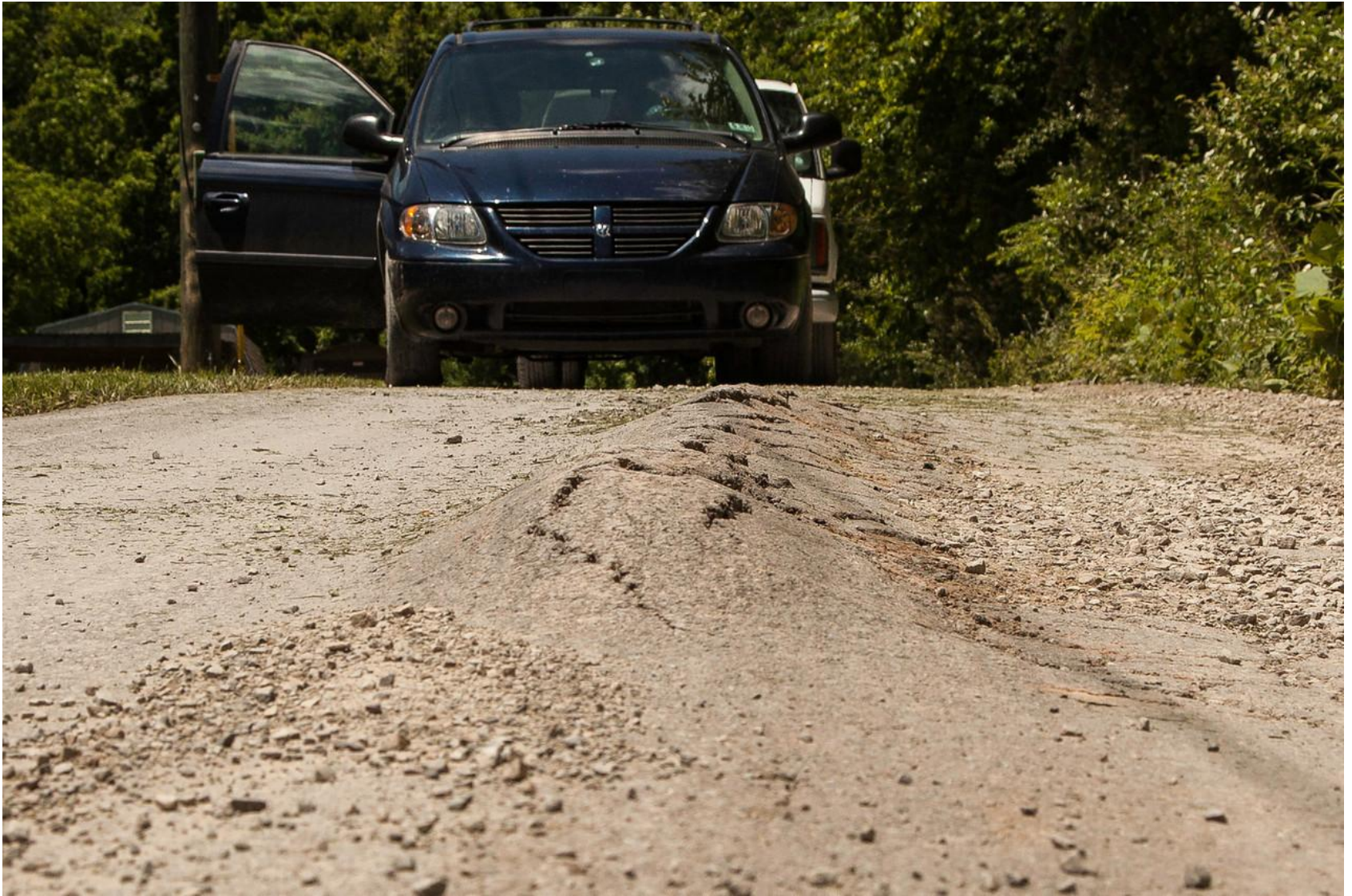
Buckled asphalt from truck traffic
