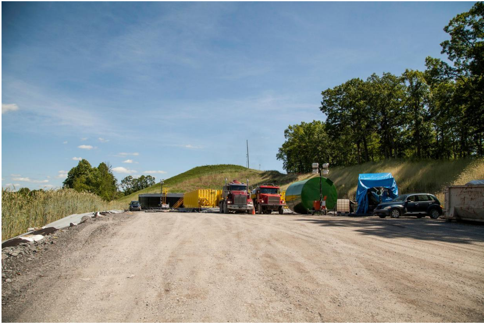
Vehicles and tanks at site, including 360 tank
