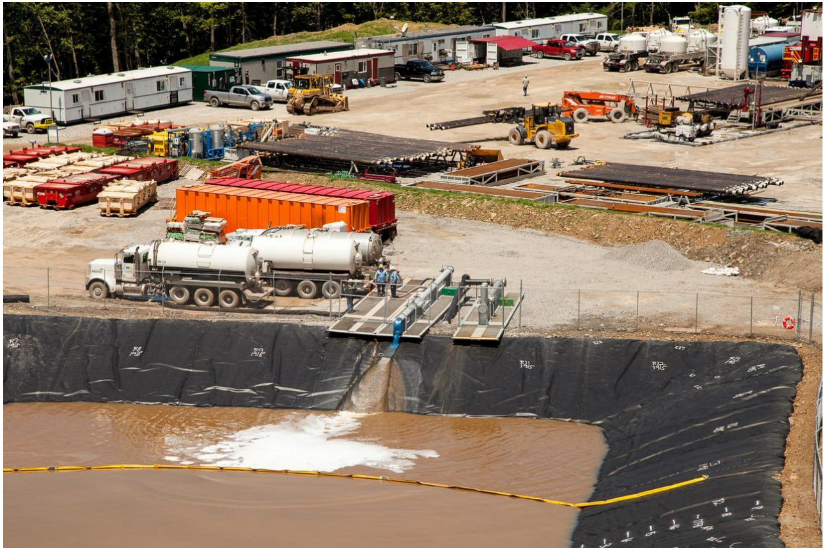
Same drill pad, adding water to storage pond.
