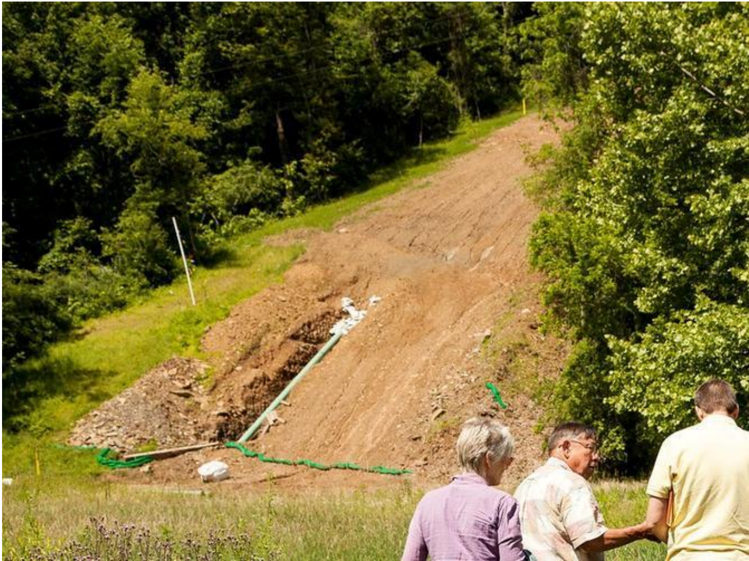
Pipeline installation at first stop
