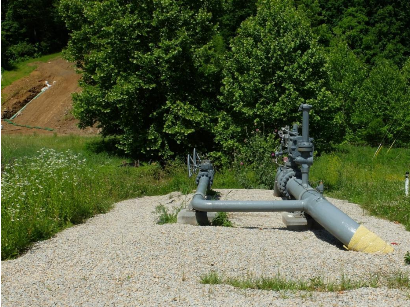
Newer pipeline and valves at first stop
