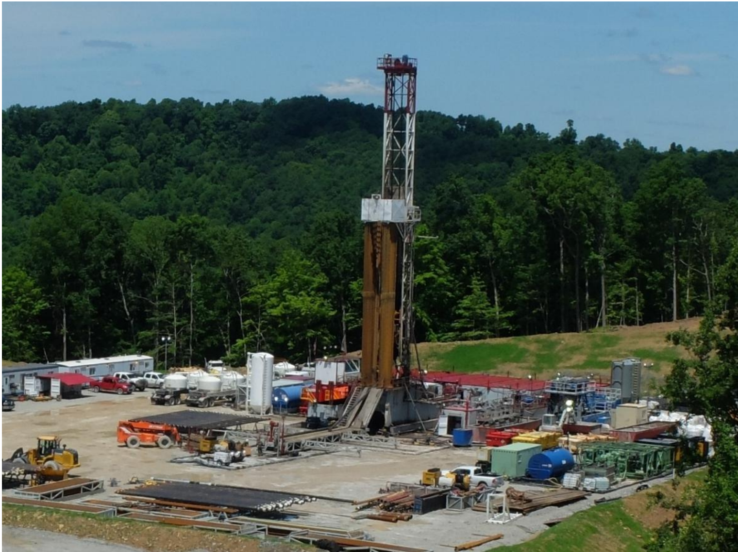
Same drill pad showing rig, pipes and other equipment
