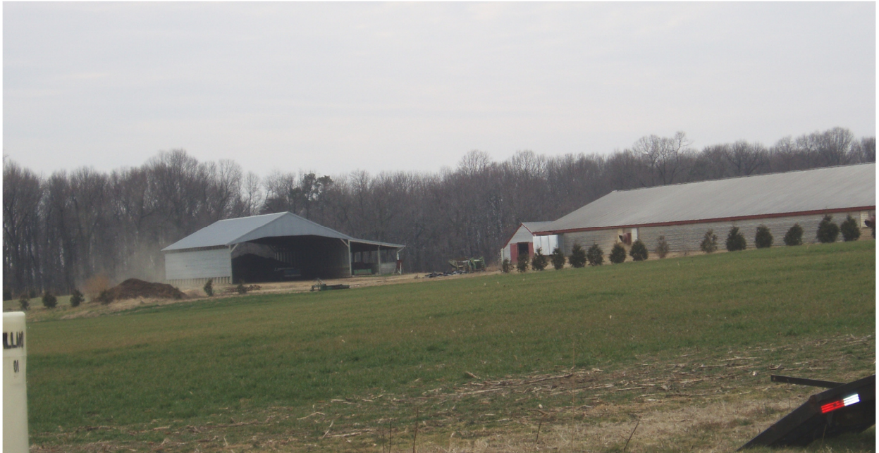
Manure Shed and Mortality Facility at the Loller Farm
