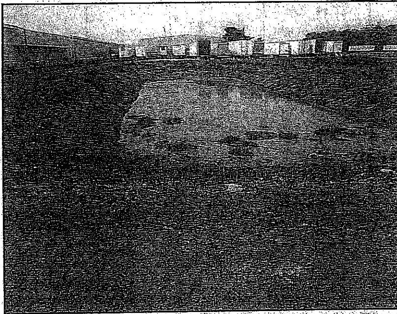
Egg wash, at the Millington Layer site, is captured in this style earthen storage. This water is later spray irrigated on grass areas or cropland.
