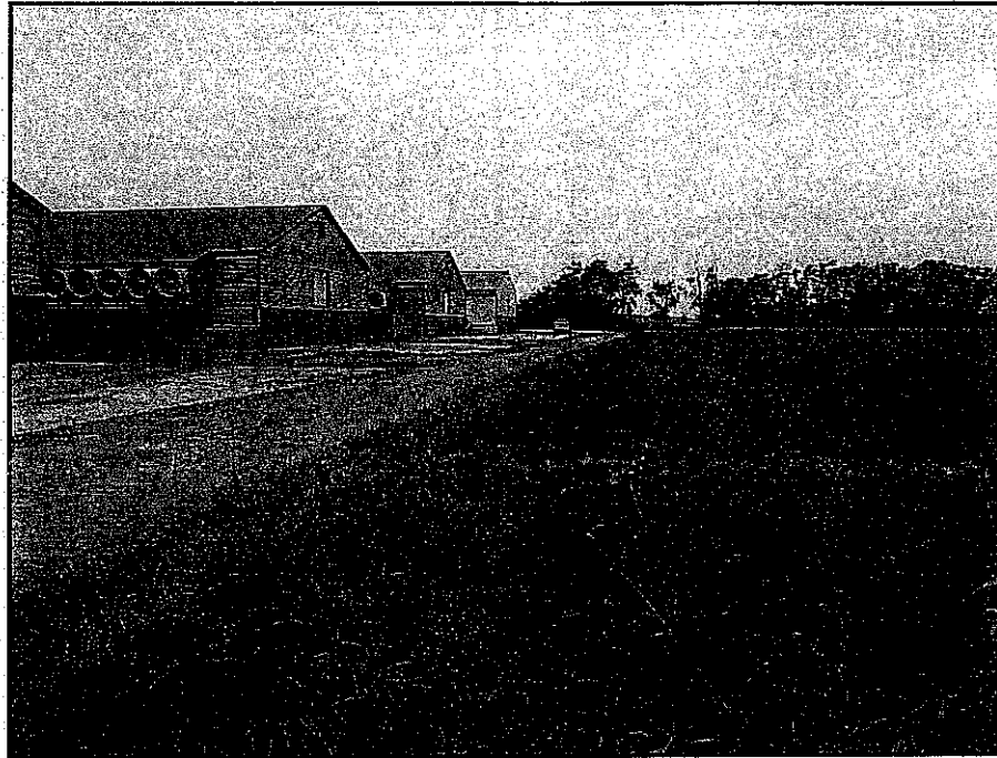
Stormwater runs away from buildings and directed into these vegetative swales.
