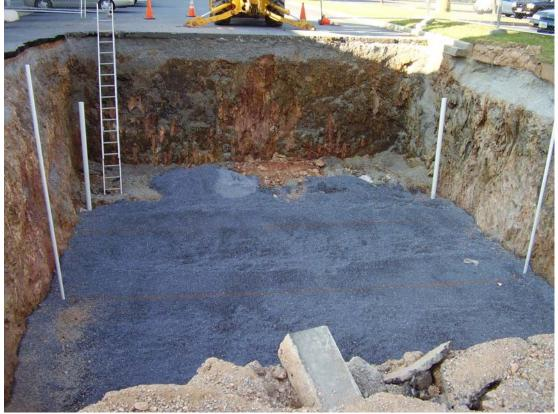
Photo 1- A view of the Green Valley Citgo tank field looking South towards former MW-3. Relict bedding planes are somewhat visible on the West (right) side wall (zoom in) between the two PVC pipes. Strike is generally less than N5<sup>o</sup>E and similar to geology observed under the canopy which is approximately 30 feet to the left of the photo.
