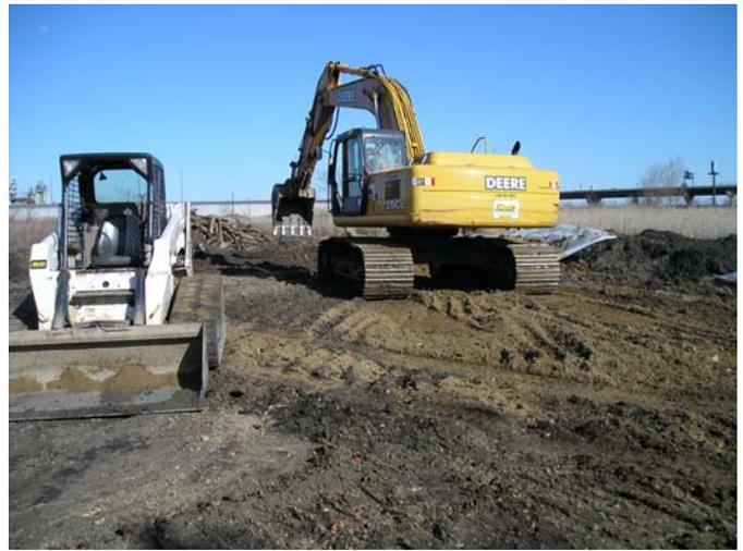
**PHOTOGRAPH 8** Compaction of Central Trench
