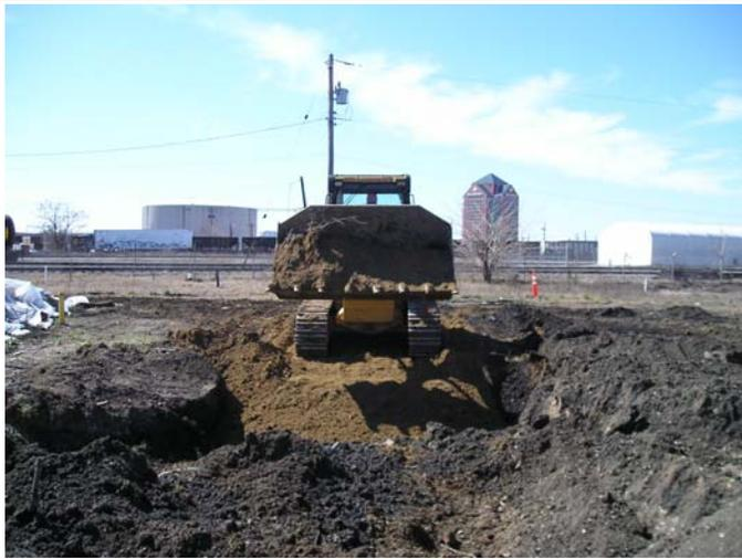
**PHOTOGRAPH 7** Backfill of Central Trench
