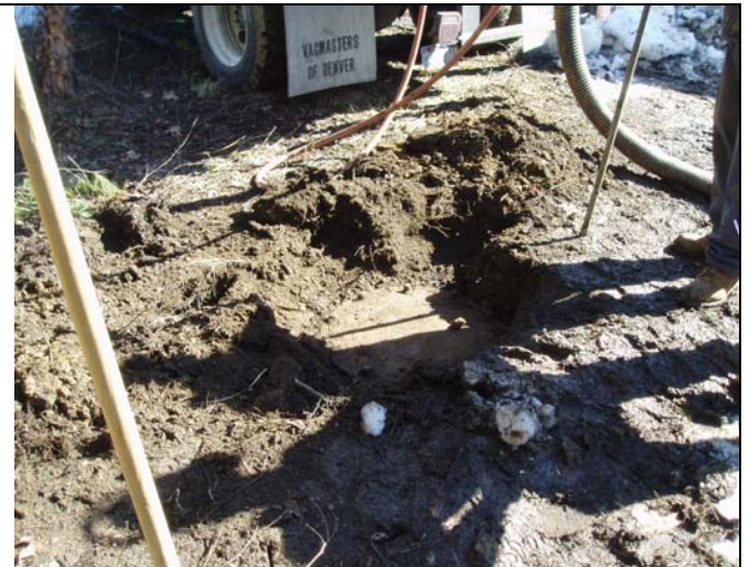
Photo 6: View of steel manhole exposed with air vacuum extraction at UST #2.
