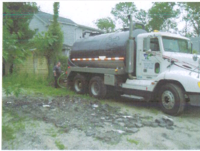
Photo 13: Setting up at UST # 4/5 to vacuum liquid contents.
