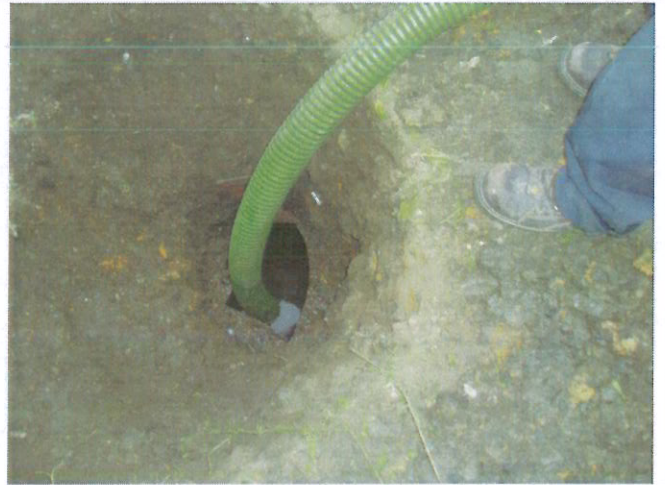
Photo 14: Draining water from UST # 4/5.
