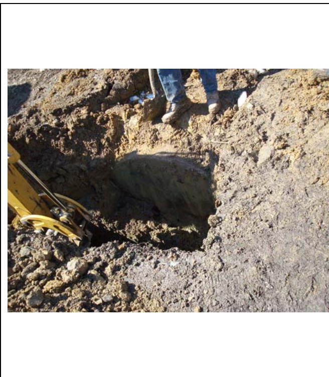
Photo 7: Test pit adjacent to exposed UST #1.
