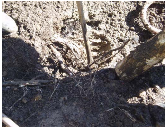
Photo 4: View of the air-knife and vacuum tube exposing tree roots within UST#2's access port.
