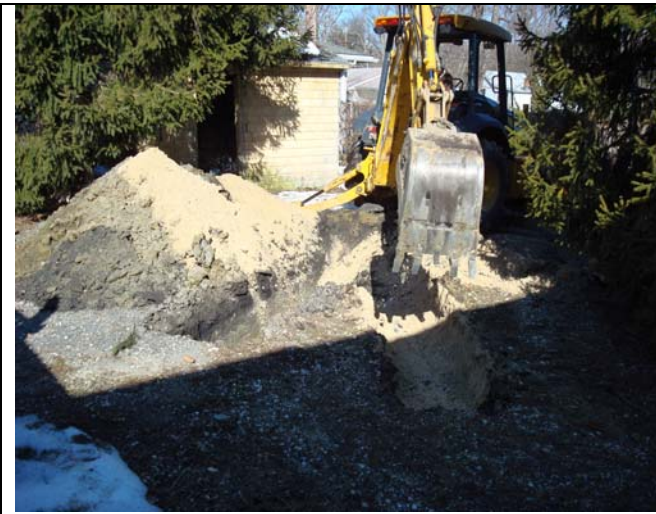
Photo 5: Excavation reveals clean sand backfill at UST target area #8.
