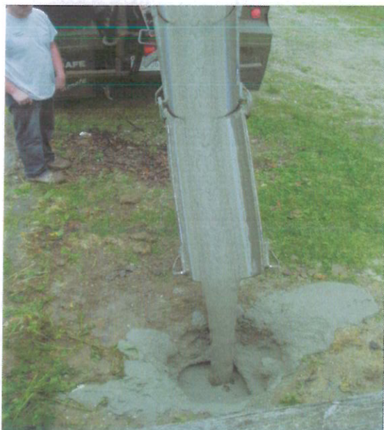
Photo 9: Sealing UST # 1 with flowable fill.
