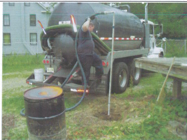
Photo 2: Preparation for draining product from UST #1.
