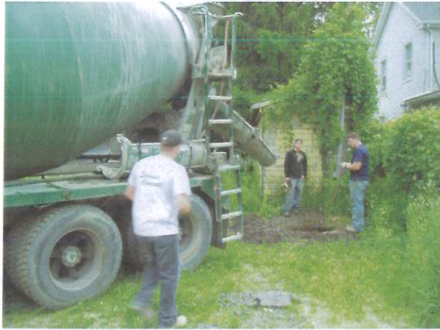
Photo 17: Setting up on UST #4/5 for sealing.
