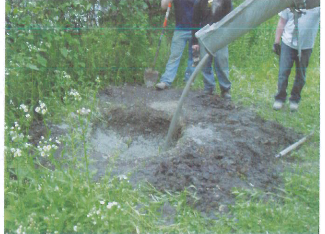
Photo 18: Sealing UST #4/5 with flowable fill.
