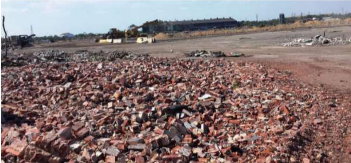
Materials Management Plan submitted and approved for reuse of concrete and brick. The plan requires sampling of each pile after crushing prior to reuse as backfill.
