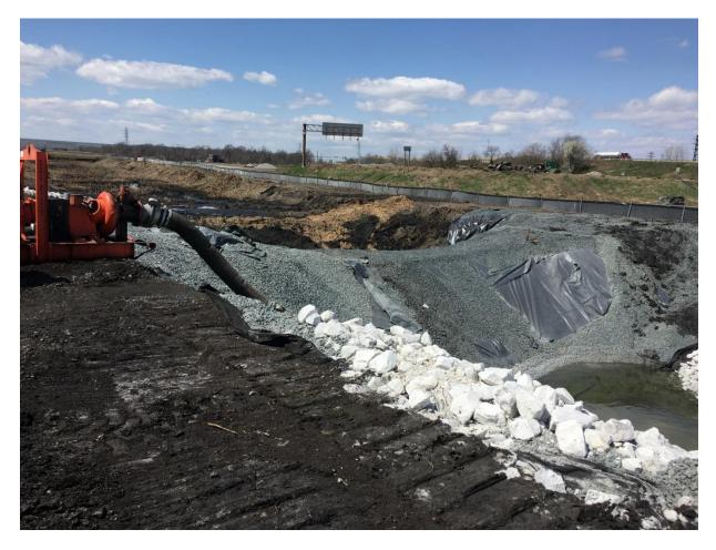
View of Coffer Dam at Upslope End of Active Work Section
