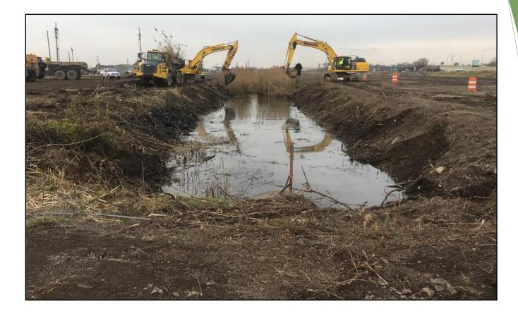
Removing Phragmites from Tin Mill Canal Prior to Sediment Removal
