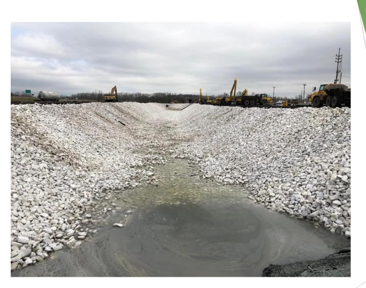
Sections #1 and #2 of Tin Mill Canal Following Placement of Rip- Rap
