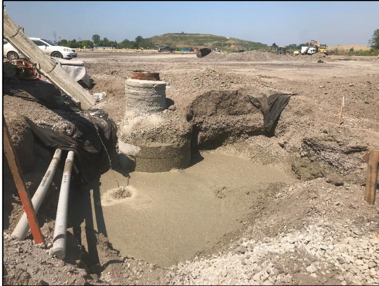
Photo 5: Trench plug construction
