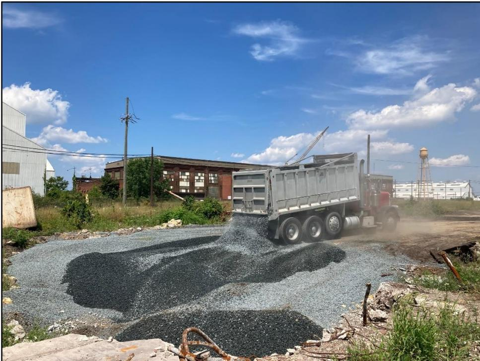
072720-1: End dump placing #57 stone during backfilling. A 38-ton wheel loader was used to spread and compact the stone.
