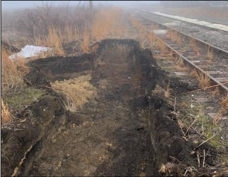
011720-1: B4-037Y excavation area was excavated to approximately 2 ft bgs. The excavation was located directly west of an active railroad line.
