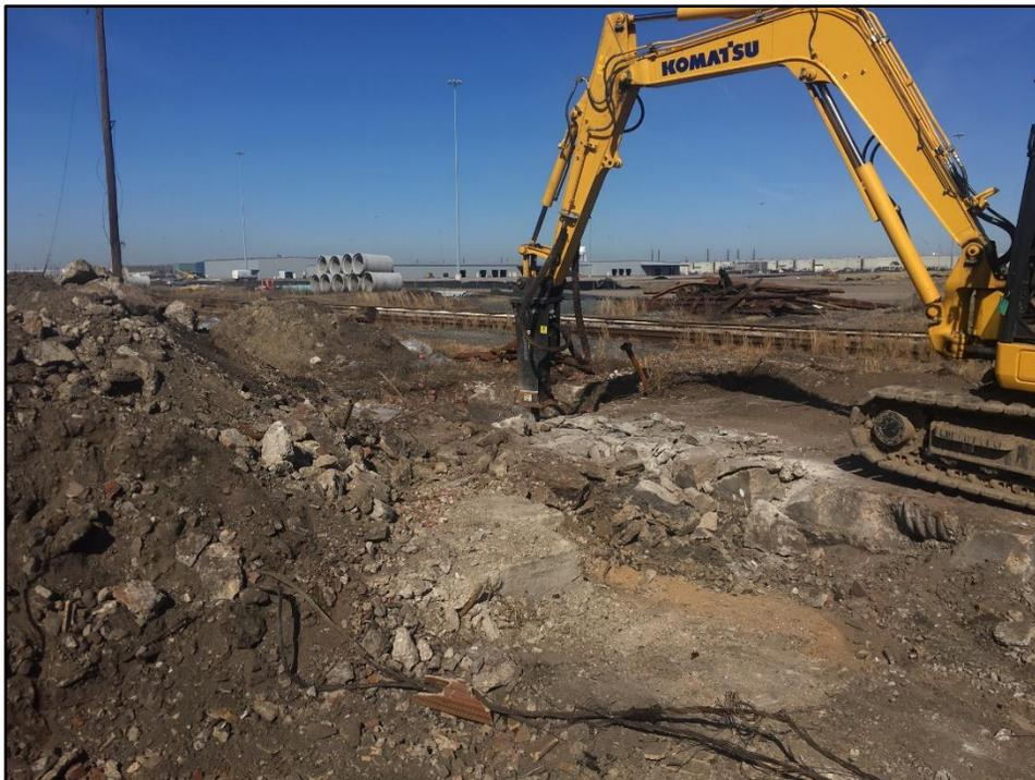
030920-2: Hydraulic hammer being used to remove the concrete area around the B4-037 excavation area.
