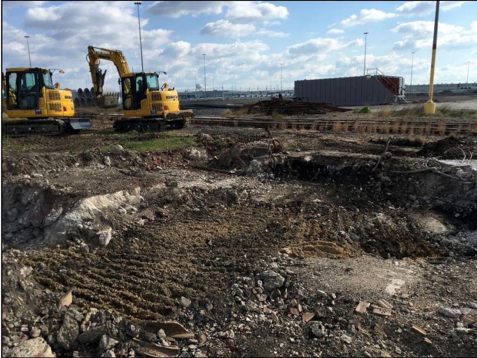
041620-1: The expanded excavation area, with a majority of the excavated area dug to approximately 3 ft bgs.
