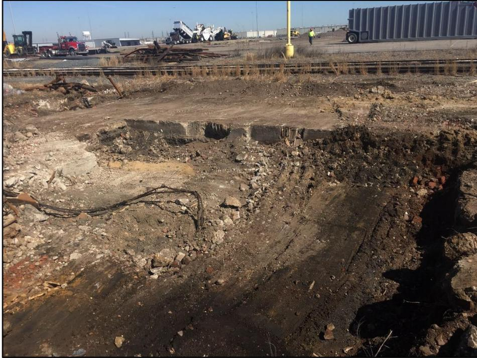
030920-1: Expanded B4-037B excavation area. Various layers of concrete were observed throughout the excavation.
