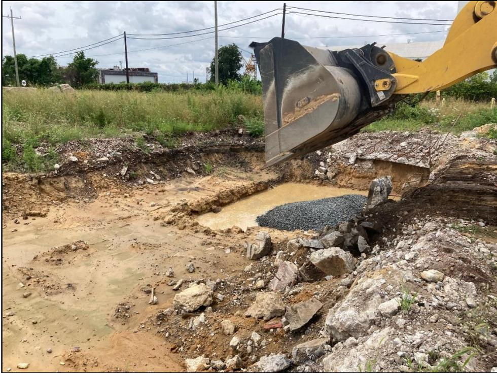
072420-1: Placing #57 stone fill in the deepest portion of the excavation.
