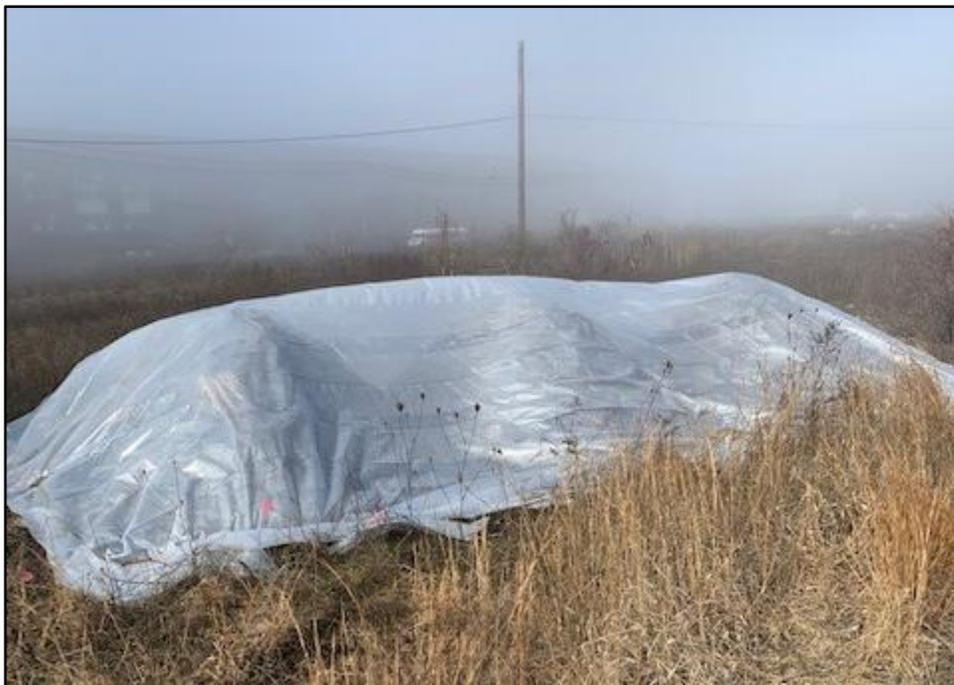
011720-4: Waste material stockpiled and covered after the first round of excavating.
