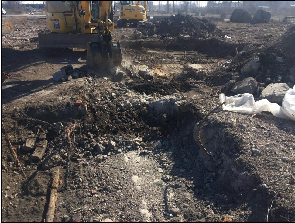
030920-3: Connecting the B4-037 and B4-037B excavation areas by removing soil and concrete located between the two areas.
