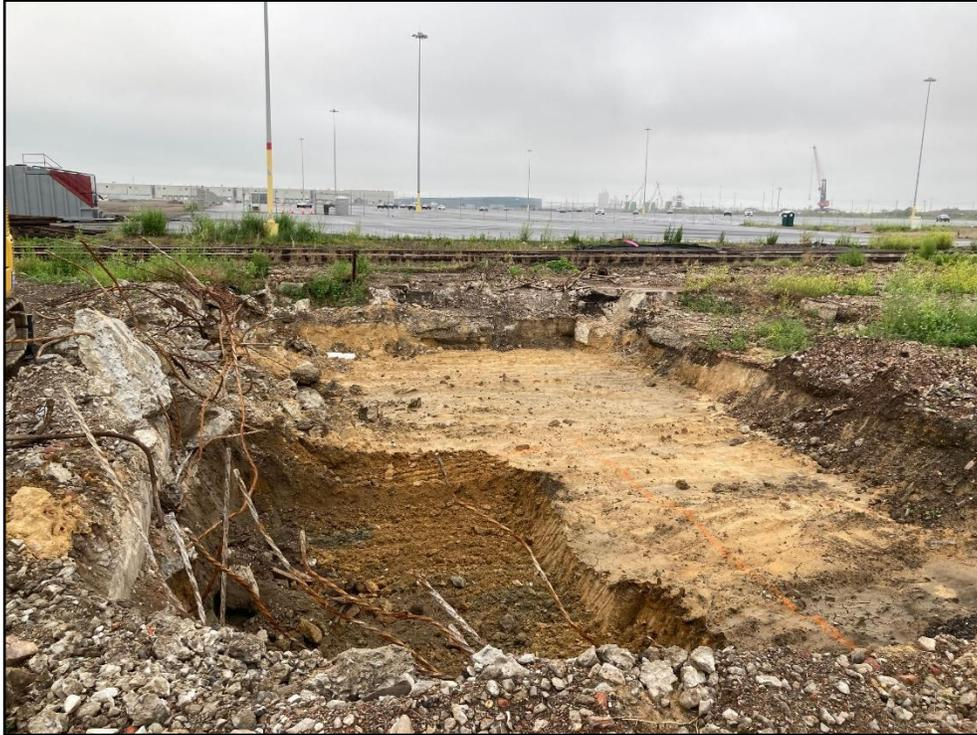
061820-1: Digging in the area of the final bottom sample exceedance. Soil below 4 feet bgs was lighter colored than the material above.
