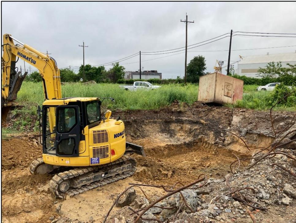
061820-2: Digging a portion of the excavation area to a depth of approximately 6 ft bgs. A majority of the excavation was dug to approximately 5 ft bgs, while the B4-037B area remained at approximately 1.5 ft bgs.
