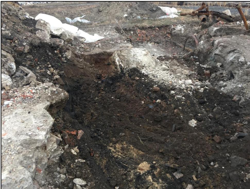
030920-4: Sub-surface material observed during the B4-037 and B4-037B excavation included concrete, slag, brick, and sand.
