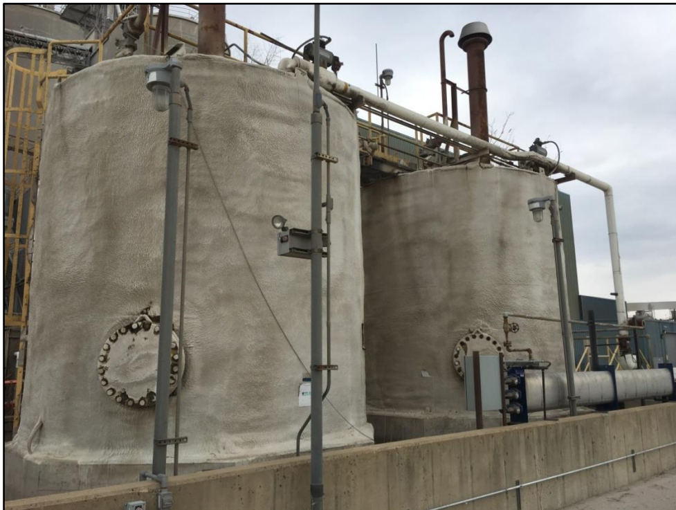
Photo 12 (3/15/18): View of two ASTs, one labeled as “used oil” and the other was unlabeled, located along the southwest corner of the Mill Building occupied by Lafarge.
