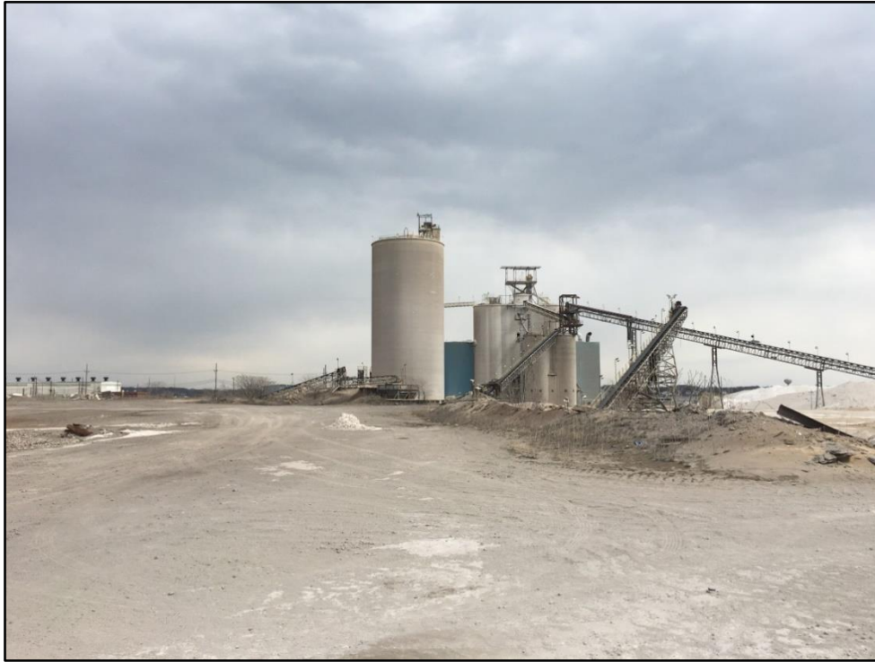
Photo 9 (3/15/18): Additional view of the Lafarge operations along the western perimeter of Parcel B20 facing east.
