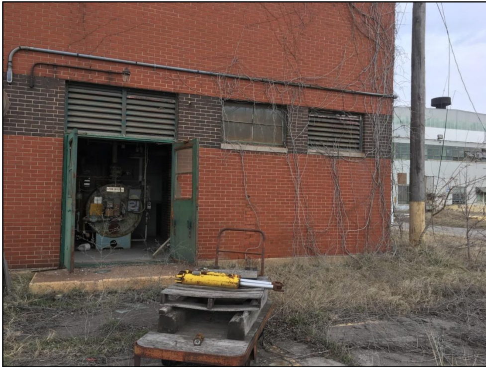
Photo 7 (3/15/18): Boiler room in southeast corner of service building.
