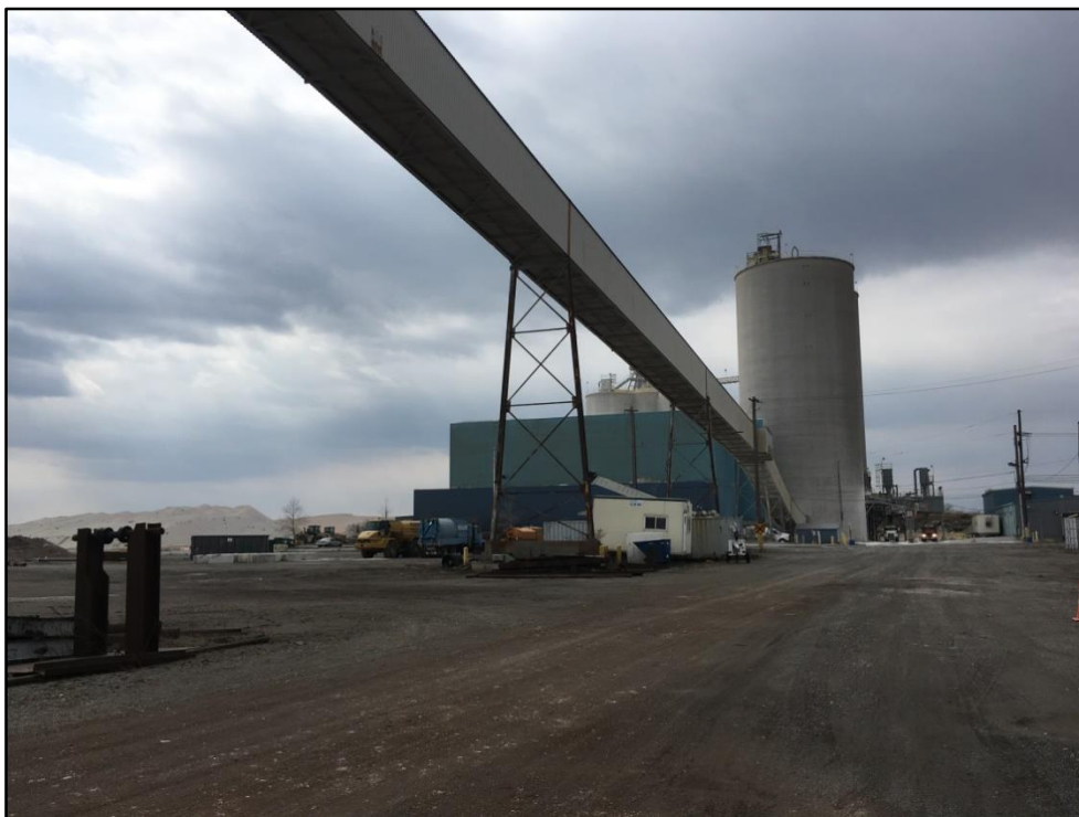
Photo 8 (3/15/18): View of the current Lafarge operations which includes storage silos, processing building, overhead conveyor, and material stockpiles.
