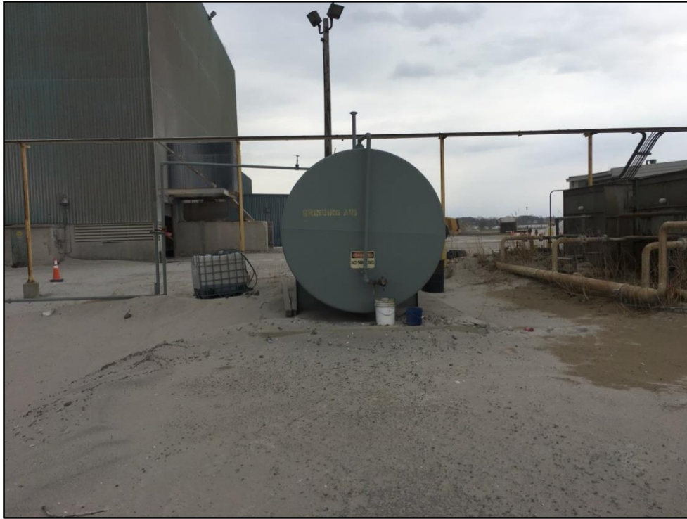
Photo 13 (3/15/18): View of a third AST labeled as “grinding aid” also located along the southwest corner of the Mill Building occupied by Lafarge.
