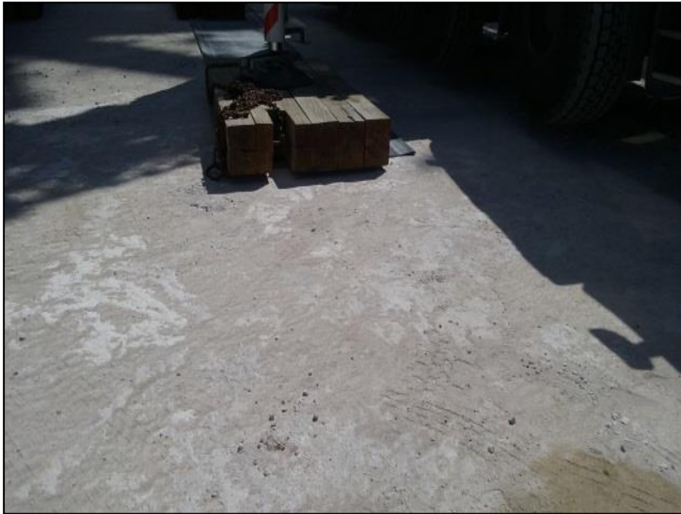
Photo 15 (8/26/16): Reported location of monitoring wells SW20-PZM006 and SW20-PZM041 next to the Mill Building. The wells could not be located.
