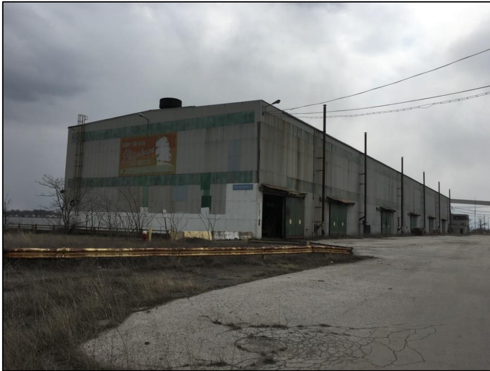
Photo 3 (3/15/18): View of Pennwood Wharf building located along the eastern shoreline facing south.
