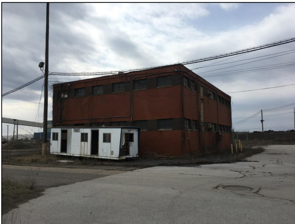
Photo 6 (3/15/18): View of former service building located southwest of the Pennwood Wharf building.
