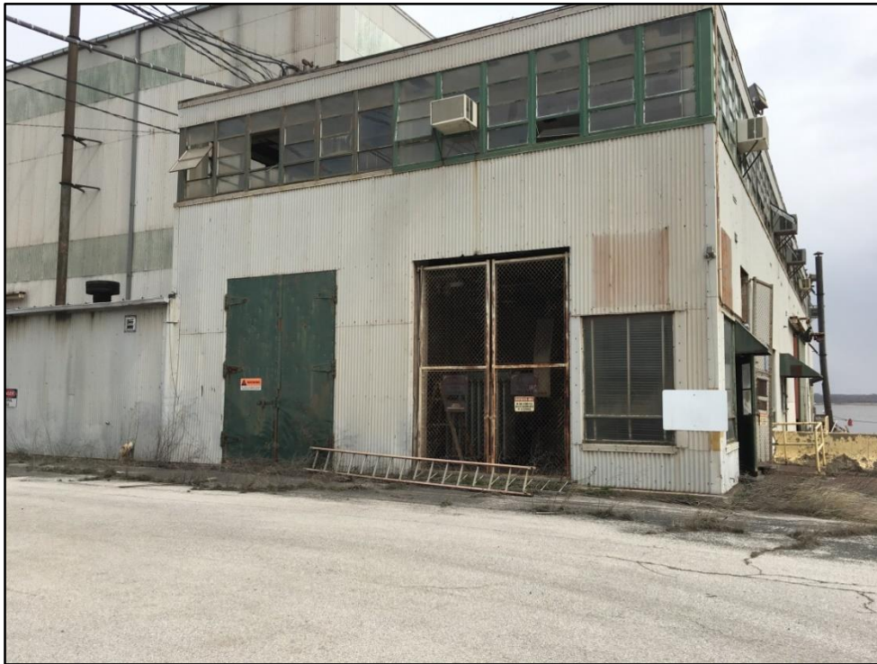
Photo 5 (3/15/18): View of an inactive substation located along the southwest corner of the Pennwood Wharf building.
