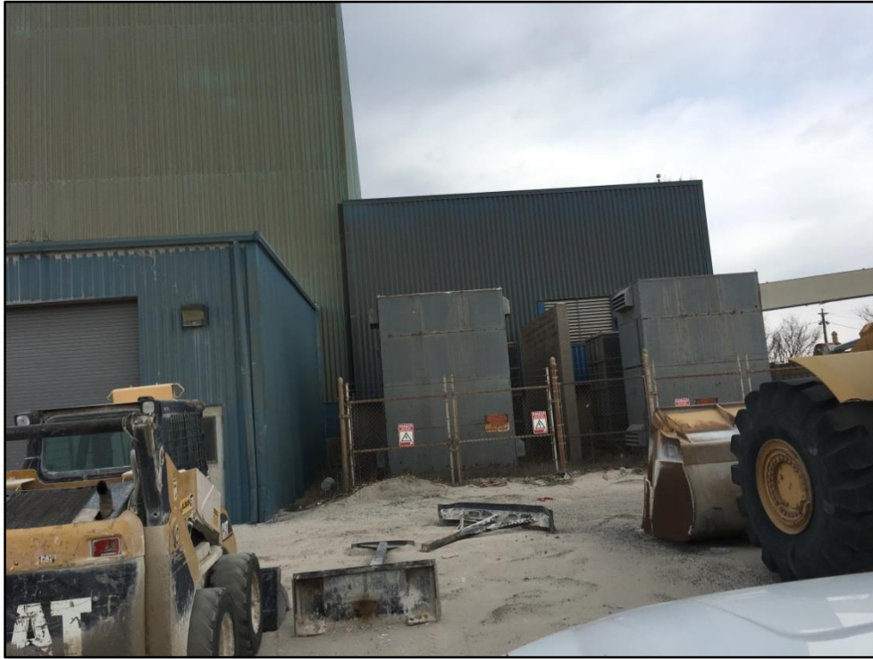
Photo 11 (3/15/18): View of another active substation, located along the southeast corner of the Mill Building, occupied by Lafarge.
