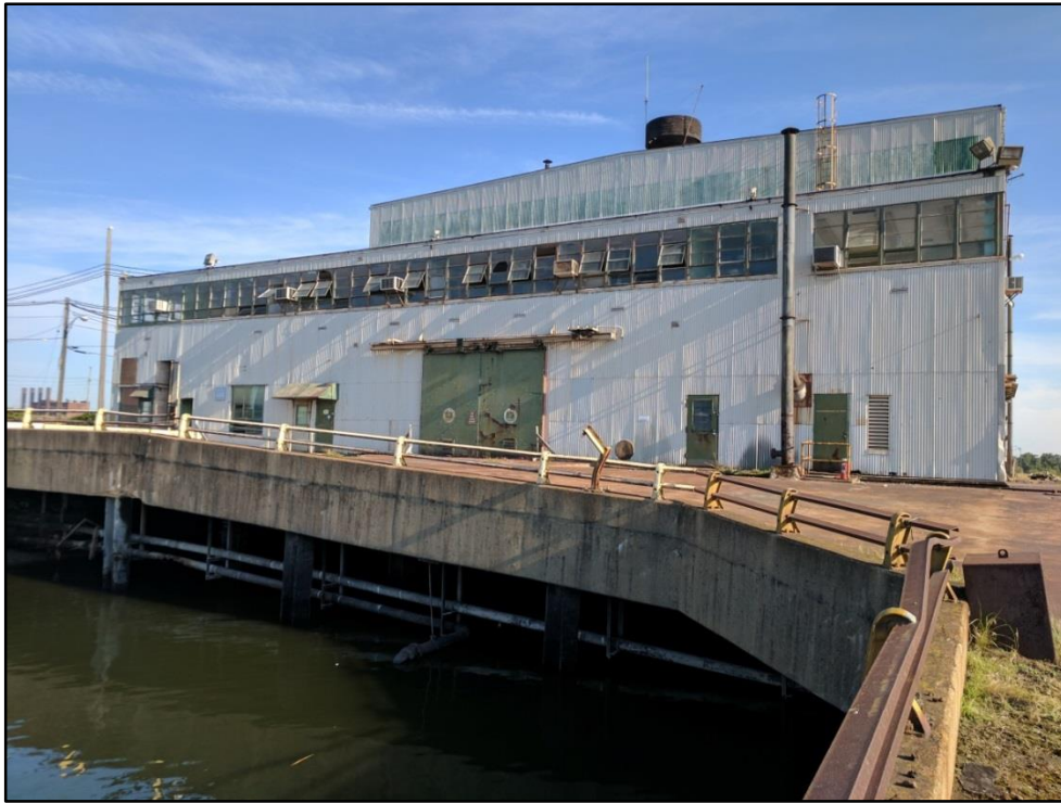
Photo 1 (7/31/17): Southern portion of the Pennwood Wharf building facing north.
