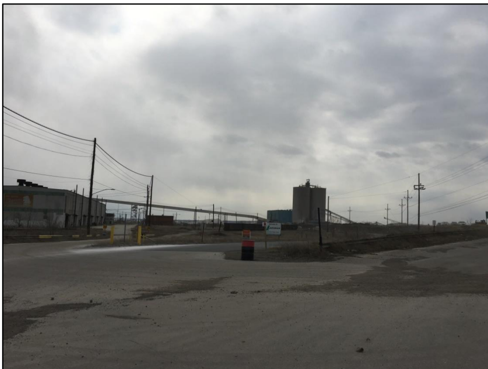
Photo 18 (3/15/18): General view of Parcel B20 facing south.
