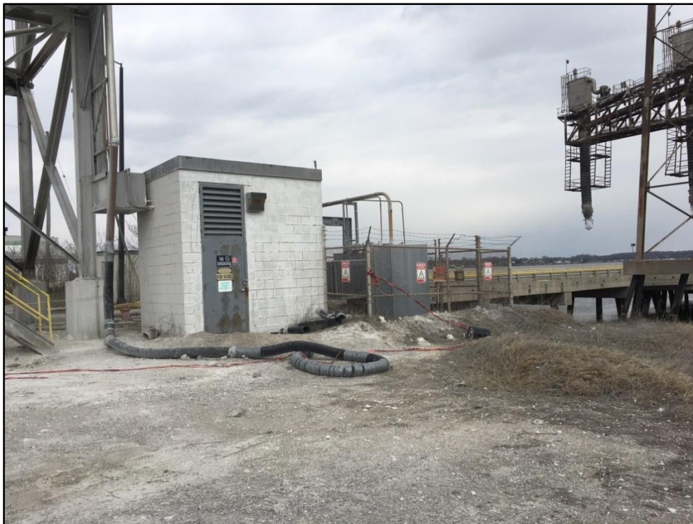
Photo 10 (3/15/18): View of an active substation, currently used by the Lafarge operations, located along the eastern shoreline.
