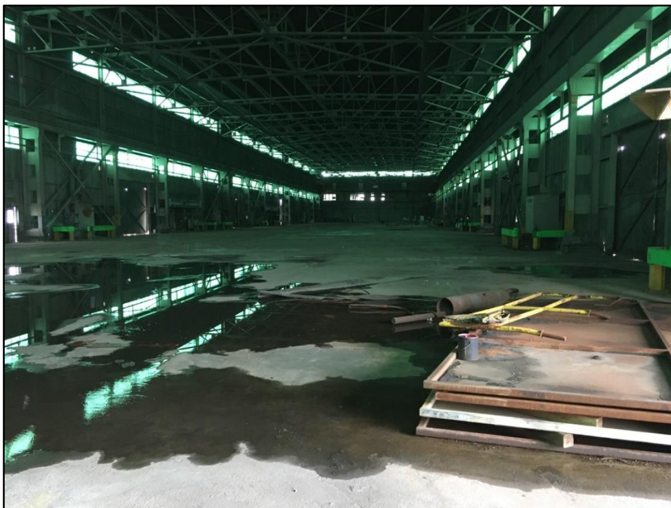
Photo 4 (3/15/18): Interior of empty Pennwood Wharf building.
