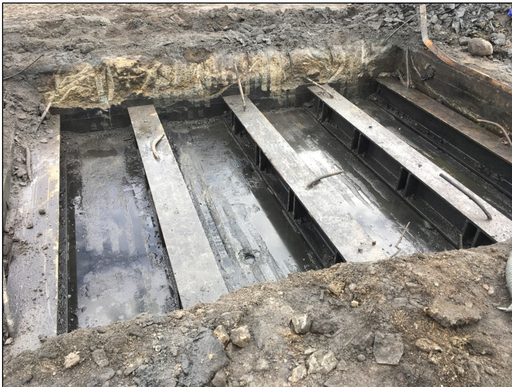
Photo 4: View of the cleaned concrete box facing east. Please note the circle along the concrete floor between the I-beams; this was the Geoprobe attempt to complete B17-007-SB.
