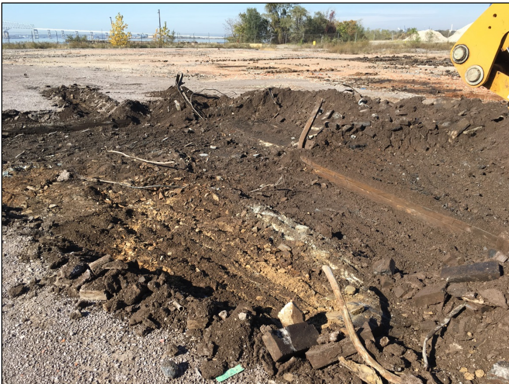
Photo 8: View of shallow test pit at B17-021-SB facing northwest. Reinforced concrete and large diameter rebar encountered during test pit activities. Little to no petroleum impacts observed.
