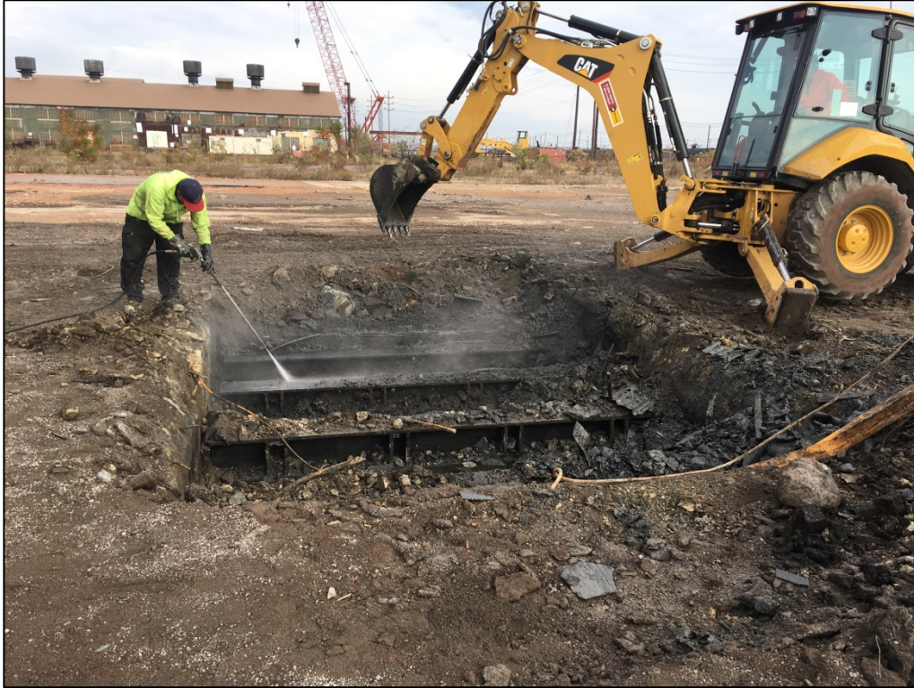
Photo 3: View of the ACE Environmental crew cleaning pit at B17-007-SB and the ENRC crew using the backhoe to remove the impacted material.
