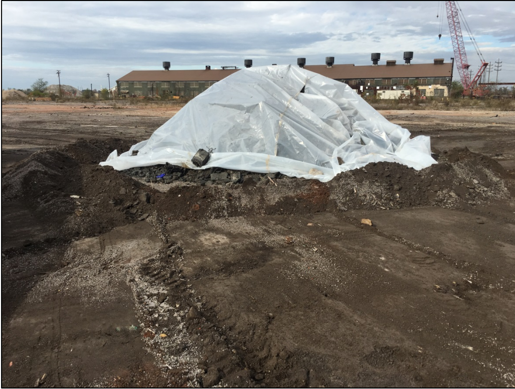
Photo 7: View of covered material removed from test pit at B17-007-SB facing north. A gravel filter berm was temporarily set up around the stockpile to prevent run-on and runoff of stormwater.
