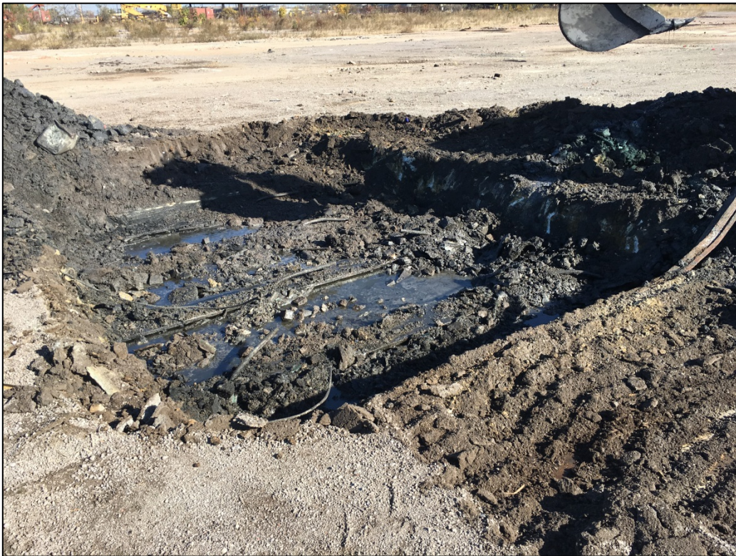
Photo 2: View of test pit at B17-007-SB prior to clearing and cleaning.
