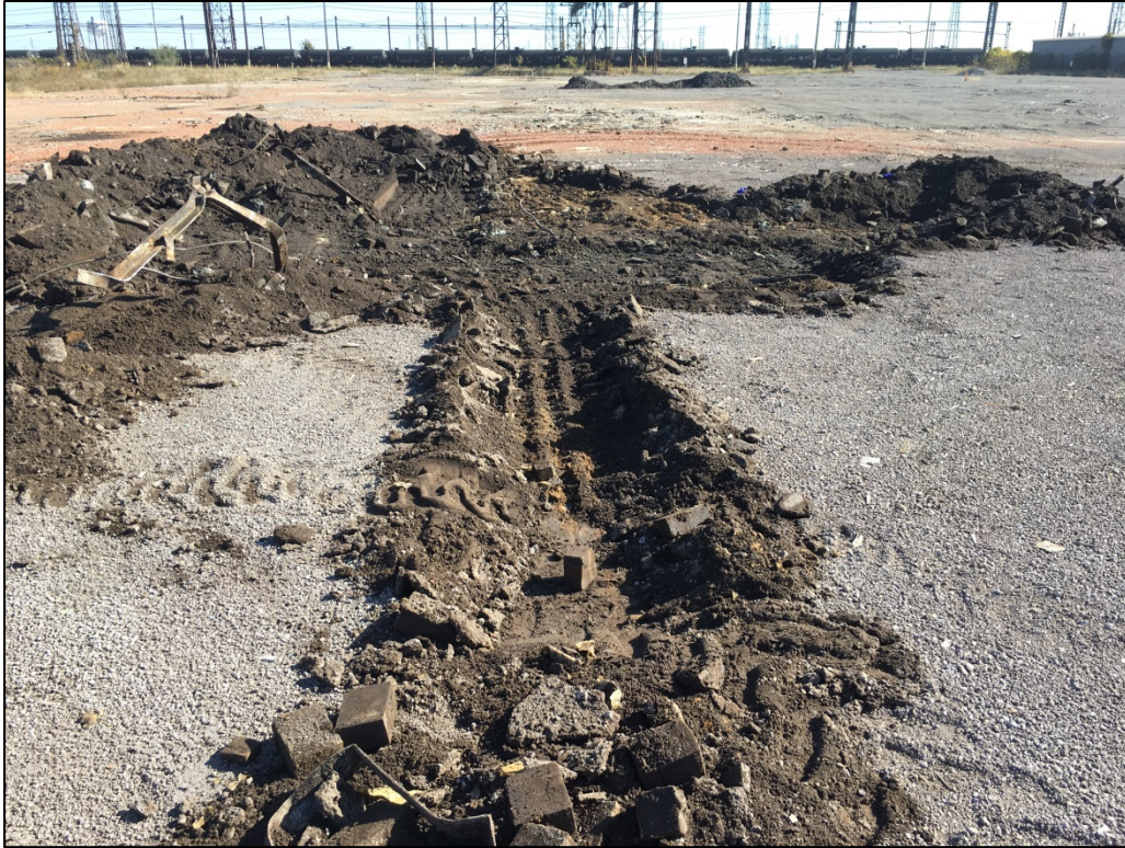
Photo 9: View of shallow test pit at B17-021-SB facing east. Reinforced concrete and large diameter rebar encountered during test pit activities. Little to no petroleum impacts observed.
