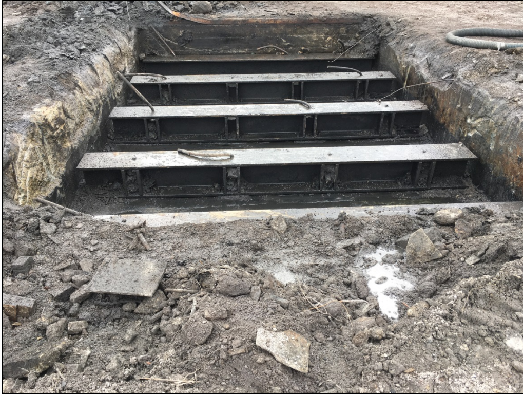
Photo 5: View of the cleaned concrete box facing south.
