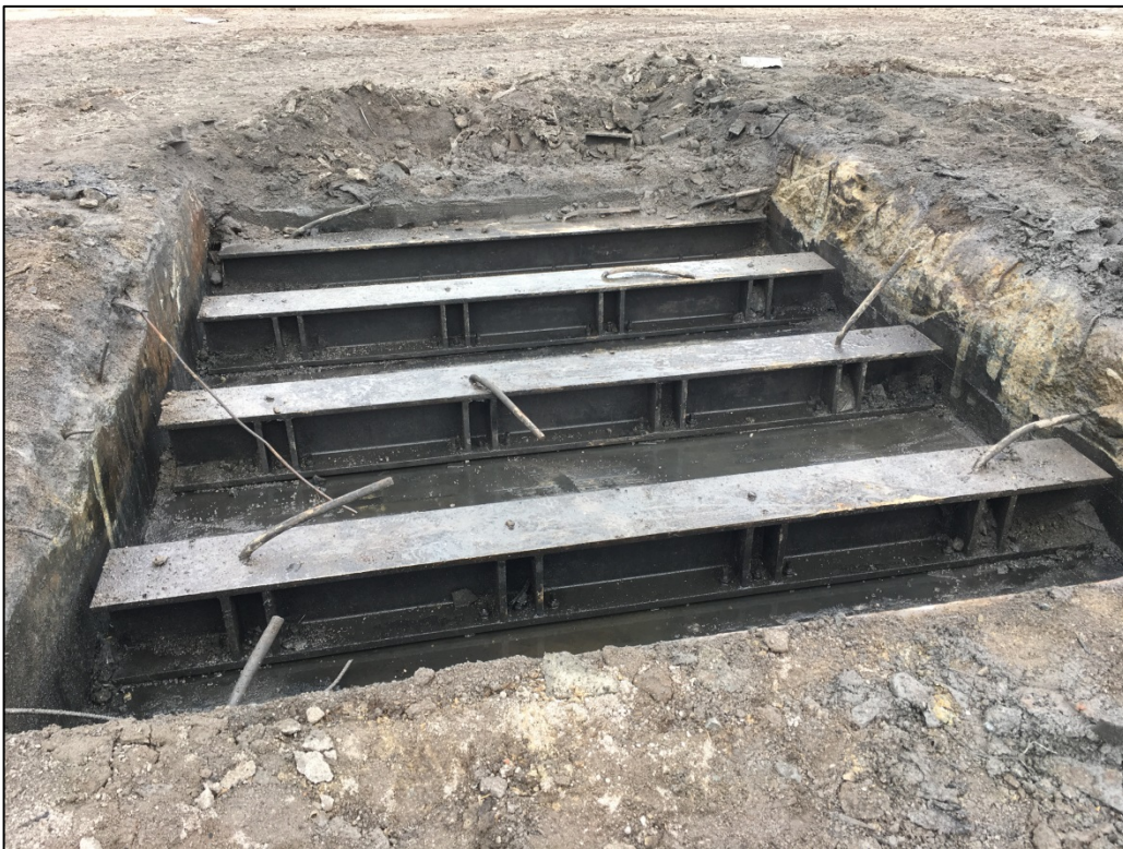
Photo 6: View of the cleaned concrete box facing north.
