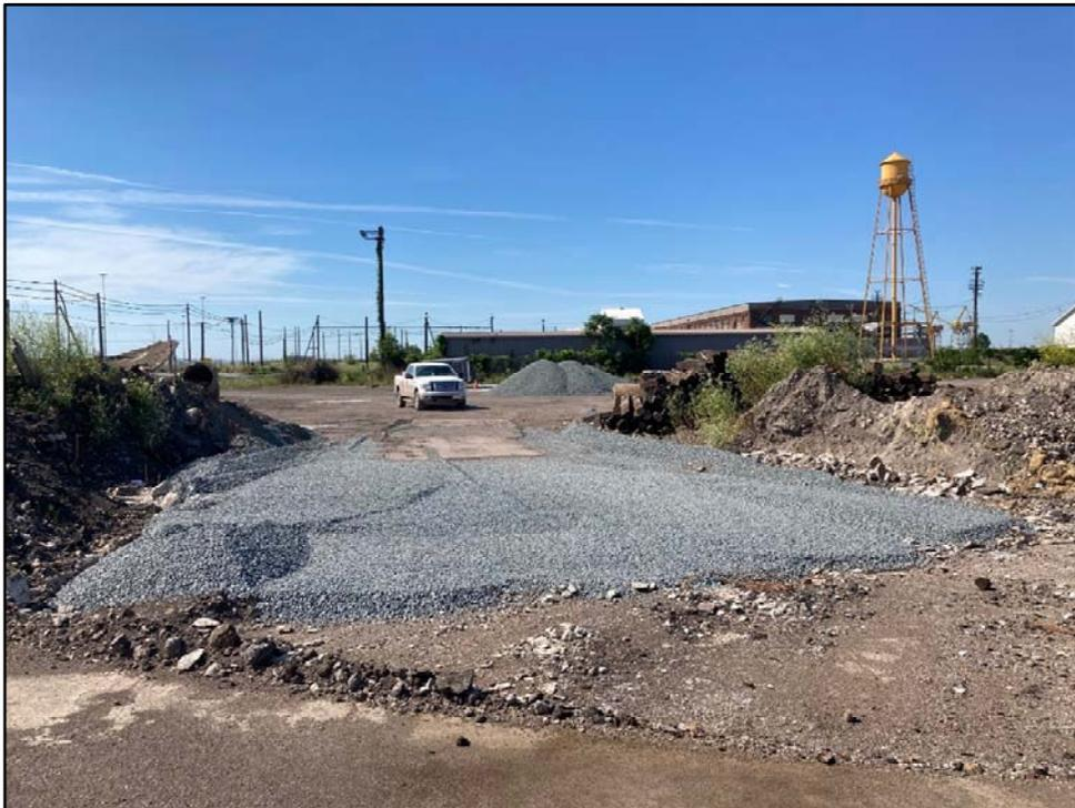
062620-2: Backfilling of B17-019-SB excavation area.
