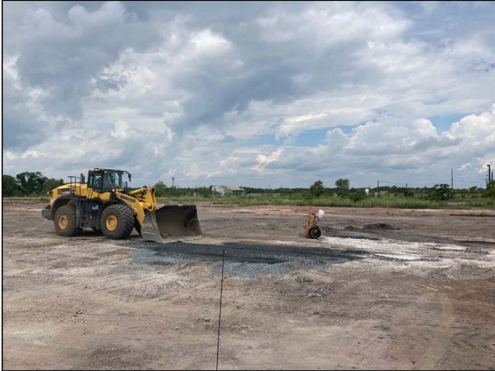
061920-3: Backfilling of B17-008-SB excavation area.
