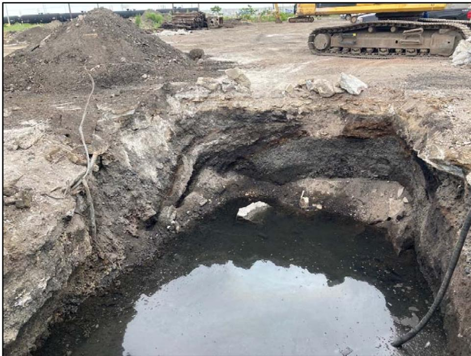
060220-1: B17-008-SB excavation area during groundwater removal with a vacuum truck. Groundwater was observed to be tide-dependent. Approximately 7,000 gallons of groundwater was removed from the excavation to bring the water level down to approximately 20" above the bottom of the excavation.
