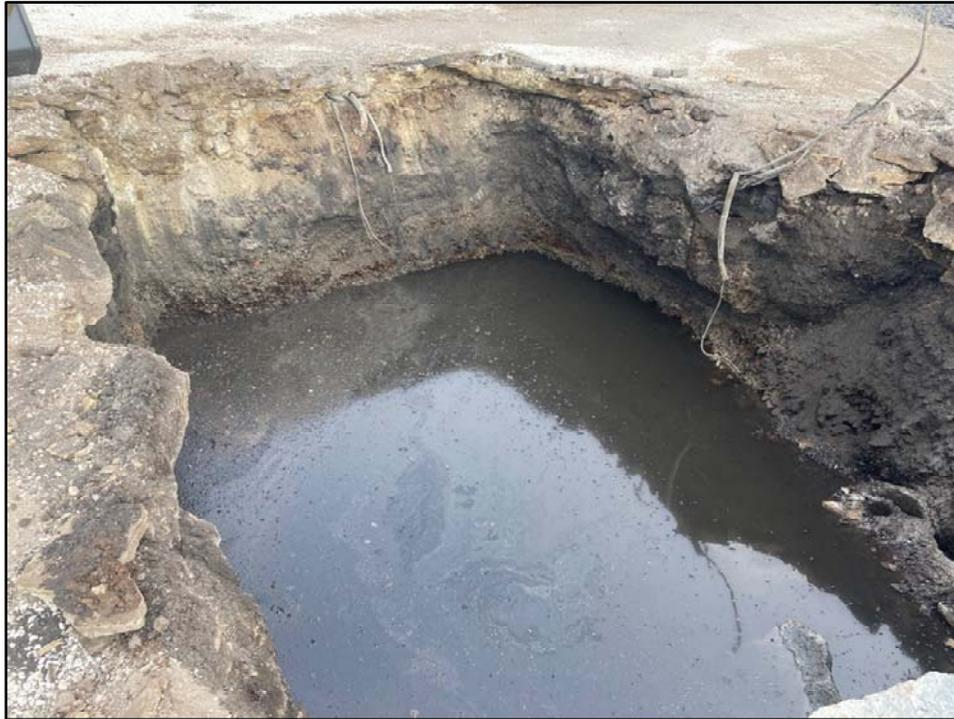
052920-1: B17-008-SB excavation area was excavated to approximately 8 ft bgs. Groundwater observed with a depth of 2-3 ft from the bottom of the excavated area.
