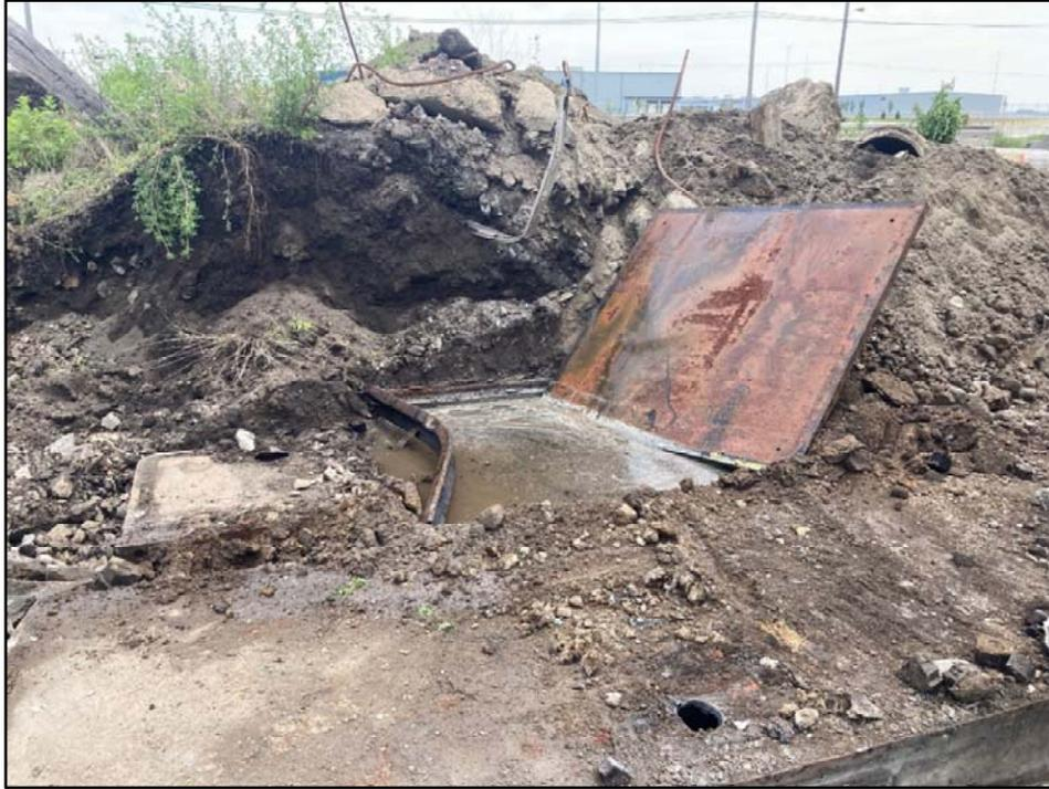
052920-4: A vault uncovered in the southeast corner of the B17-019-SB excavation area. Water in the vault was removed with a vacuum truck.
