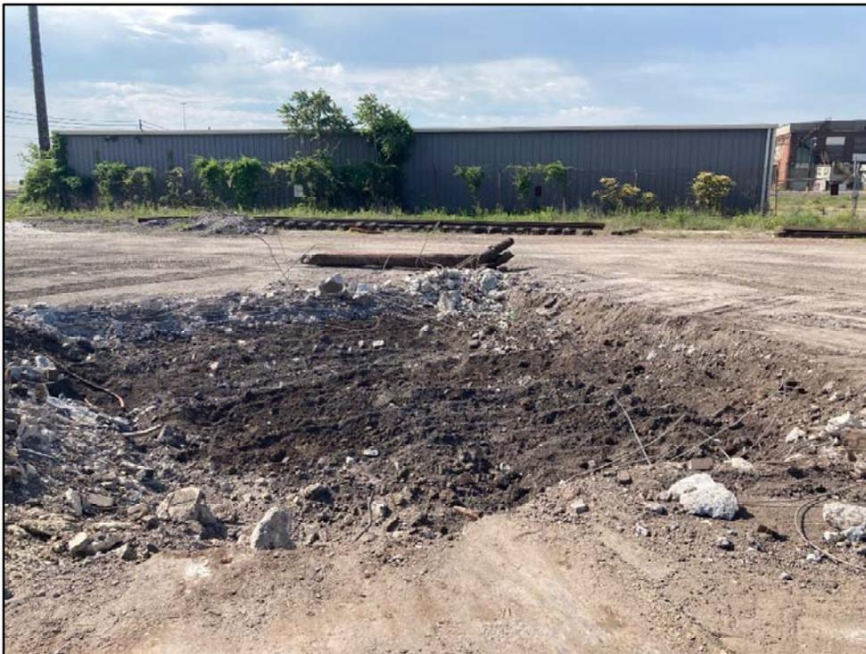
060220-3: B17-014A-SB excavation area was excavated to approximately 2 ft bgs. Rebar from the removed concrete foundations was observed around the excavation.
