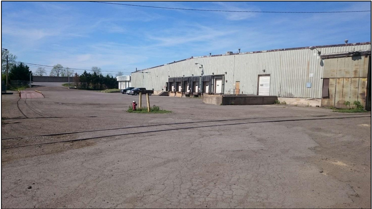
Photo 19 (4/24/19): Wide-angle view of the southwestern portion of the Site, facing north. The western site entrance is visible in the background.
