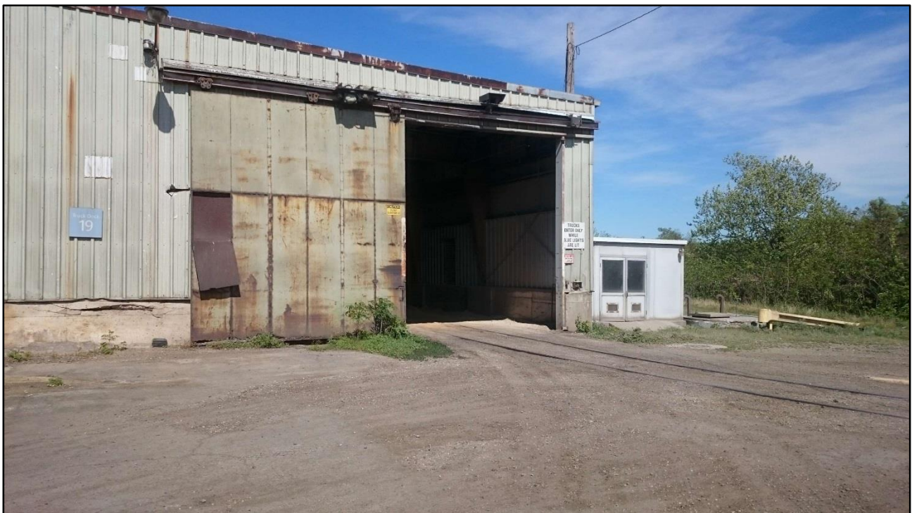
Photo 8 (4/24/19): Active railway into large bay at the southern corner of the CRW, facing northeast.
