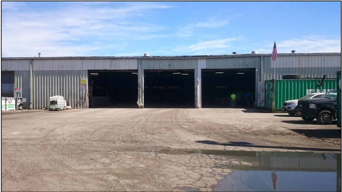
Photo 23 (4/24/19): View of bay doors on the northwestern side of the CRW, facing southeast. Miscellaneous storage on either side of the bay doors.
