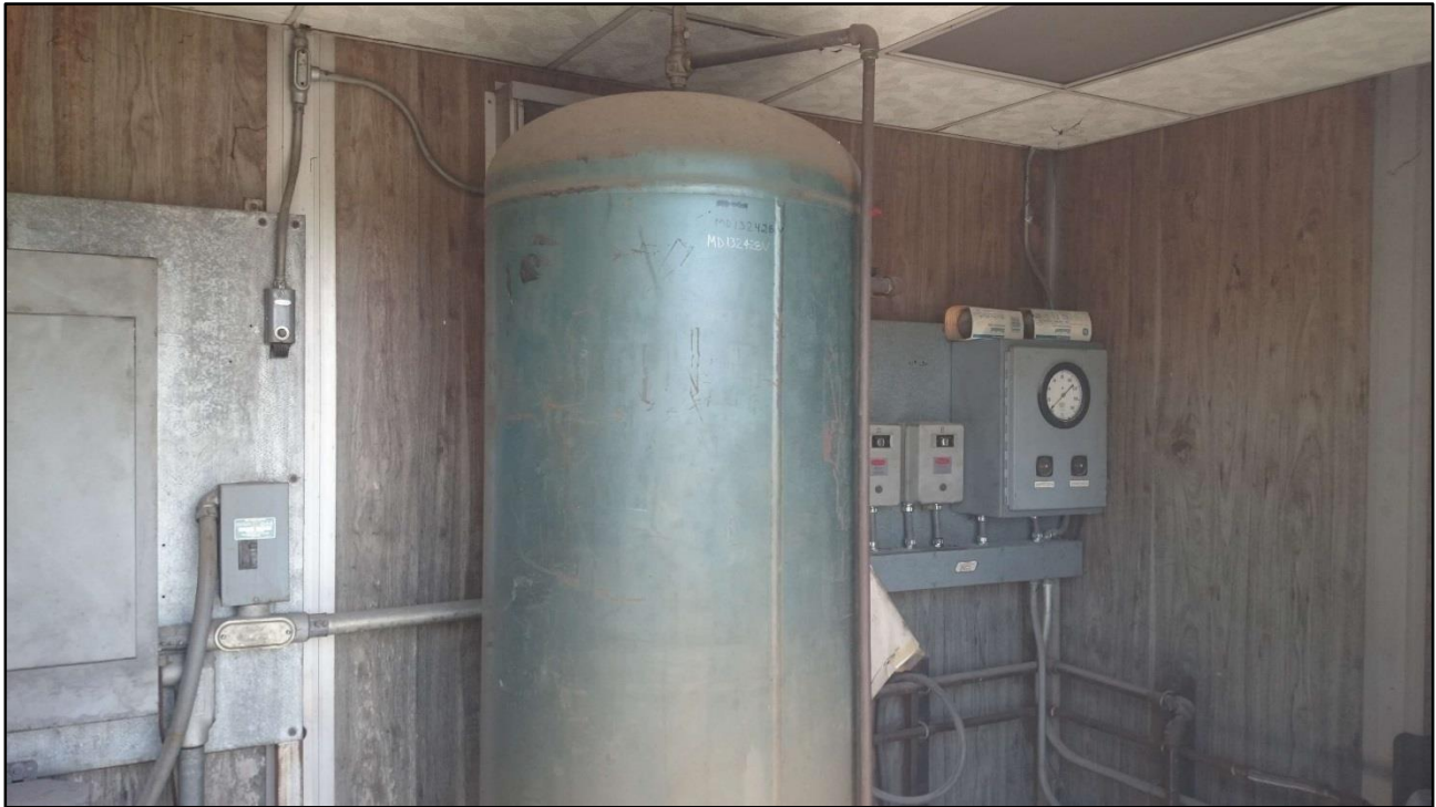
Photo 11 (4/24/19): Tank (possibly for compressed air) in the center of the outbuilding.
