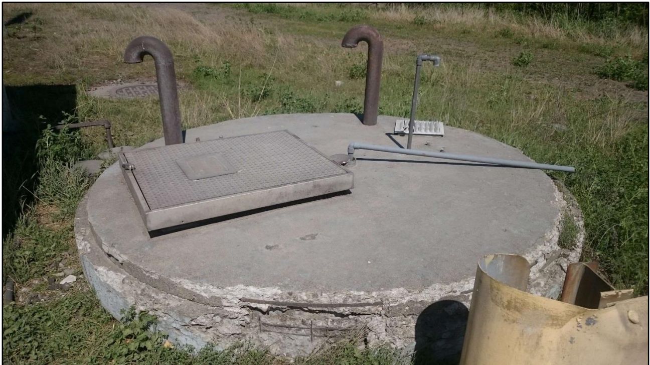
Photo 14 (4/24/19): Exterior view of the wet well adjacent to the outbuilding. Hatch is marked with warnings as a confined space.
