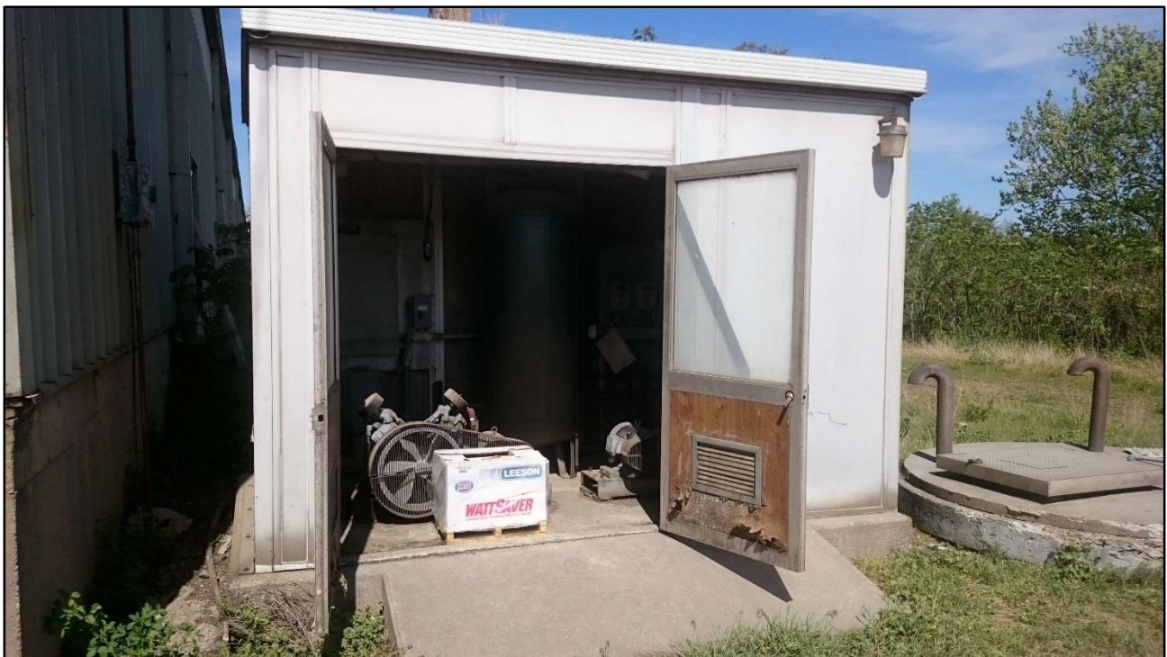
Photo 10 (4/24/19): Interior view of the outbuilding, with features of potential interest (see trailing photographs).
