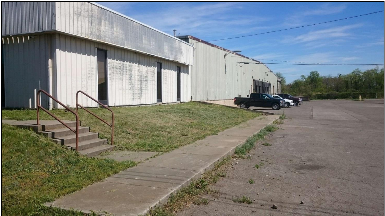
Photo 2 (4/24/19): View of the Central Receiving Warehouse (CRW), facing east.
