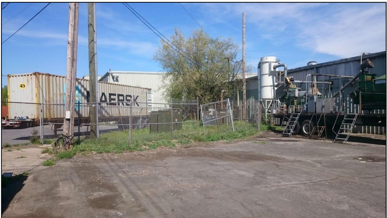
Photo 24 (4/24/19): View of electrical equipment at the far northern corner of the Site. Access to this area is restricted by chain-link fence.
