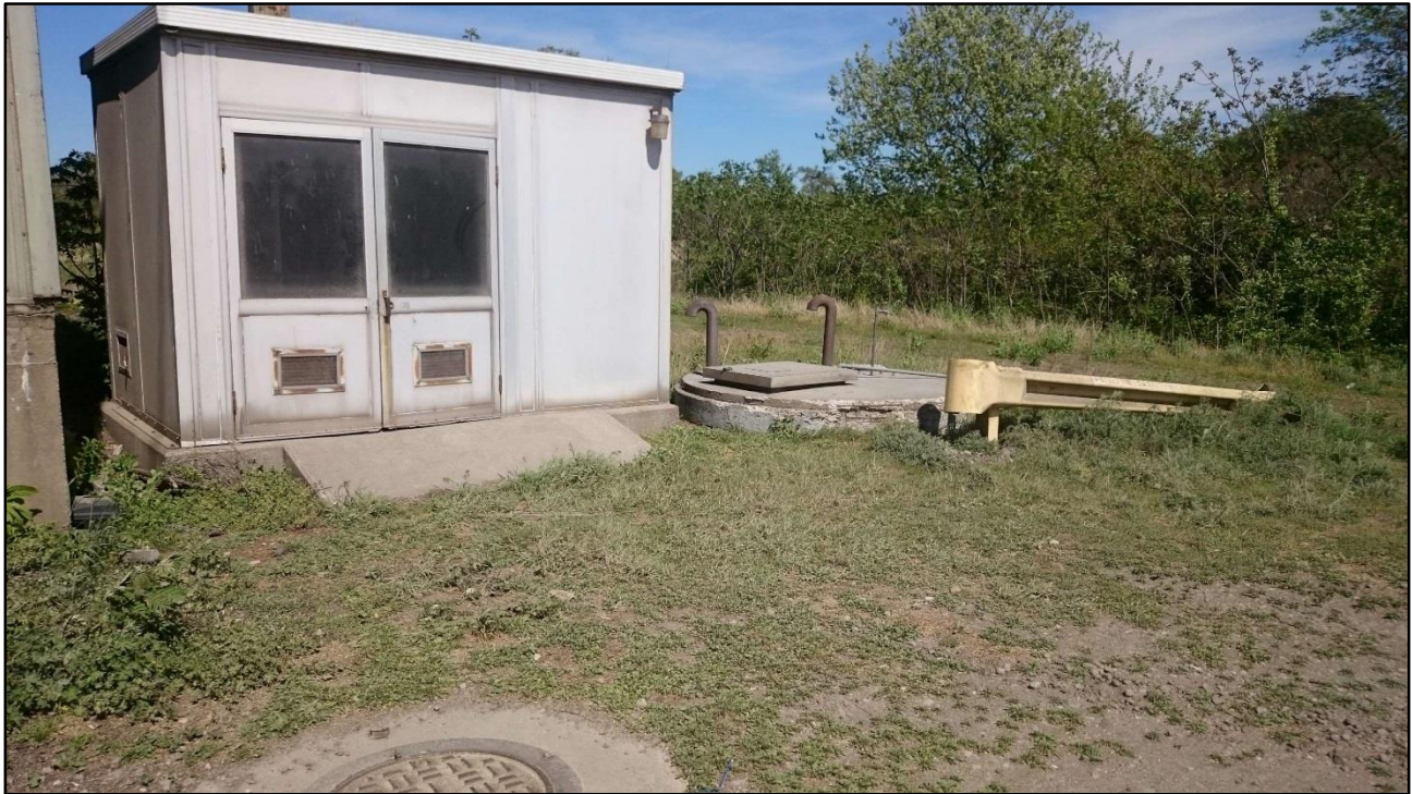
Photo 9 (4/24/19): Small outbuilding (ejector station) at the southern corner of the CRW, facing northeast. Buried wet well is present immediately to the southeast of the outbuilding.
