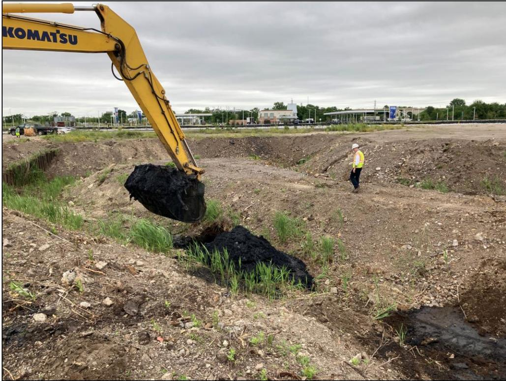
061720-3: View of excavated material from test pitting activities at the PORI Lagoon. Sheet piling is visible in the background.
