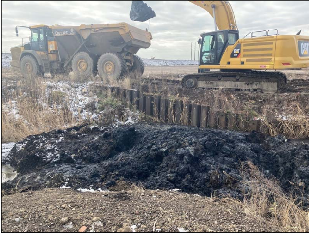
121820-3: Material placed within the lagoon for drying. Historic sheet piling observed in some sections of the PORI Lagoon's sidewalls was left in place.
