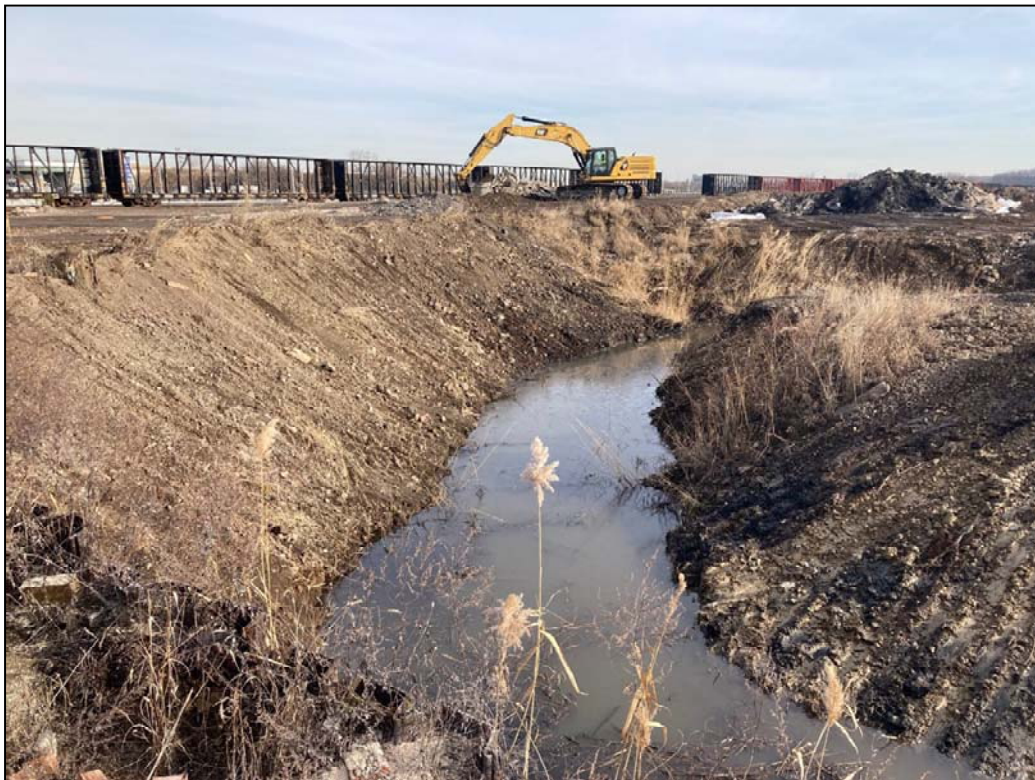
122320-2: The northern portion of the PORI Lagoon near the completion of material removal.
