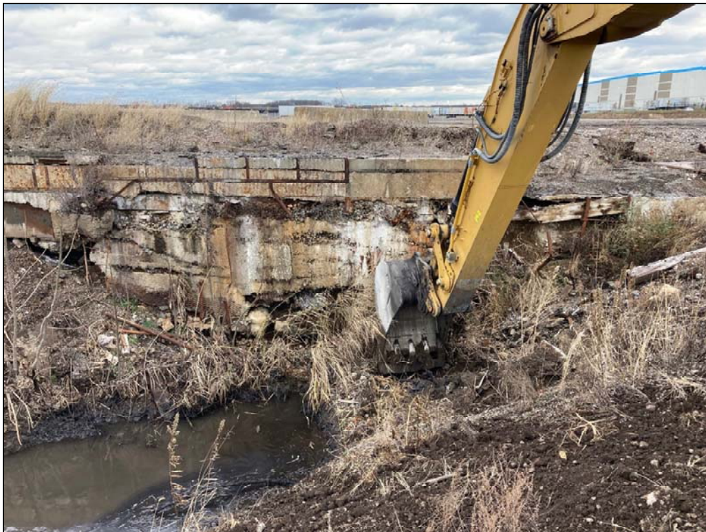
122220-1: Material excavation in the southeastern end of the lagoon.
