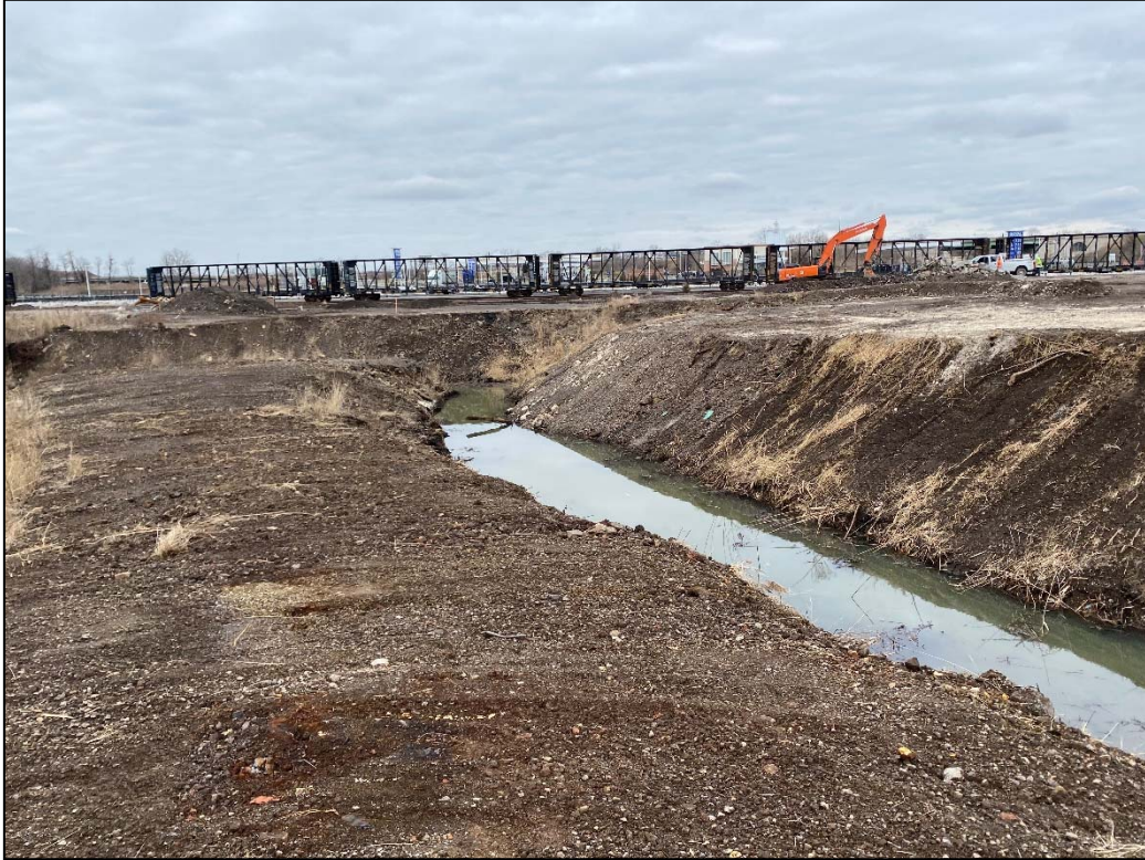
010521-1: The eastern portion of the PORI Lagoon following the completion of material removal.
