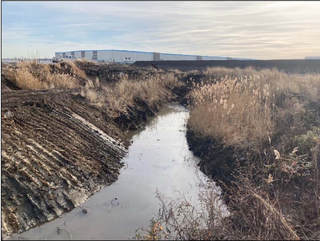
122320-1: The western portion of the PORI Lagoon near the completion of material removal.
