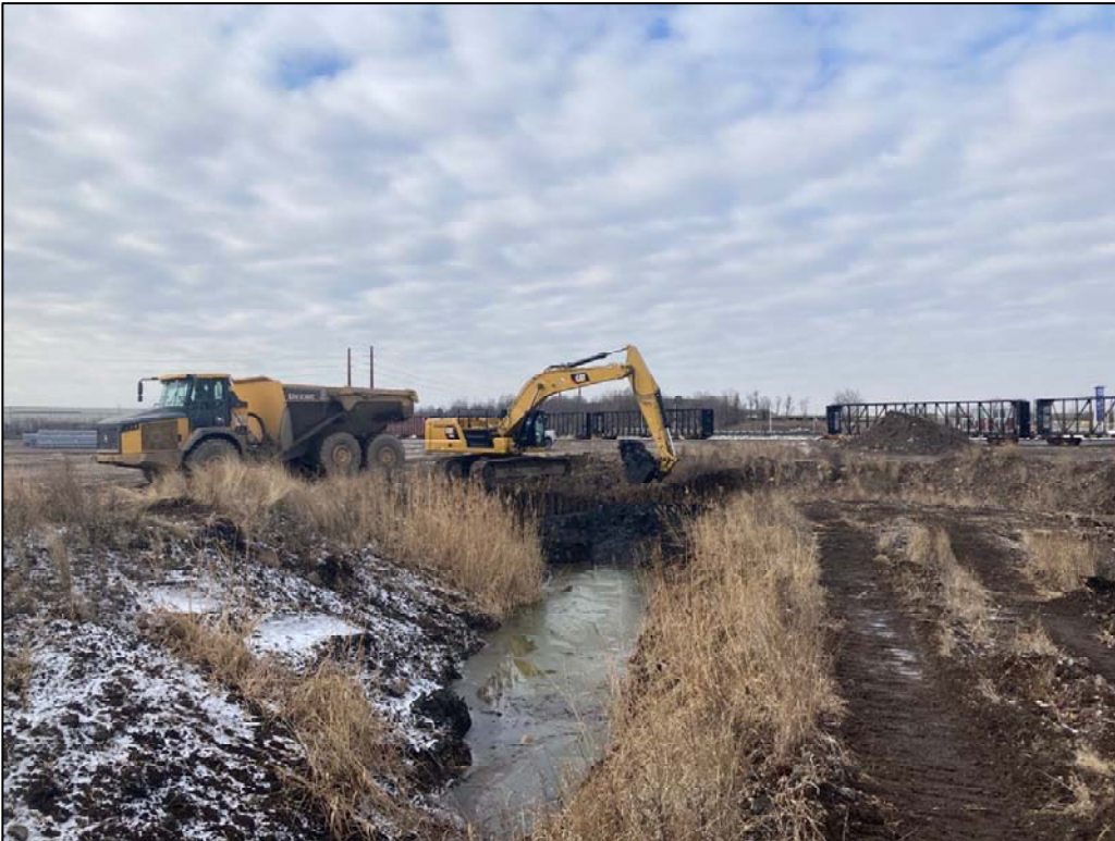
121820-2: Dried material being loaded for transport to Greys Landfill.
