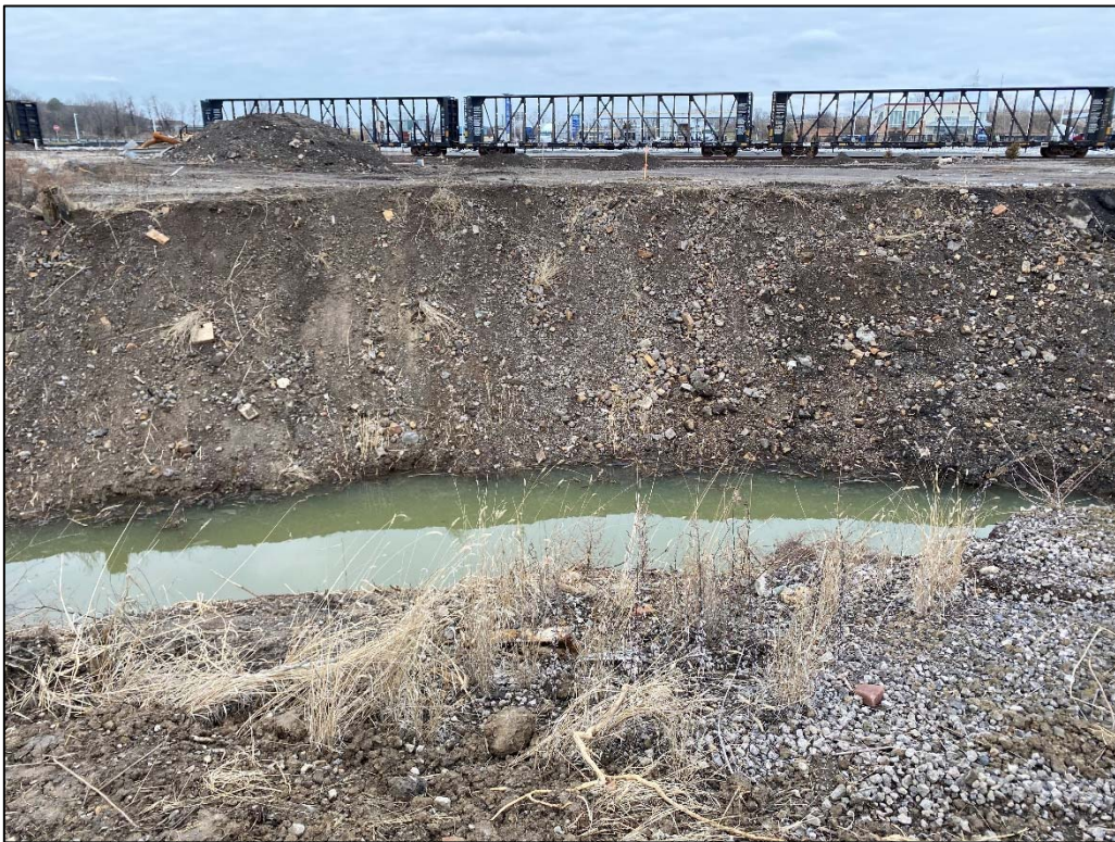
010521-2: The northern portion of the PORI Lagoon following the completion of material removal.
