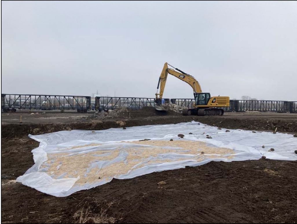
122120-2: Material dry-out pad constructed with polyethylene sheeting and a berm. The dry-out pad allowed liquids drained out of the excavated material to drain into the lagoon.
