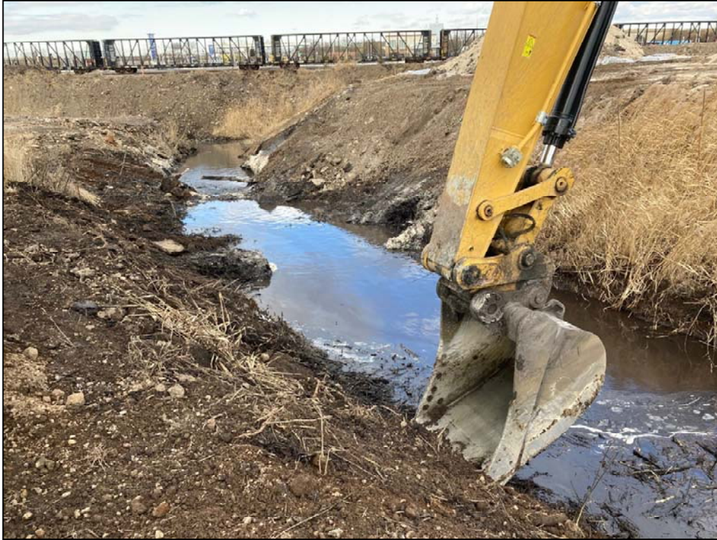
122220-2: Excavator bucket completing confirmation sampling at the approximate water table elevation.
