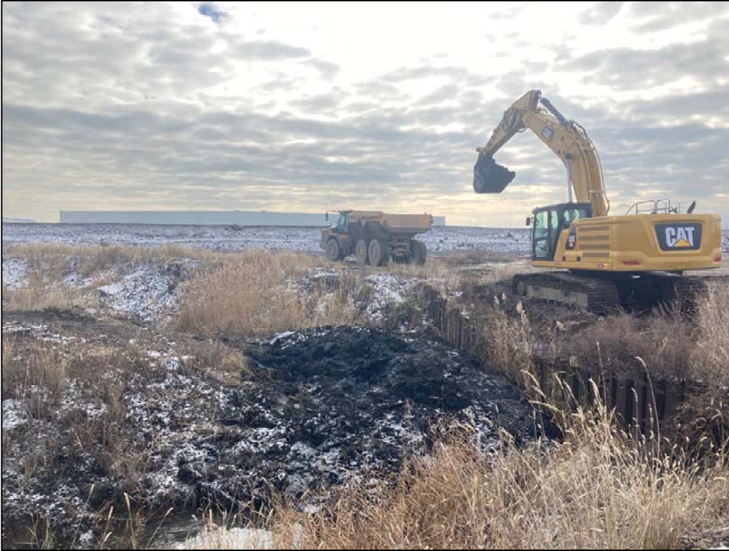
121820-1: Excavated material piled for drying within the lagoon.
