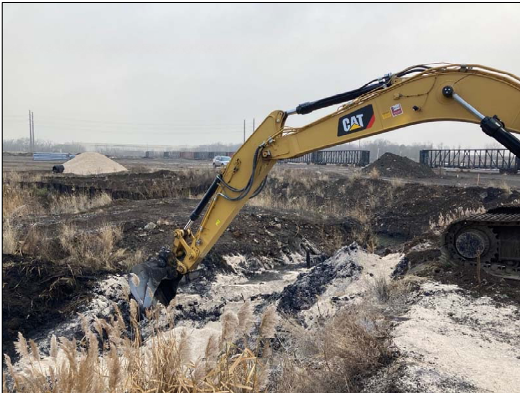
122120-1: Excavated material combined with calcite to accelerate the drying process.
