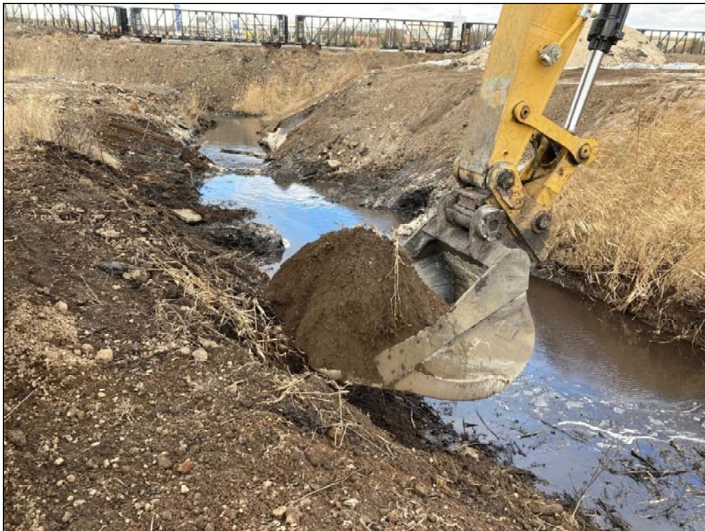
122220-3: Material collected from the lagoon sidewall for confirmation sampling. Material from the lagoon sidewalls did not have the oily appearance of the material from within the lagoon's channel bottom.
