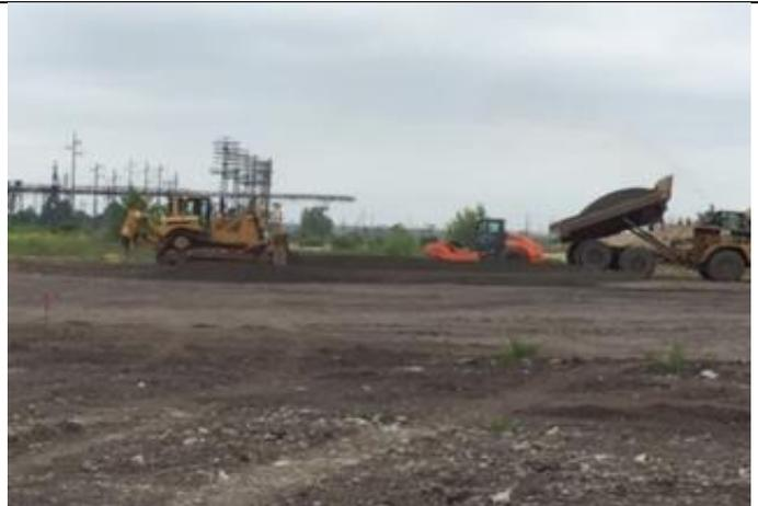
Figure 4: G&S placing slag for fills.
