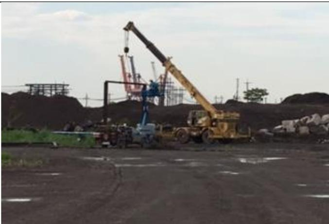
Figure 3: TPA installing water truck access pipe.
