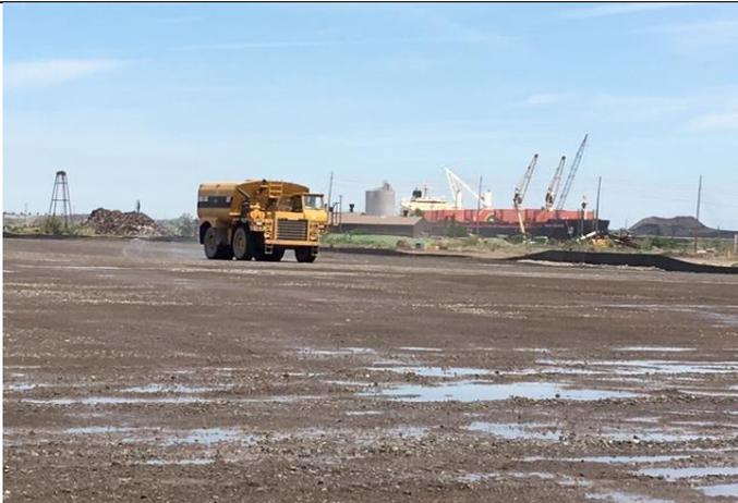
Figure 3: Watering slag for dust control.
