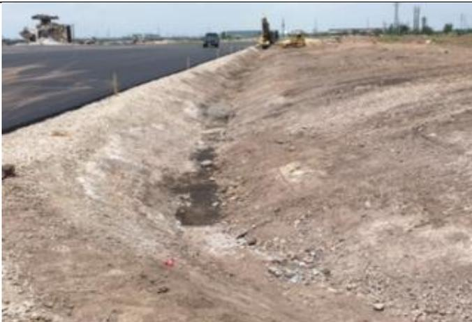
Figure 5: Excavation along storm swales on east side.
