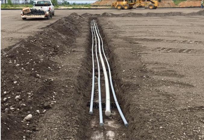
Figure 1: Installing underground electrical conduits for light poles.
