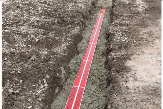
Figure 2: Concrete encasement and tracer tape over electrical trench.
