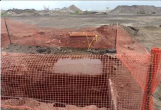
Figure 5: Main valve tie in for domestic water installation.
