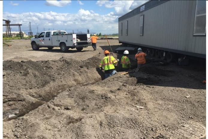
Figure 2: Installing the plumbing line to the trailer.
