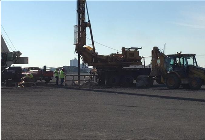
Figure 3: Drilling pole bases for 100’ light poles.
