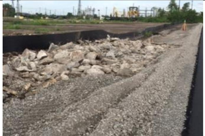
Figure 2: Demolished concrete (unforeseen) in the swale. Concrete removed for storm structure installation.
