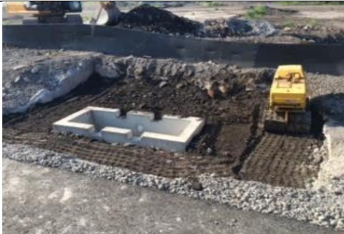
Figure 3: Installation of storm structures in swales.
