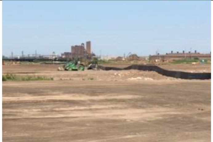
Figure 2: Silt Fence installation progress along the south side of the site.
