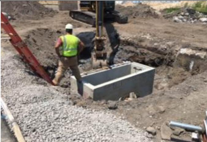
Figure 3: Storm structure installation and backfilled.
