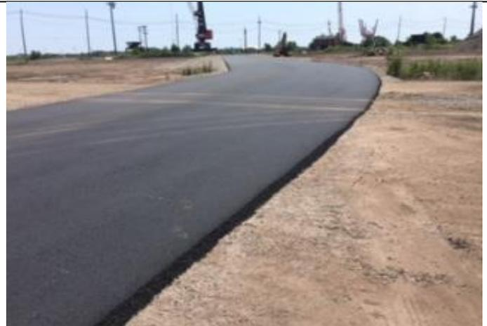
Figure 4: Asphalt paving along the northern half of the stern road. Awaiting final design to complete tie-in.
