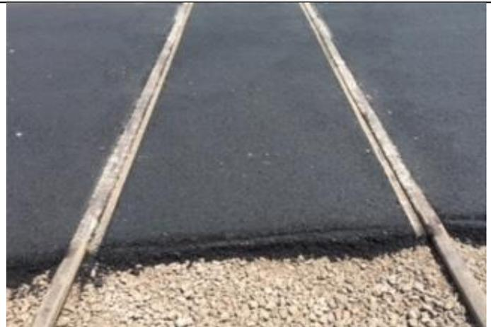
Figure 6: Paving tie-in at railroad crossing.
