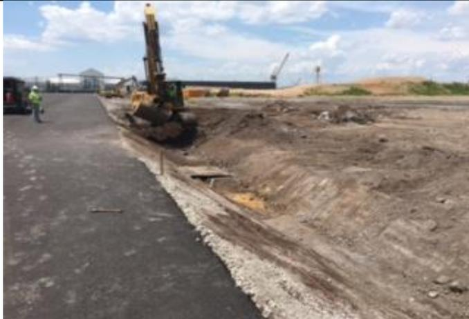
Figure 1: Continued grading of storm swales around the site.
