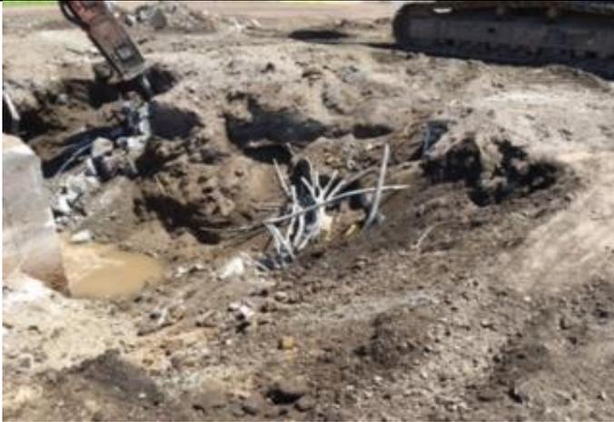
Figure 1: Unforeseen concrete and rebar during excavation.
