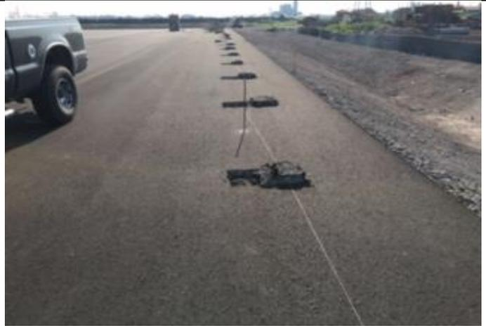
Figure 2: Cutting asphalt for fence post installations.
