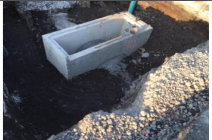
Figure 4: Backfilling and compacting around storm structure installations.
