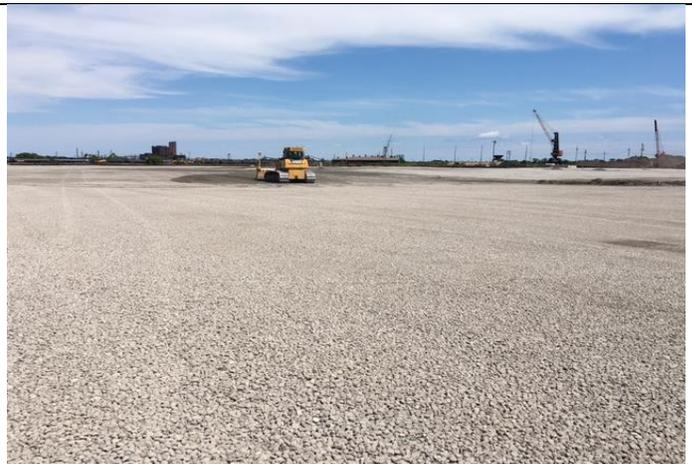
Figure 6: Installing GAB subbase for paving.
