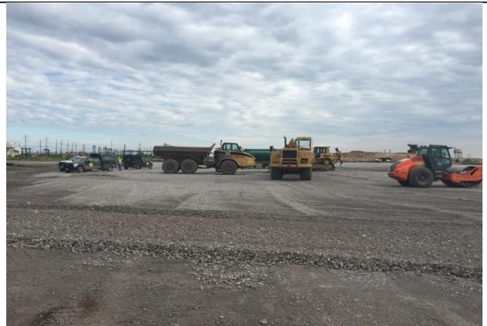
Figure 6: Compacting slag base.
