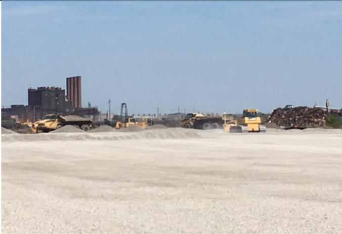
Figure 1: Continued installation of GAB subbase for paving.
