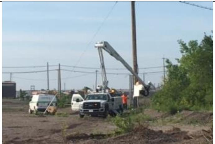
Figure 4: Installing temporary power for the trailer.
