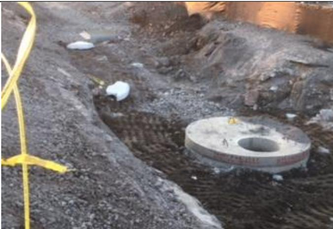
Figure 5: Backfilling the last inlet.
