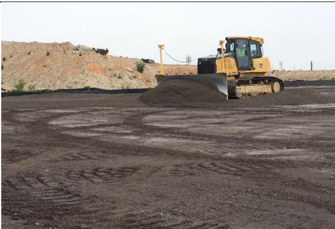
Figure 5: Grading steel slag.
