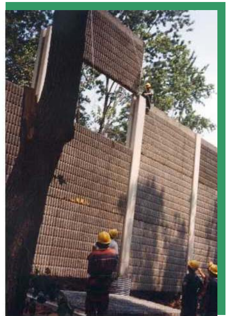
Highway Soundwall Barriers constructed from Scrap Tires
