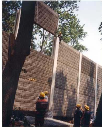
Highway Soundwall Barriers constructed from Scrap Tires
