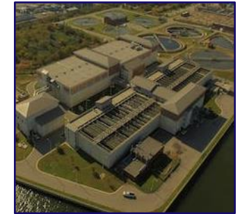
Waste heat capture
