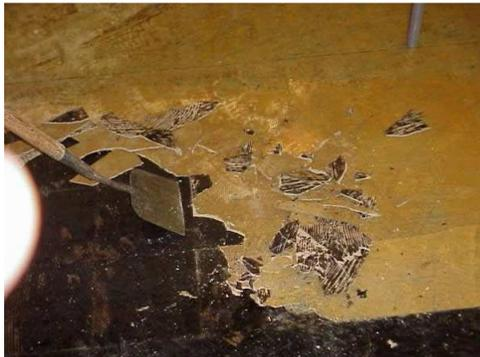
**Photo #8** - The floor tile in this picture may have been removed nonfriably and then placed in a lined fiber drum. The work crew used a hand tool to break up the floor tile in order to fit more into the drum. The floor tile has now become friable during the handling process. The floor tile needs to remain nonfriable from removal until it is disposed of.
