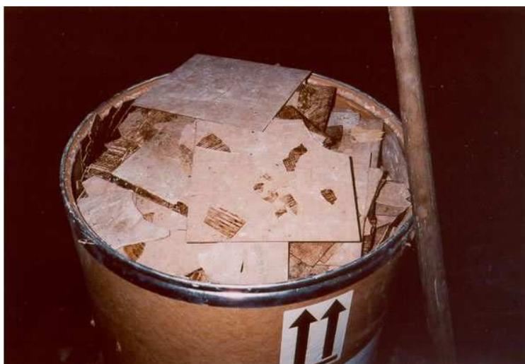
**Photo #9** - The floor tile in this picture may have been removed nonfriably. Even though the floor tile was removed as a nonfriable material, it has the potential to become friable during the handling process. The floor tile needs to remain nonfriable from removal until it is disposed of.
