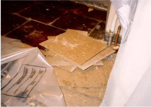
**Photo #2** - This asbestos-containing floor tile was removed with an ice chipper. The tile remained in whole pieces with little breakage.
