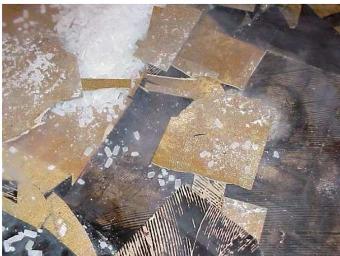
**Photos #5 & #6** - The floor tile in these photos are friable. It was removed with the hand tools that can be seen near the top of Photo #6. Floor tile being removed in this manner must be removed according to the MDH Asbestos Abatement Rules.
