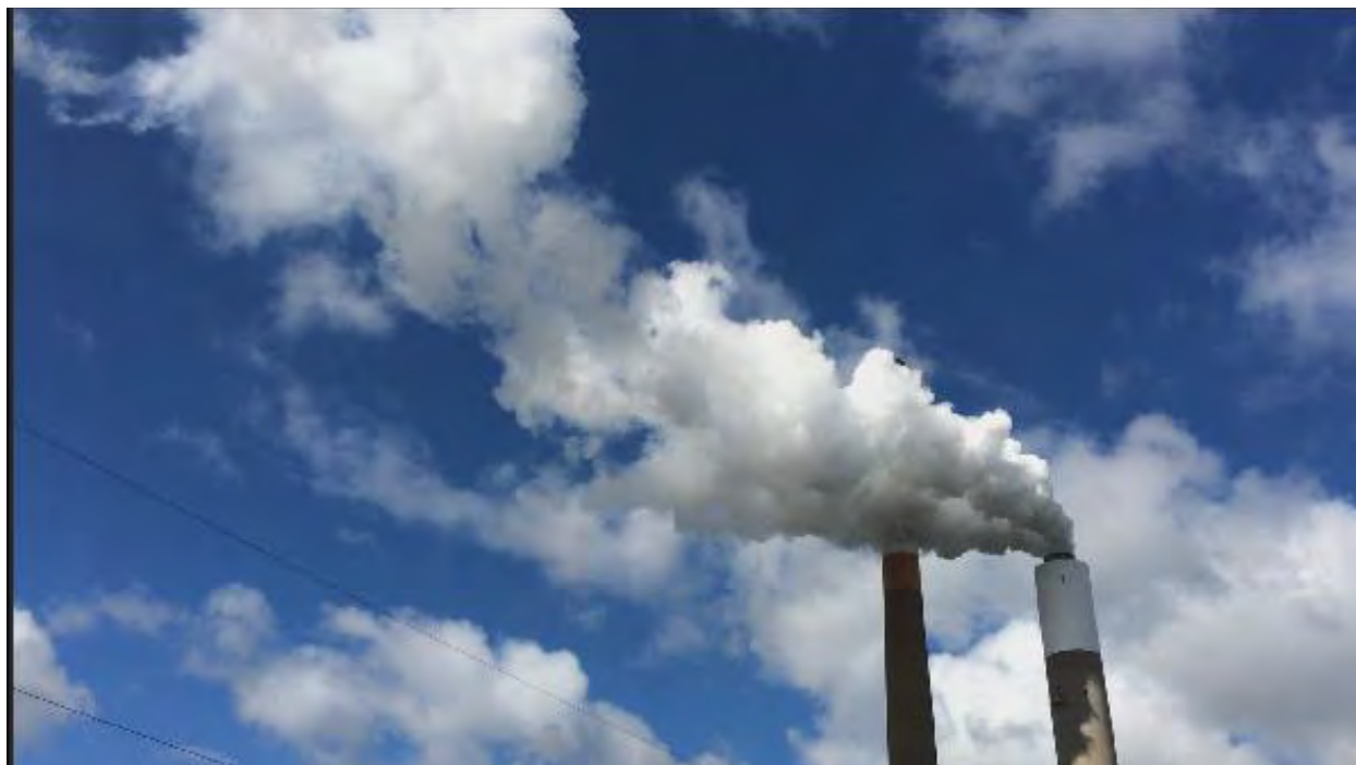
Figure 3-2: Example of Moist Plume Trajectory Lifting Due to Condensation
