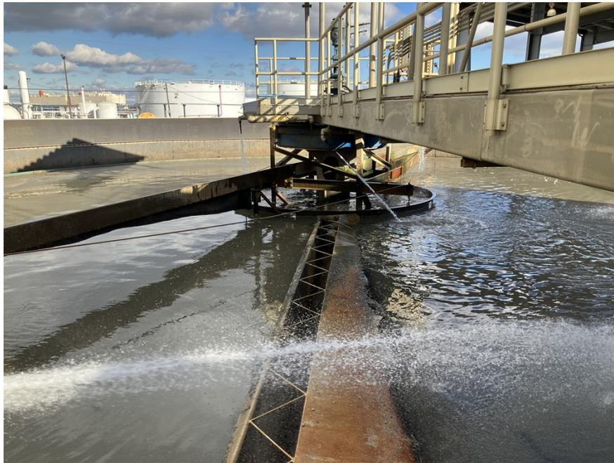
Image 2: GST #1, Broken & missing skimmer flaps.
