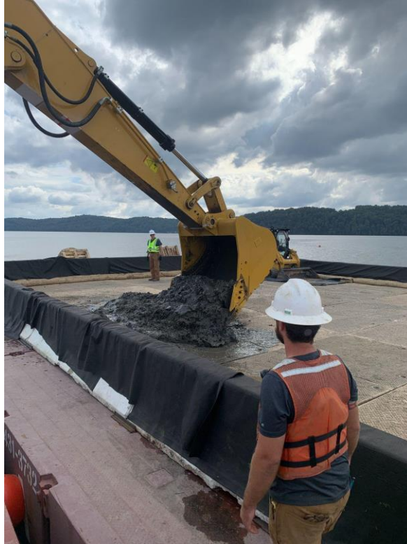
Figure 12: Dredging component of Maryland Innovative Reuse and Beneficial Reuse Pilot, October 9, 2021.
