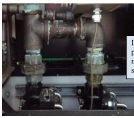
Improperly installed product pipe manifold above the shear valves
