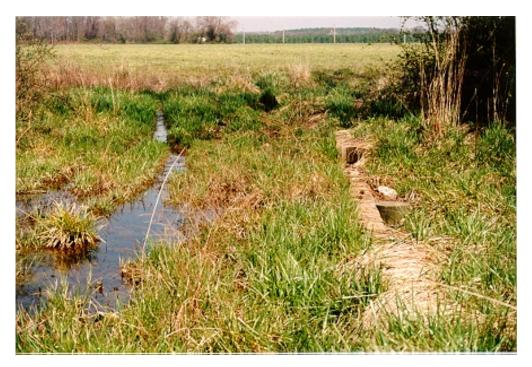
Figure G.26: Timber weir along hedgerow to control drainage (photo Noble 1/98)
