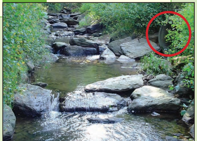
Figure 8. A steep concrete channel was replaced with a series of step-pool structures. This sequence of small pools (visible in the photo on the right) slows stream flow, disperses energy during storms, and provides a stable, naturally functioning channel with improved habitat. (Note the outflow pipe on the right-hand side of both photographs.)
