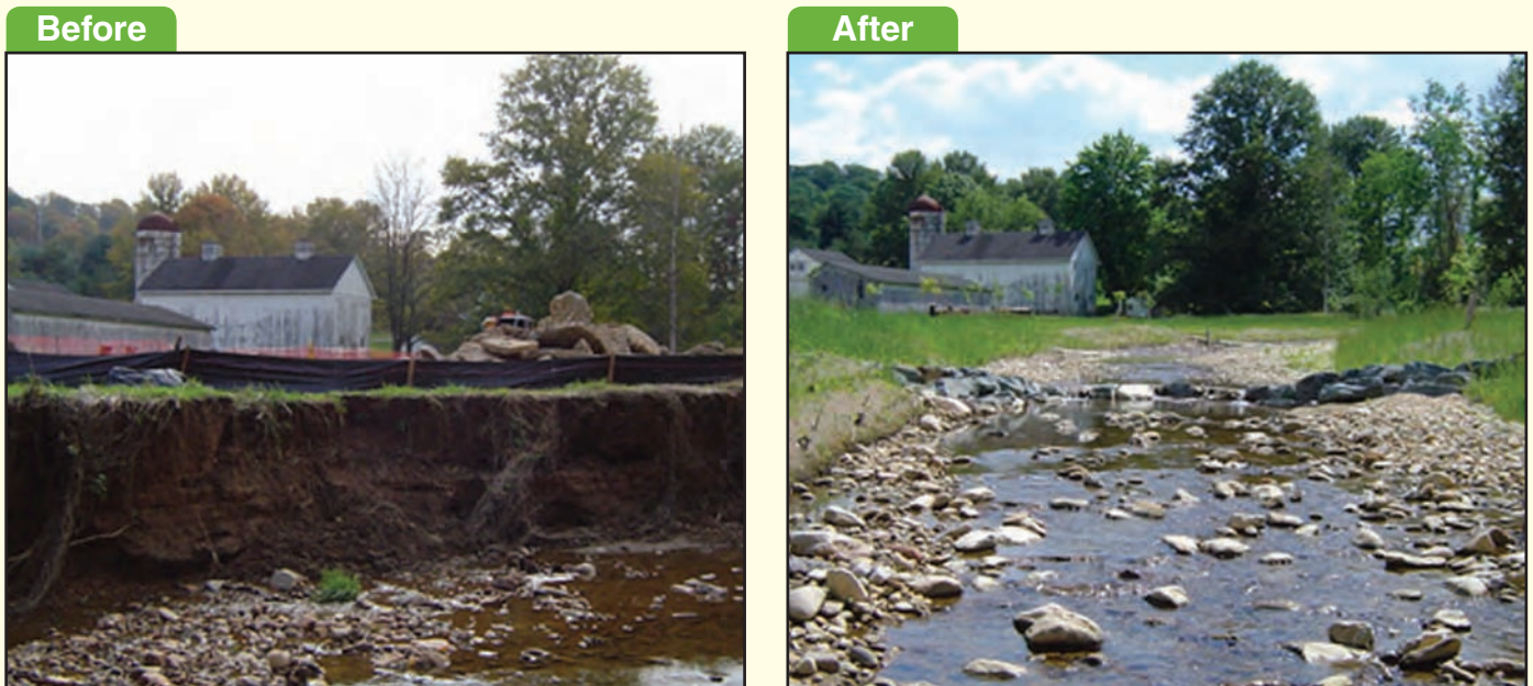
Figure 9. A severely eroded bank caused in part by agricultural activities was restored by regrading the streambank, installing rock grade-control structures (to prevent bed degradation), and establishing riparian buffer.
