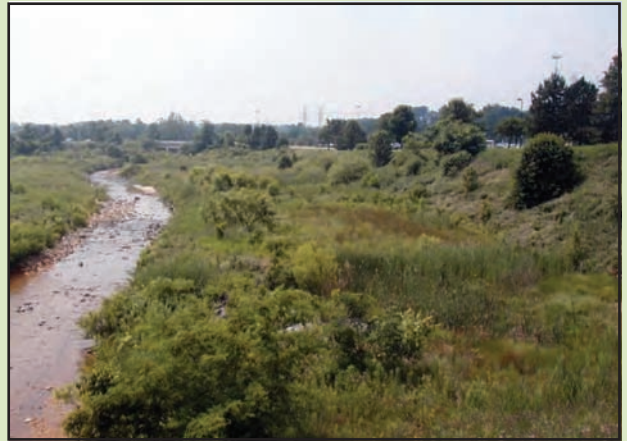
Figure 6. Natural stream/floodplain interactions restored along with the creation of adjacent stormwater wetlands.
