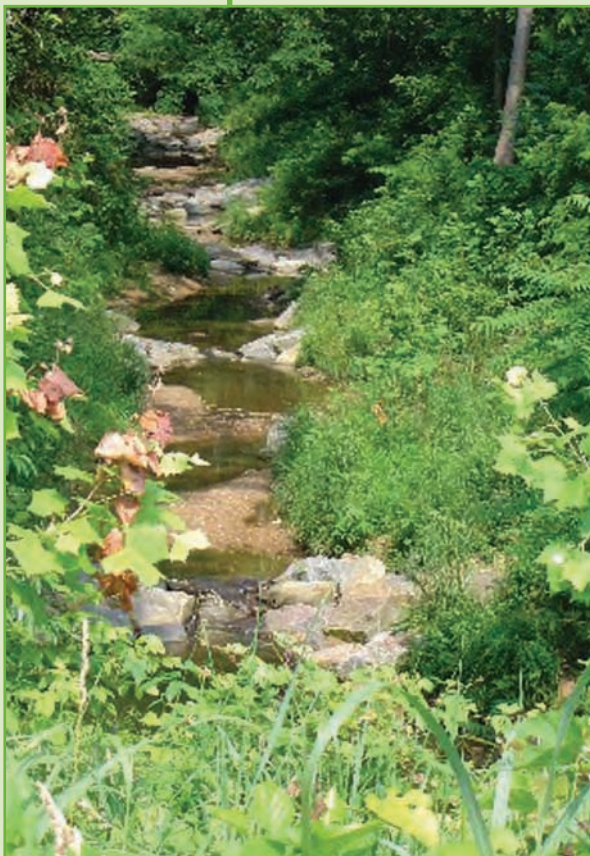
Figure 12. Minebank Run (Phase I) stream restoration three years after construction.
