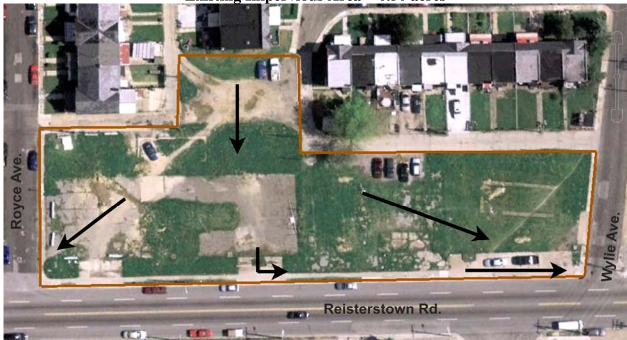
Figure 1. Site Conditions before Redevelopment Existing Impervious Area = 0.50 acres
