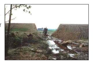
A dam is defined as any obstruction, wall, or embankment, together with its abutments and appurtenant works, constructed for the purpose of storing water. Dams may be constructed of earth, concrete, wood, or rock. Most dams in Maryland consist of an earthen embankment to store water and a combination of spillways designed to pass water safely around or through the facility.
