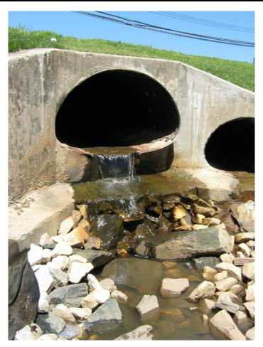
Figure 3-23: Very Severe Exposed Fish Migration Barrier (rating = 1)
