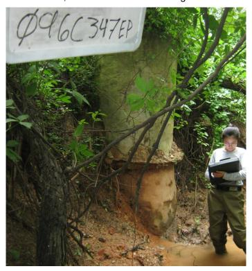
Figure 3-21: Examples of a Potentially Severe Exposed Pipe Problem (rating = 2)
