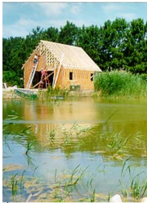
Captains Knoll under construction
