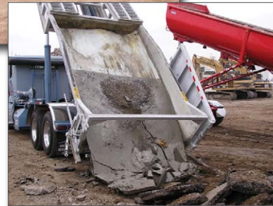
Figure 15. Delivering hardened Concrete to a recycler
