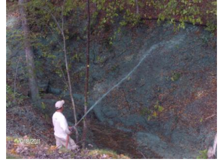
Ravine 3 - During Restoration
