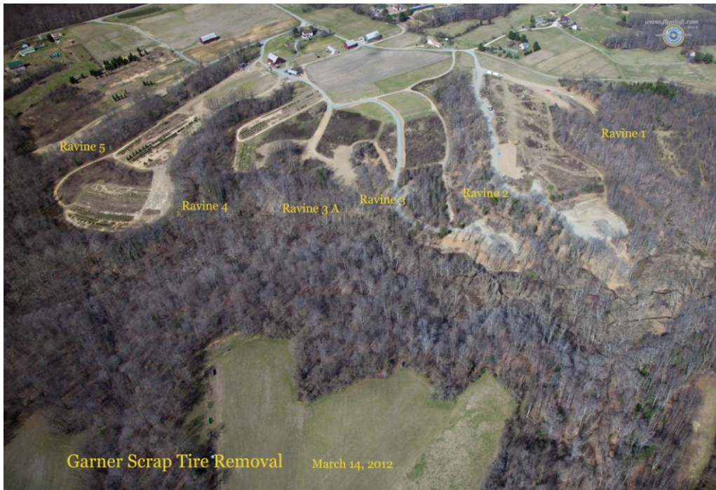
Aerial Photo of Entire Site During Cleanup
