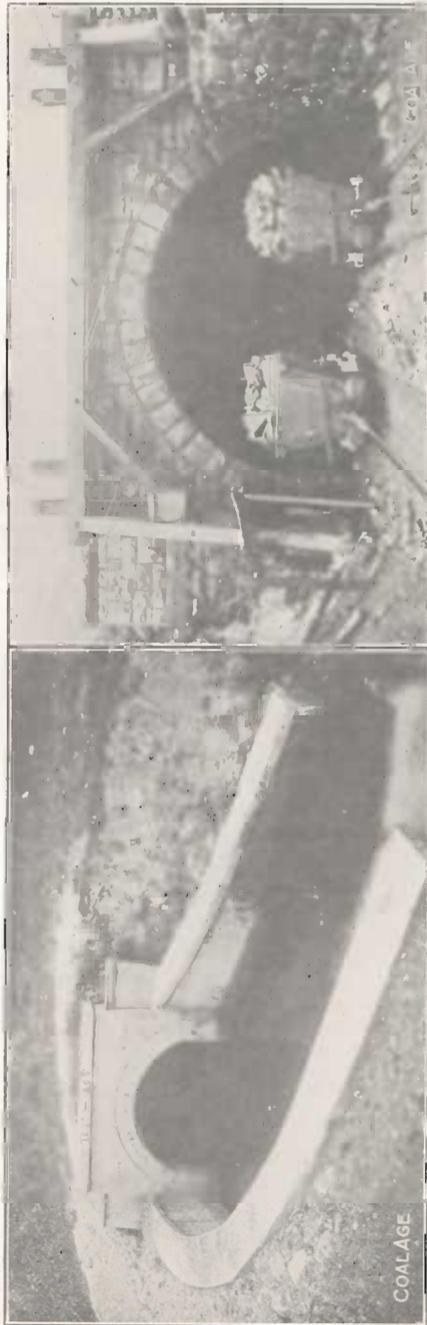
Drainage Tunnel Draining the Big Vein Seam at Clarksville.
