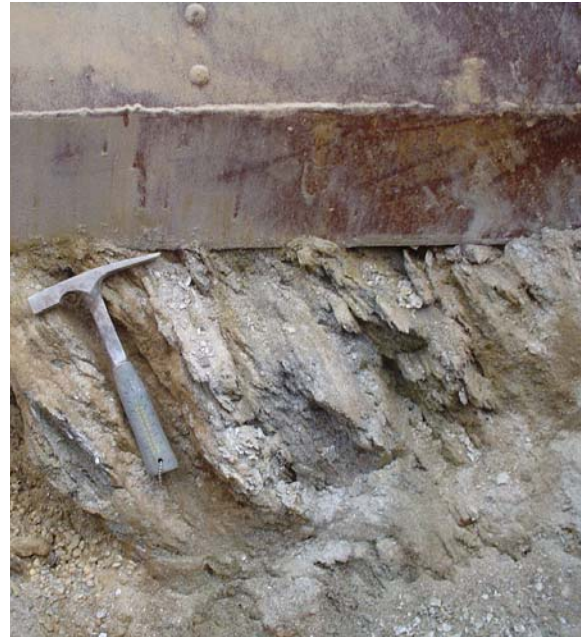
Photo 1: Bedrock foliation looking southwest in tank field excavation.
