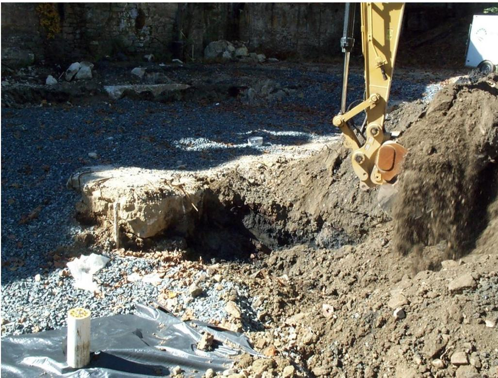
Photo 2: 10/23/12 Excavation along footer wall, adjacent to MP-11
