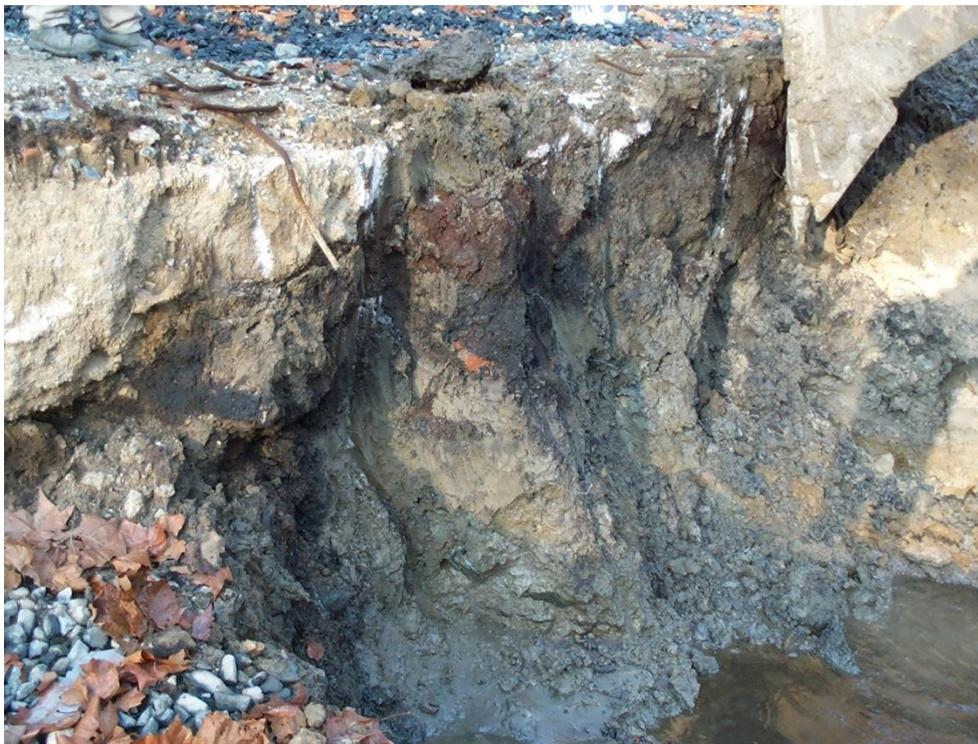
Photo 4: Staining visible along footer wall
