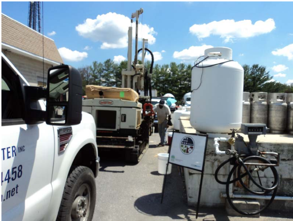
Photo #5 Soil Boring B-8, at United Propane, Inc., looking south 06/15/12
