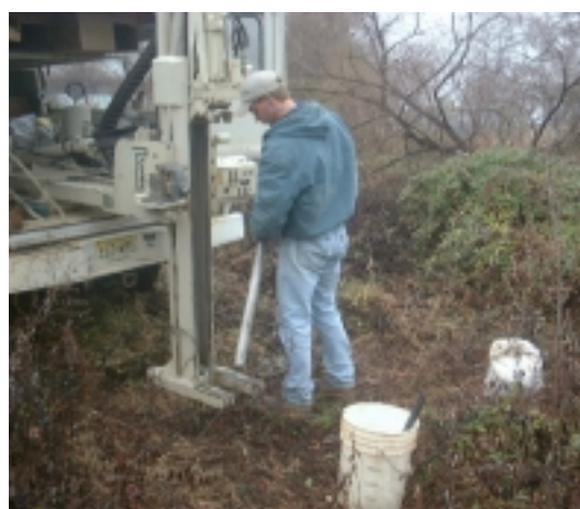
Direct push technology at work to collect a groundwater sample at the Sauer Dump site.
