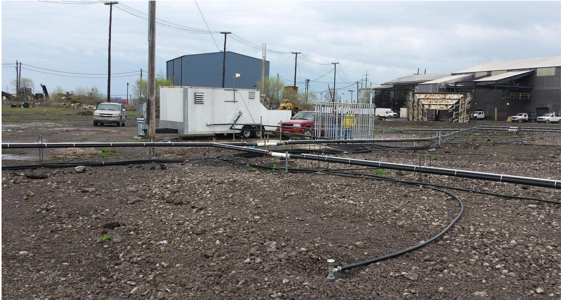
Cell 1 Piping System Completely Replaced and New Sparge Wells Added
