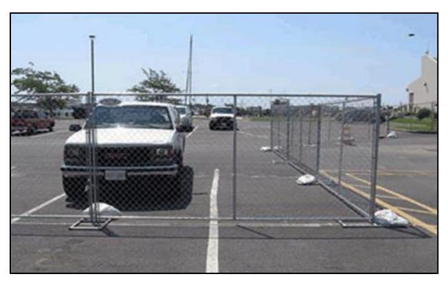
Non-Ground Intrusive Chain Link Temporary Storm Fencing Sample Photograph
