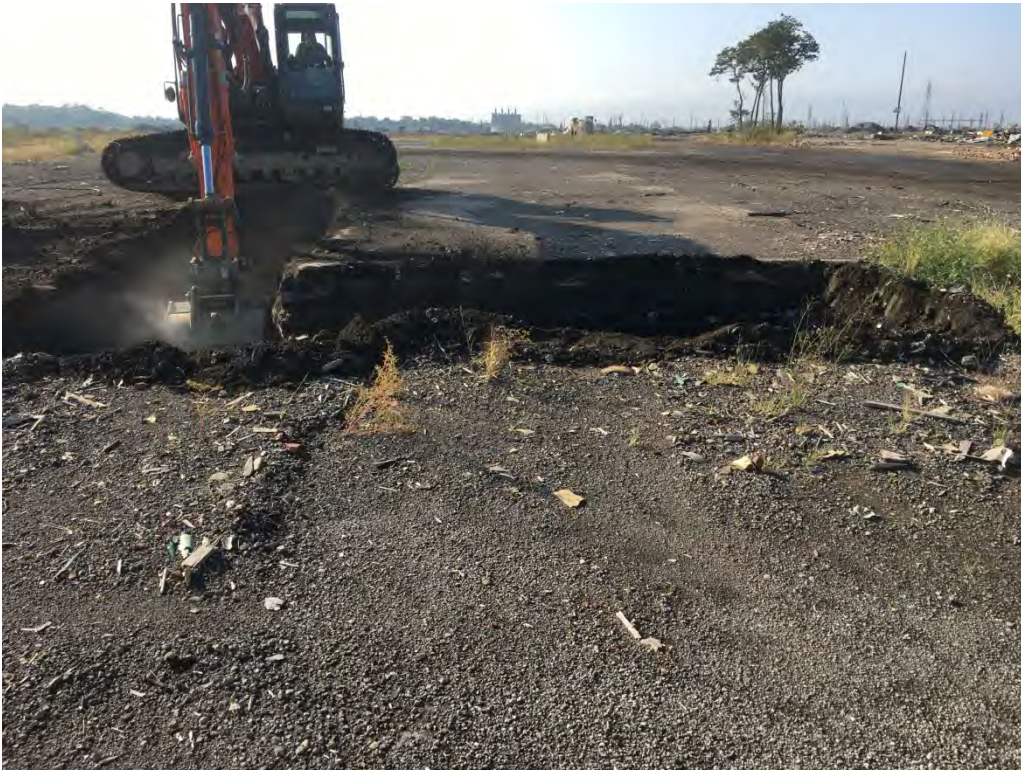
View of the excavation activities at B22-148 excavation.
