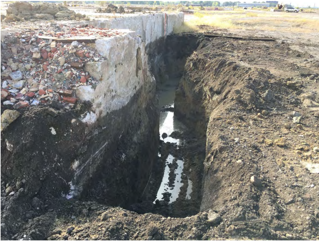
View of the west excavation, facing south, to confirm the horizontal extent of impacts.
