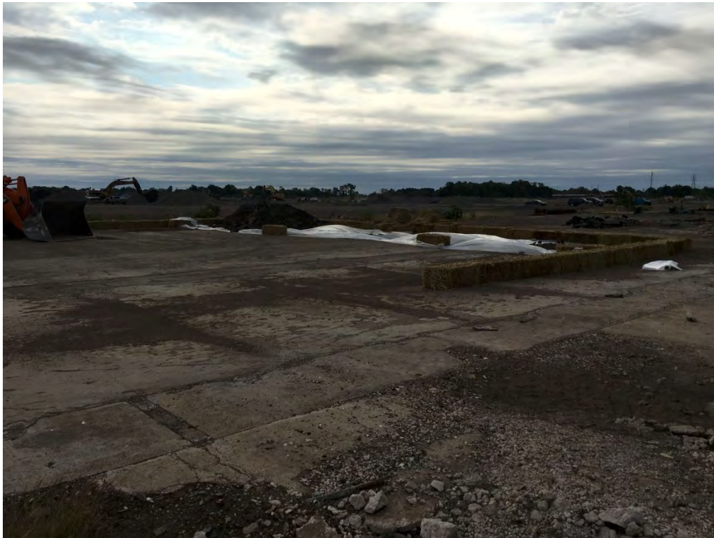
View of the PCB stockpiled material area setup prior to placement of impacted material. Poly is setup along the ground surface with hail-bails used as berms.
