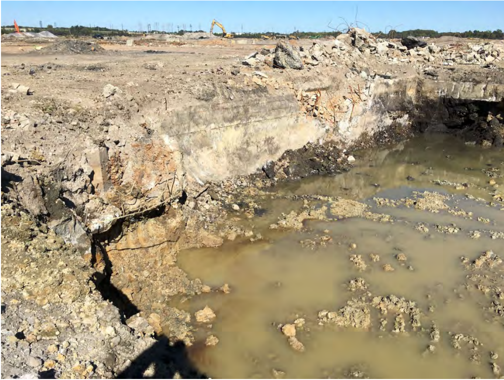
View of the west wall of the completed excavation.
