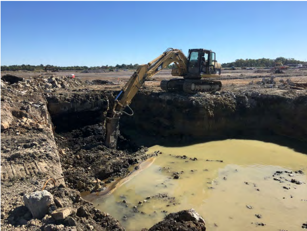
View of the east wall of the completed excavation.
