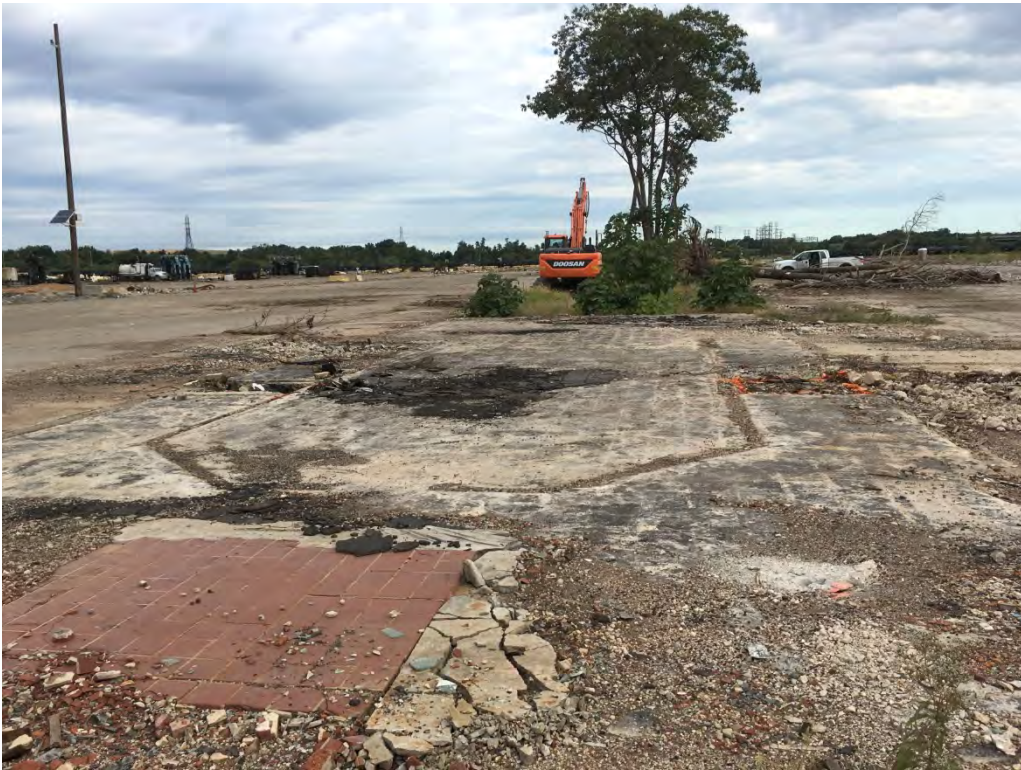
B22-028 Main excavation limits prior to removal of impacted material.
