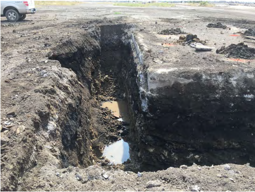
View of the eastern side of the excavation and interior east wall.
