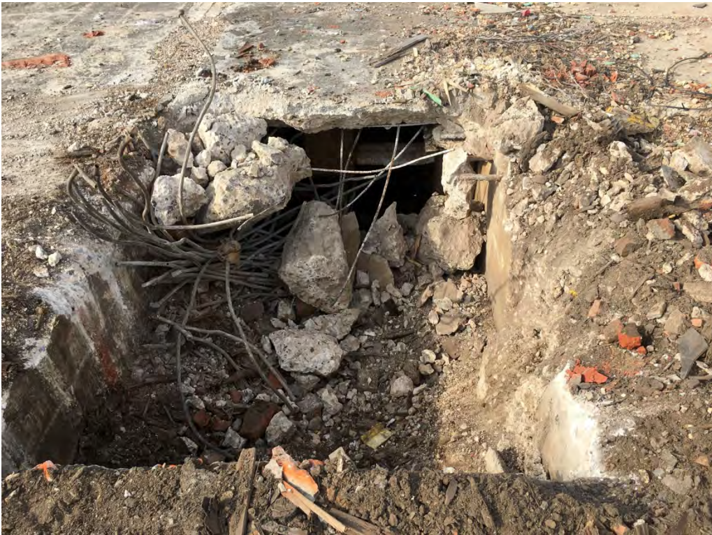
B22-028 South excavation completed to a depth of 2 feet below ground surface. Three of the four sidewalls composed of concrete, with no visible staining, and the northern portion of this excavation had no sidewall therefore only a bottom confirmation sample was taken.
