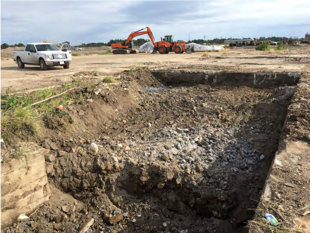
View of the south and east wall of the completed Main Excavation facing southeast.
