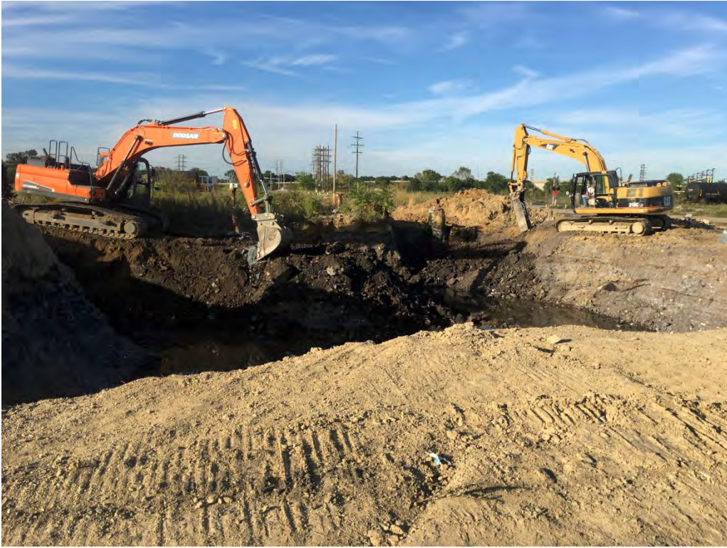
View of the MCM and ENR equipment completing excavation activities.
