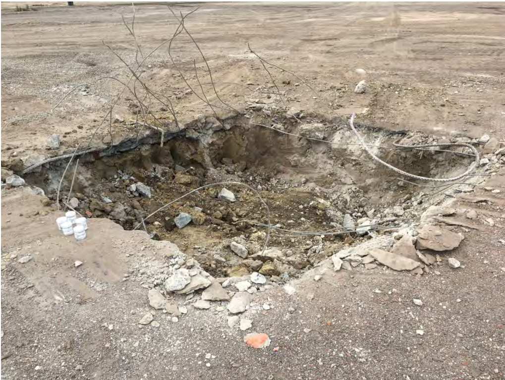
B22-065 excavation completed to a depth of 2 feet below ground surface. Four sidewall confirmation samples and one bottom confirmation sample was collected.
