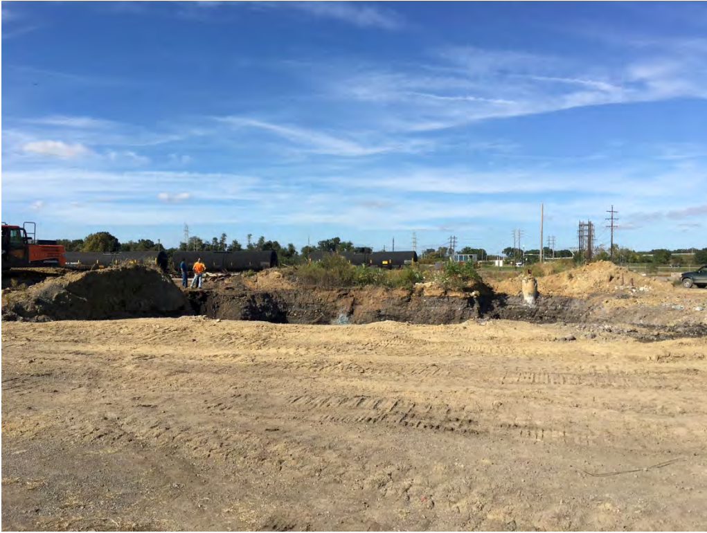
View of the completed excavation facing north.
