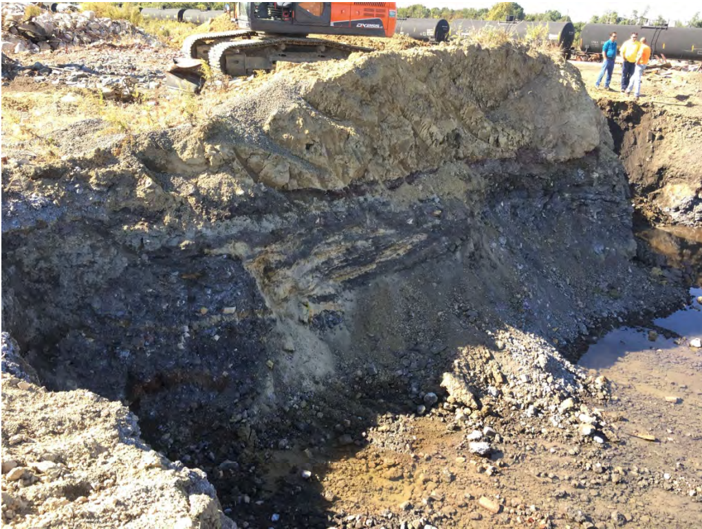
View of the west wall of the completed excavation facing northwest.
