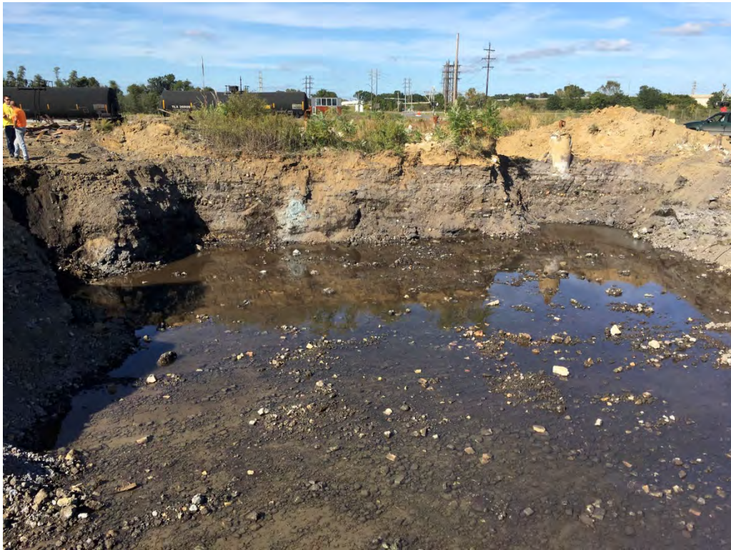
View of the north wall of the completed excavation facing north.
