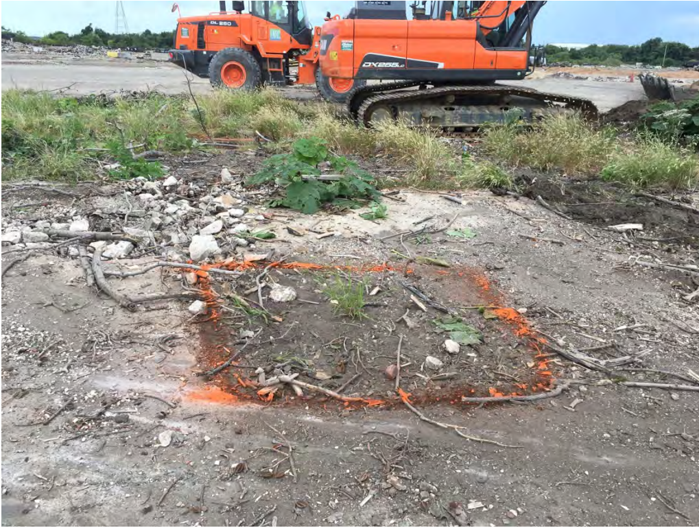
B22-028 East excavation limits prior to break up of the first 8-10" of the reinforced concrete pad and removal of impacted material.
