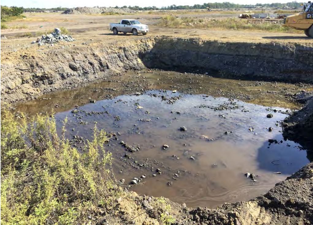
View of the completed excavation facing southeast.
