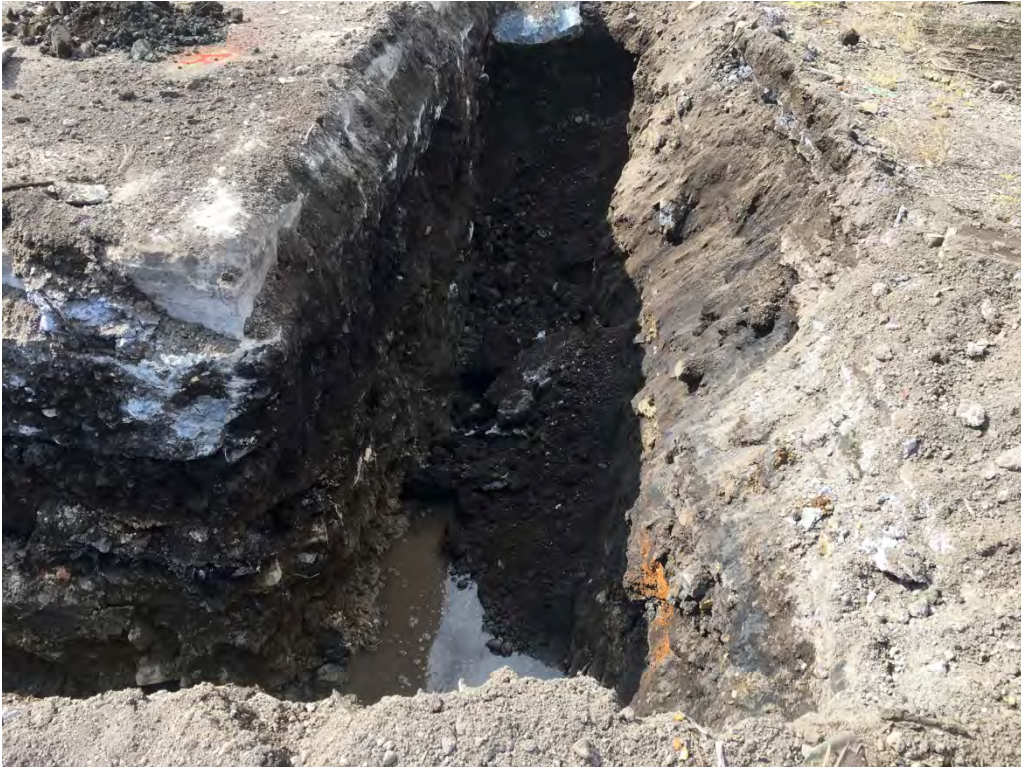
View of the northern side of the excavation and north interior wall.
