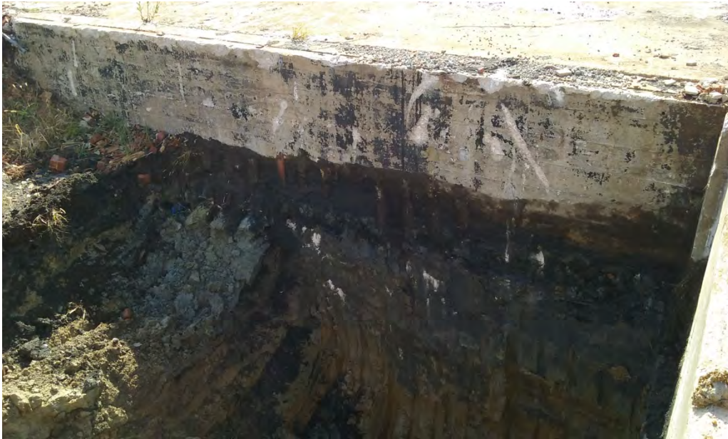
View of impacted material observed along the south wall of the main excavation area.
