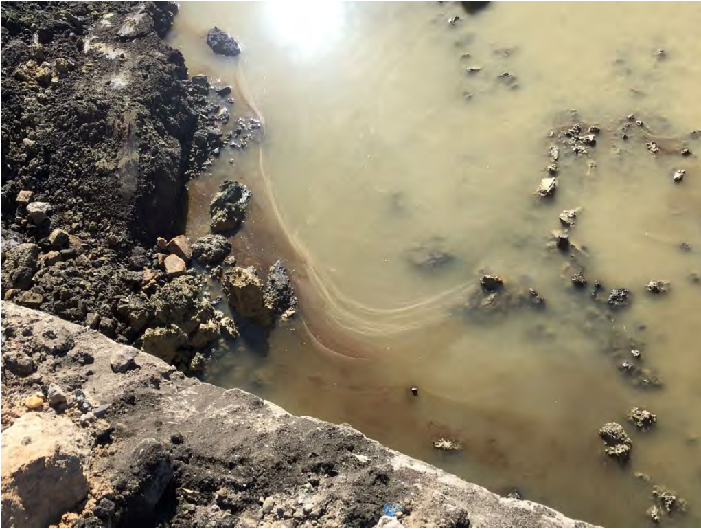
View of product observed on the bottom of the excavation.
