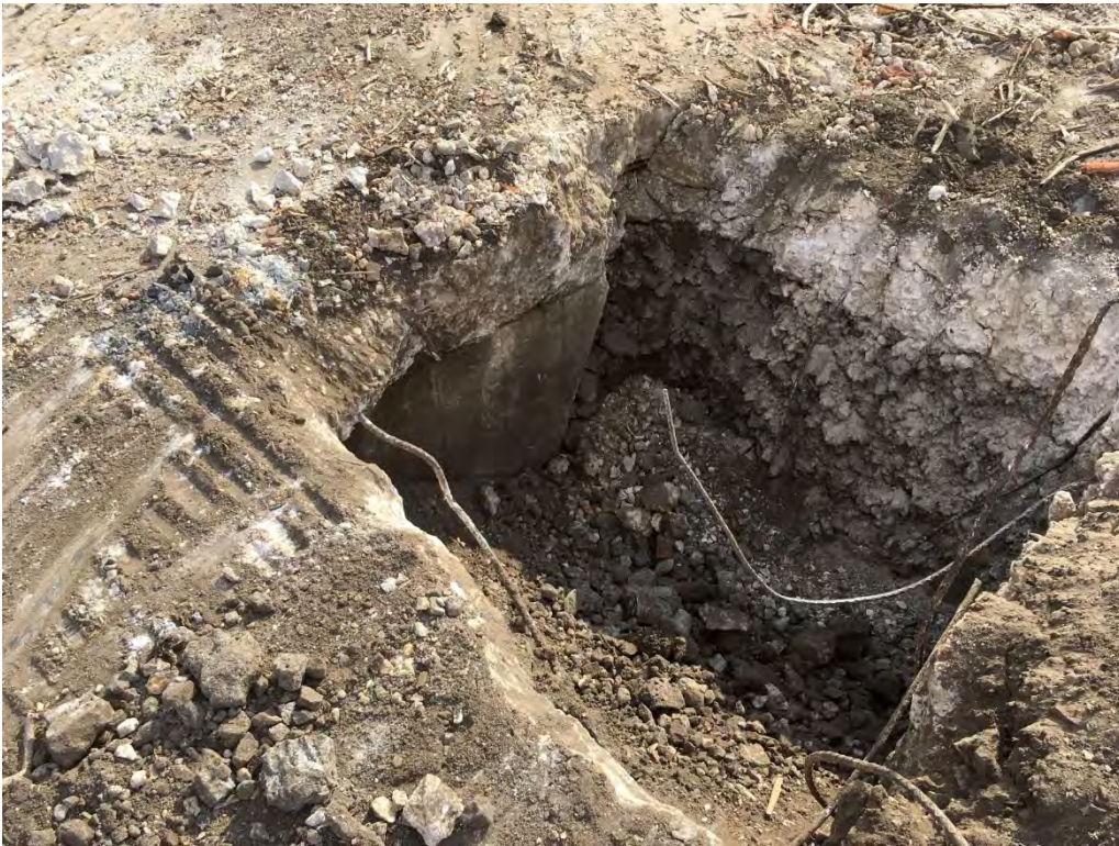
B22-028 East excavation completed to a depth of 2 feet below ground surface. All four sidewalls composed of either concrete, with no visible staining, and/or large gravel therefore only a bottom confirmation sample was taken.
