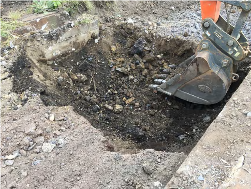
Impacted material observed in the middle of the Main excavation adjacent to the trench manhole. An additional three feet of impacted material was removed.
