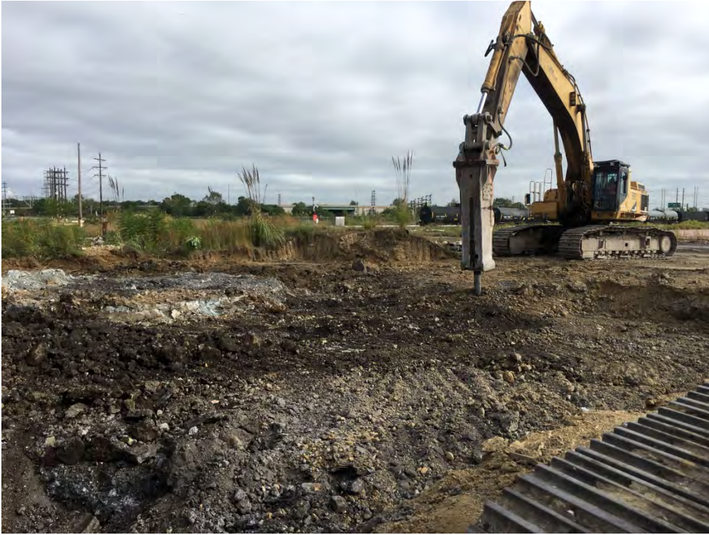
View of the MCM excavator with the jackhammer attachment used to break-up the slag throughout the excavation.
