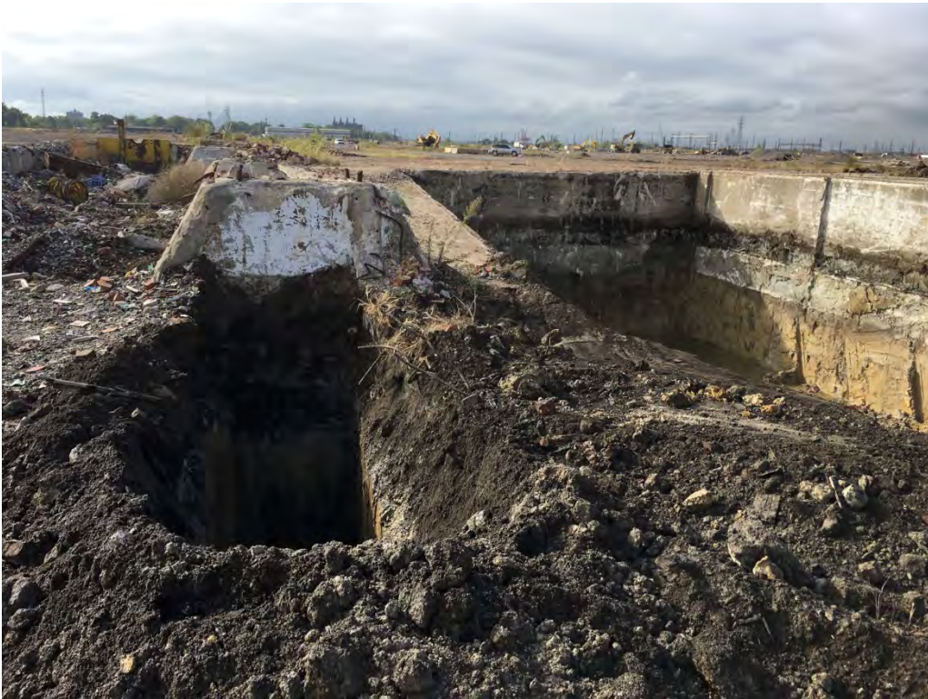
View of the location of the east excavation area facing south.
