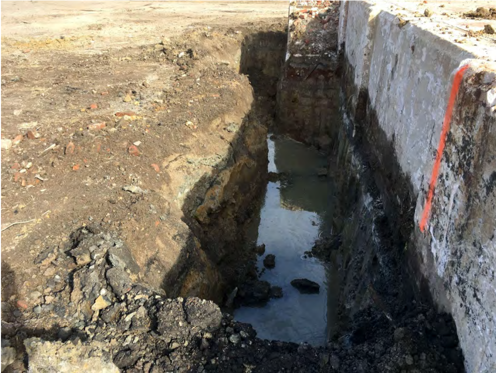
View of the west excavation, facing north, to confirm the horizontal extent of impacts.
