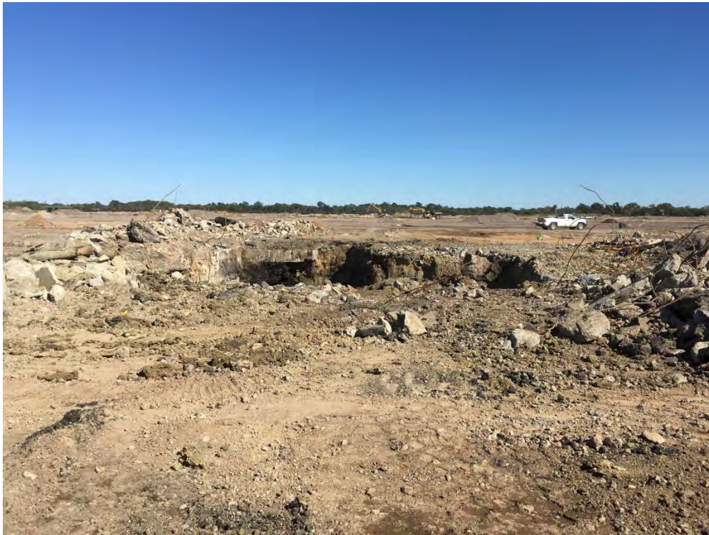
View of the completed B22-162 & B22-163 excavation facing east.
