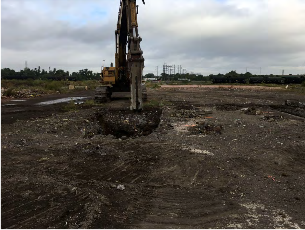
View of the MCM excavator with the jack hammer attachment used to break-up the french drain and slag.
