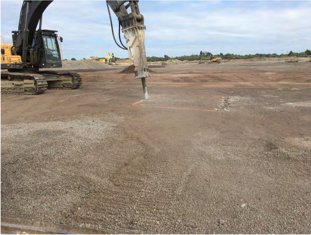
B22-065 excavation limits and use of hammer attachment to break up the first 8-10” of the reinforced concrete pad and removal of impacted material.
