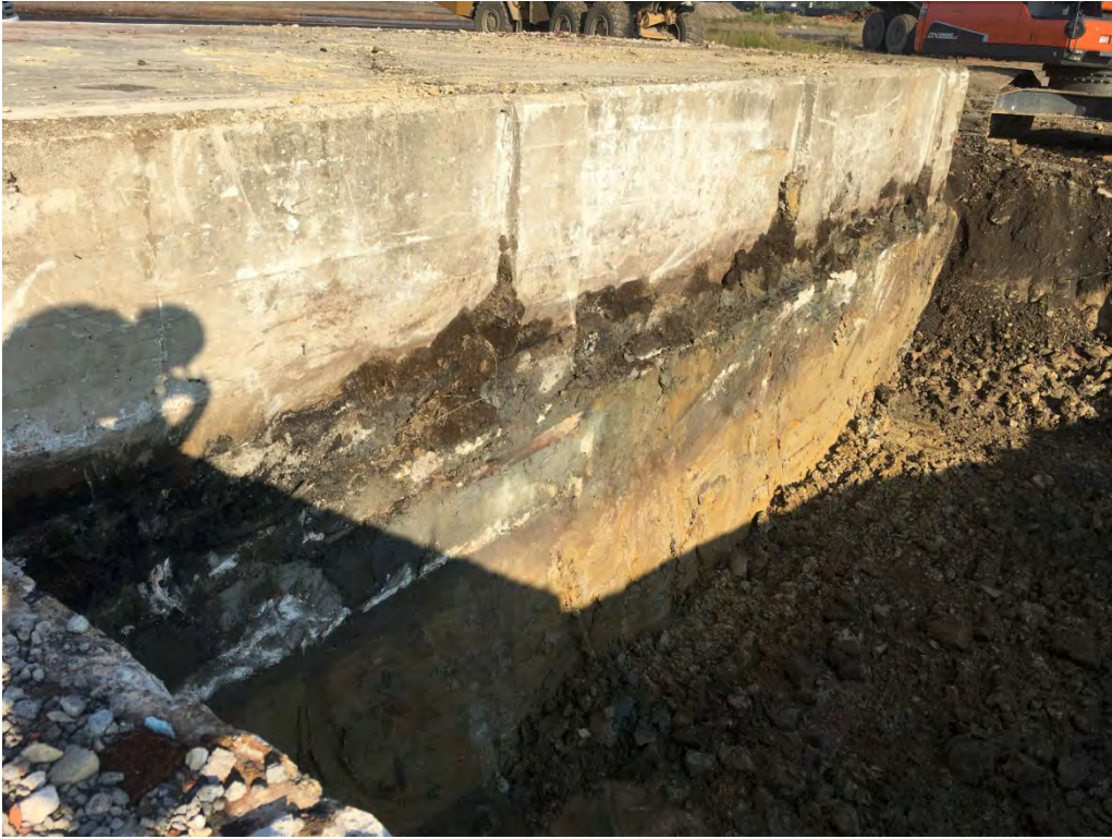
View of impacted material observed along the west wall of the main excavation area.
