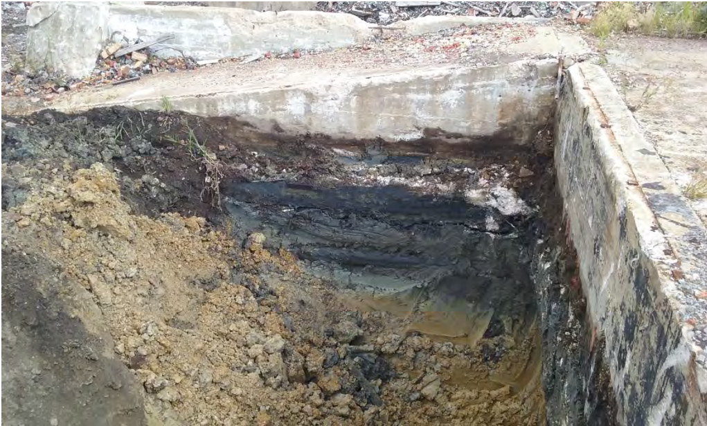
View of impacted material observed along the east wall of the main excavation area.
