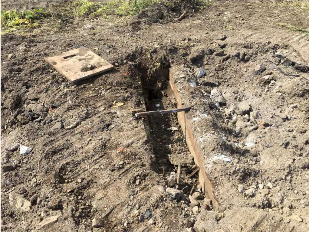
View of the french drain observed in the northwest corner of the excavation.
