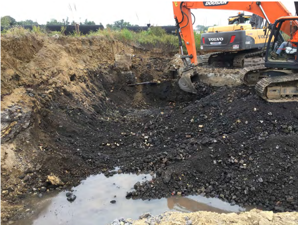
View of significantly impacted material, facing north, located adjacent to a potential fill pipe for the former tank. This area is located along the western wall of the excavation.
