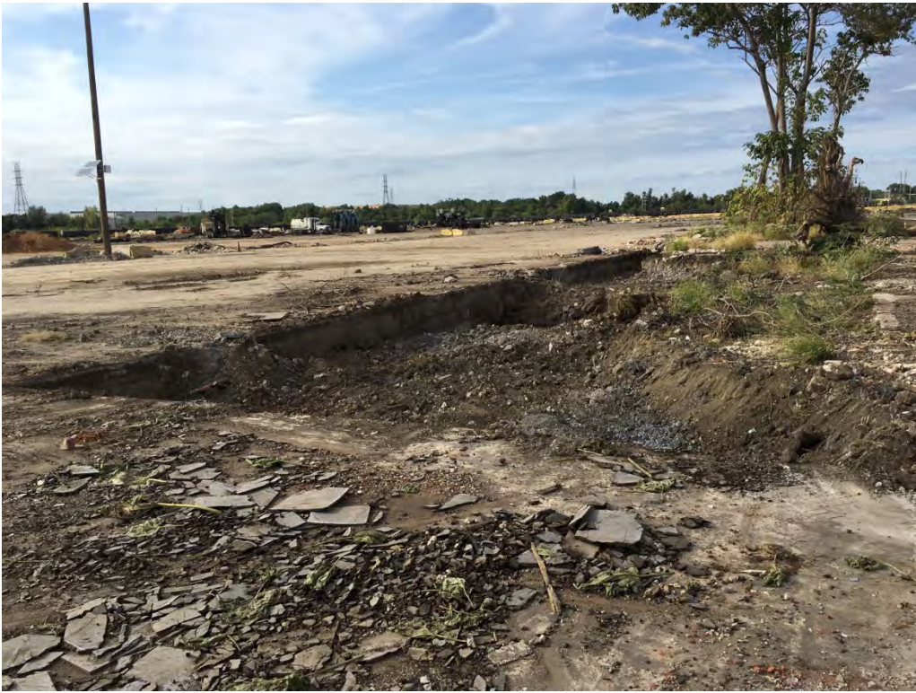
View of the east wall of the completed Main Excavation facing northwest.
