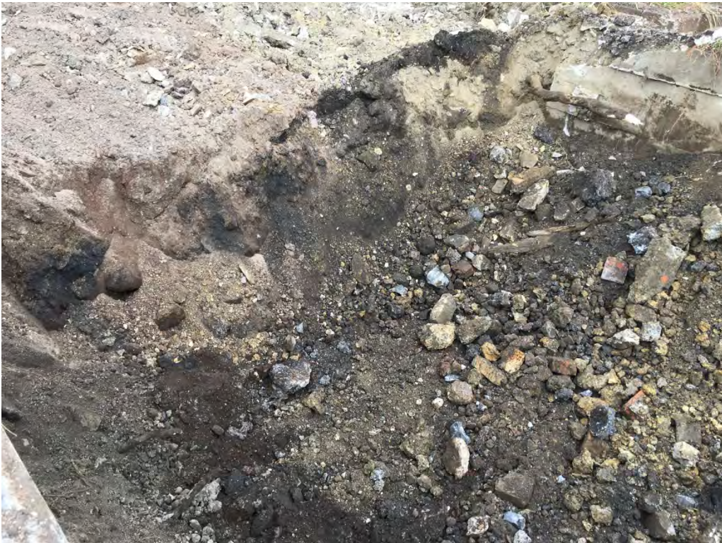
A view of the north wall of the additional impacted material observed in the middle of the Main excavation adjacent to the trench manhole.
