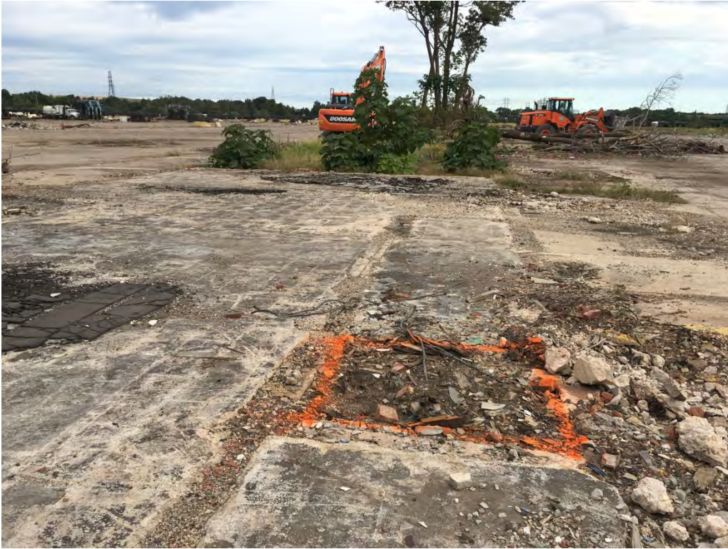
B22-028 South excavation limits prior to removal of impacted material.
