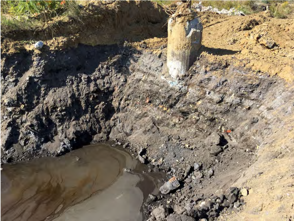
View of the northeast corner extension, due to significant impacts, and product observed on the bottom of the excavation.
