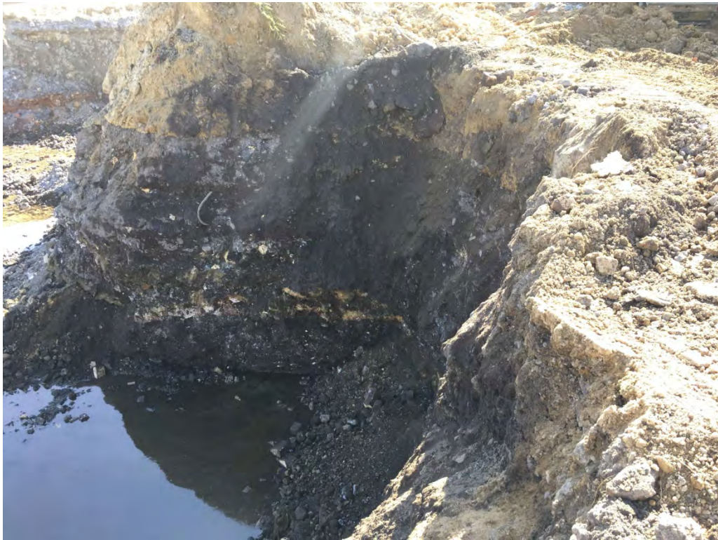
View of the west wall extension due to significant impacts observed. The product pipe was routed through this area.
