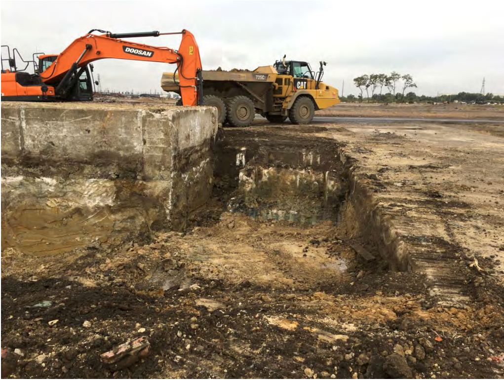
View of impacted material observed along the concrete box. The non-impacted benched area is located in front of the concrete box.
