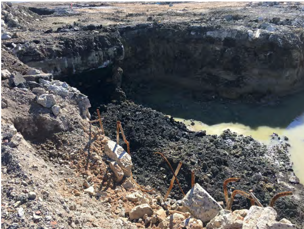
View of the east impacted material along the bottom in the northeast corner.
