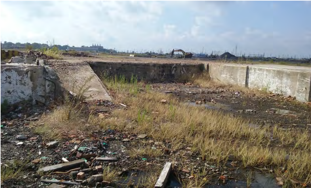
View of the B22-070 excavation, facing south, prior excavation activities.
