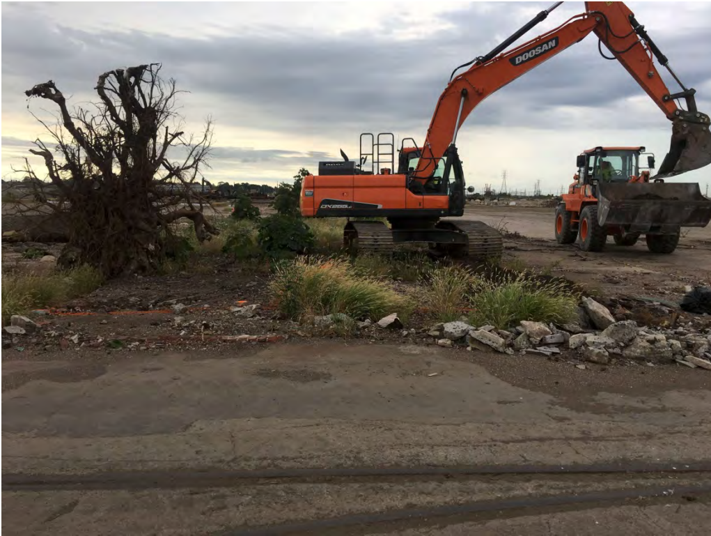
Excavation activities along the northern section of the B22-028 Main excavation.
