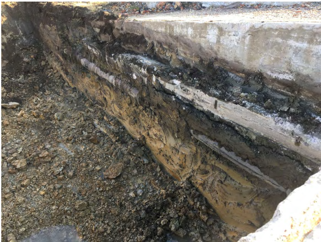
View of impacted material and the utility pipe observed along the east wall of the main excavation area. Highly impacted material was observed between the utility pipe and the bottom of the slab above it.
