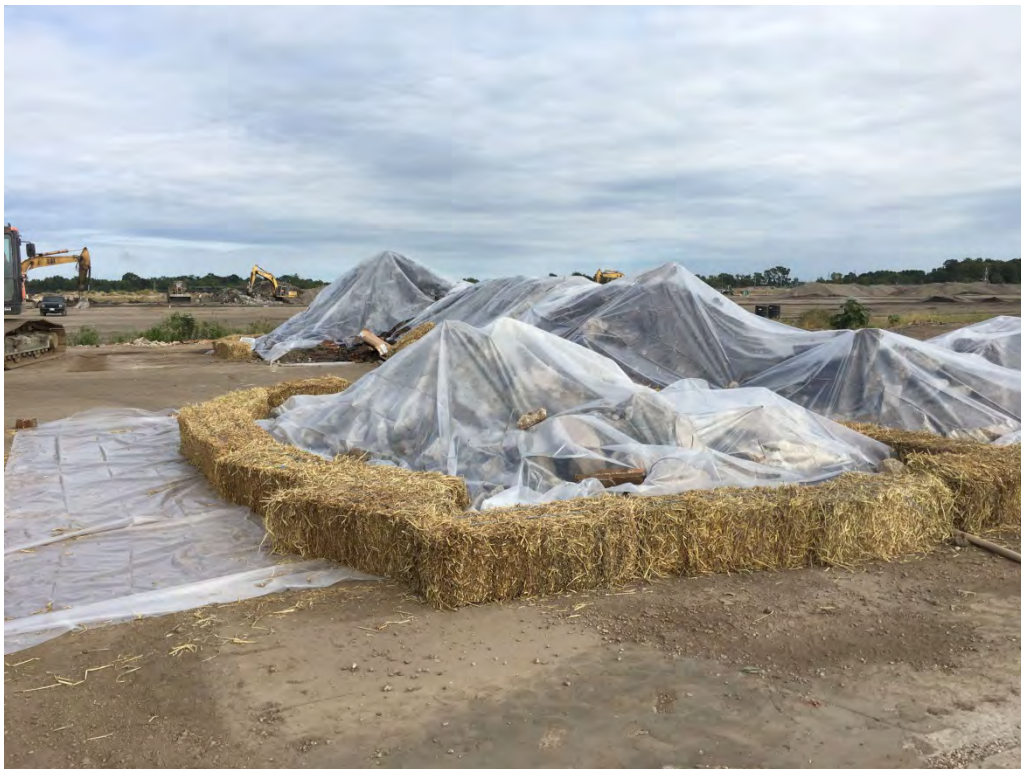
View of the covered PCB stockpiles at the conclusion of the PCB excavations. Soil and concrete materials were segregated and stockpiled separately.
