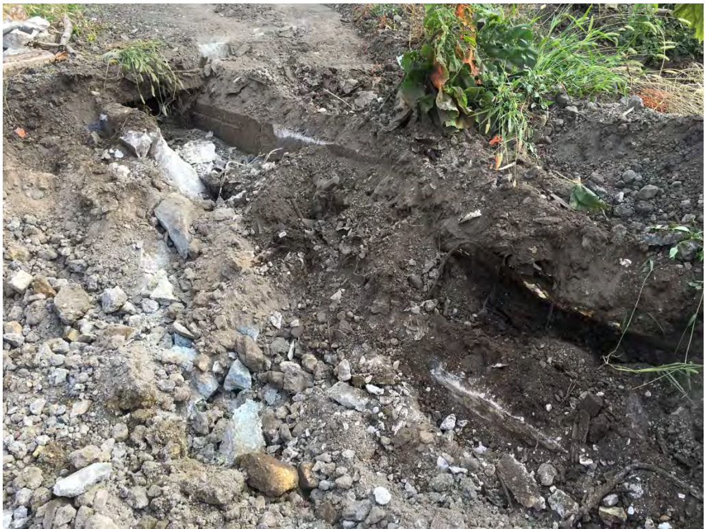
View of the french drain observed within the Main excavation. The french drain extends from the north wall to the south wall within the excavated area.
