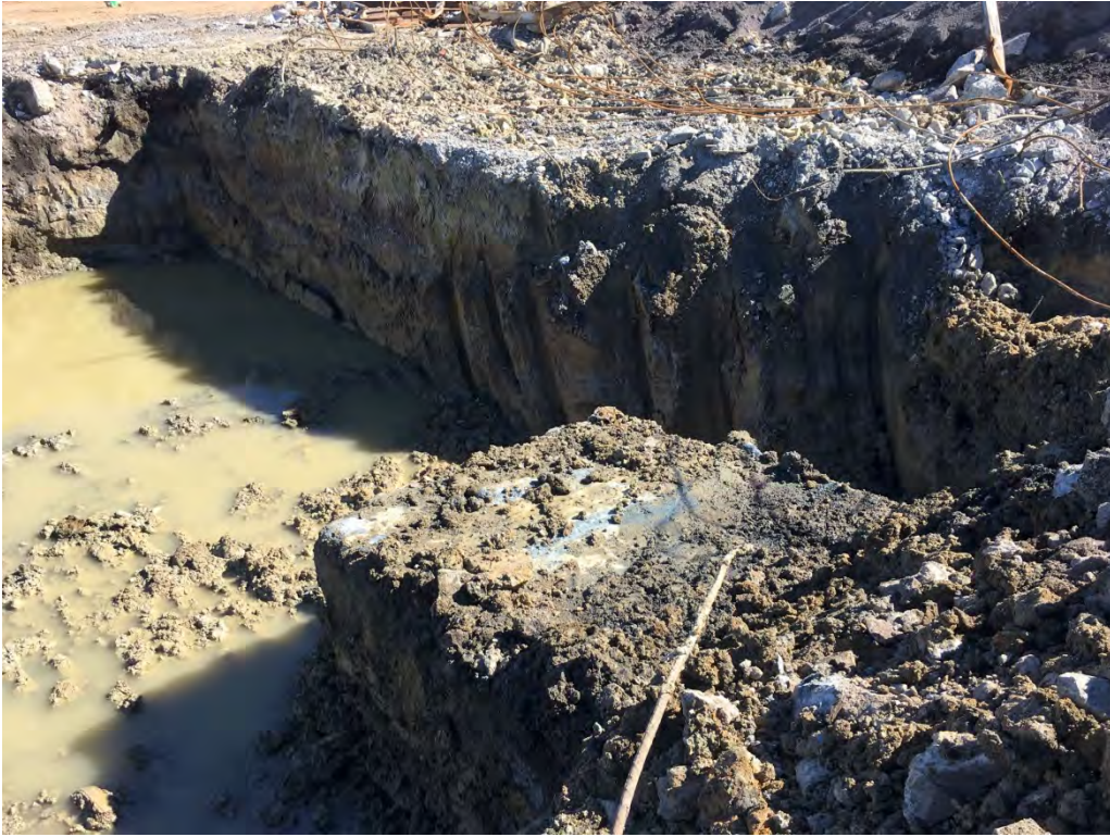
View of the south wall of the completed excavation.
