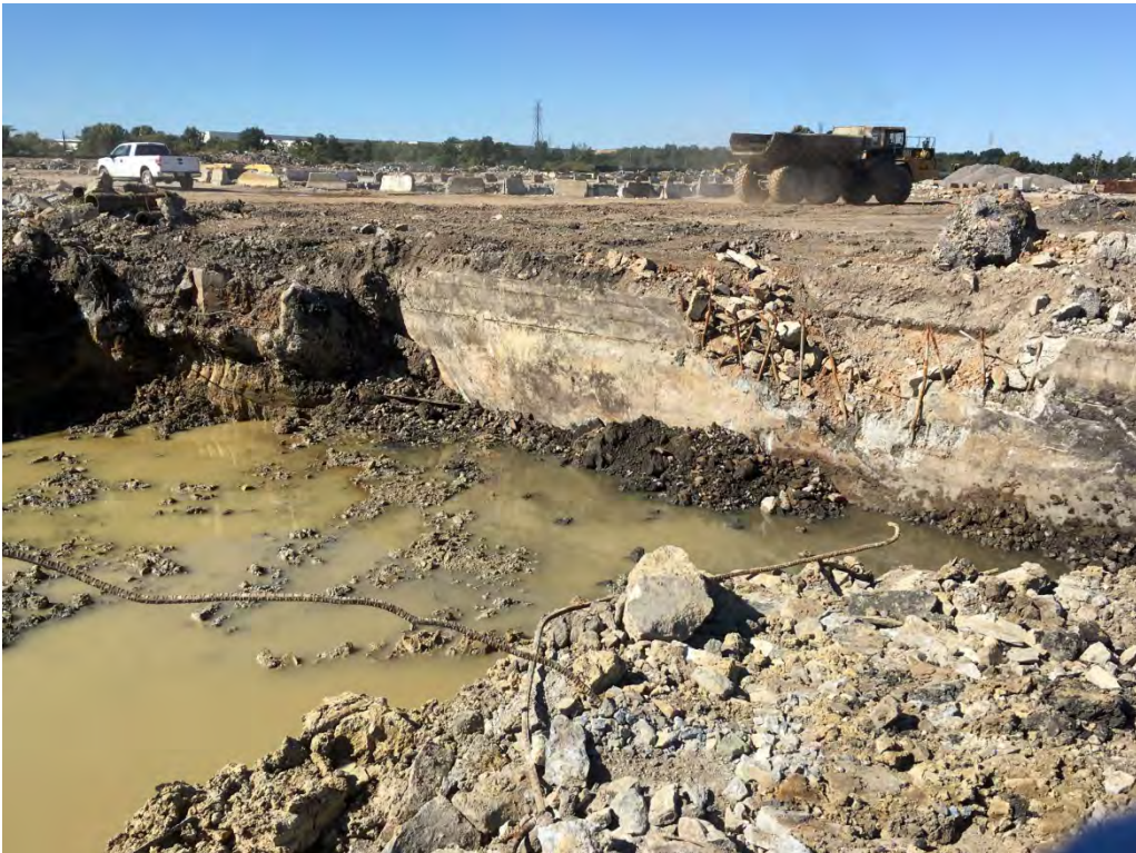
View of the north wall of the completed excavation.
