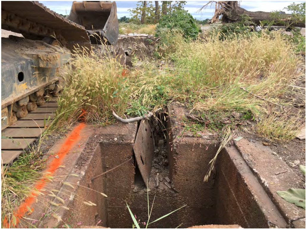
View of the french drain connected to the manhole facing north.
