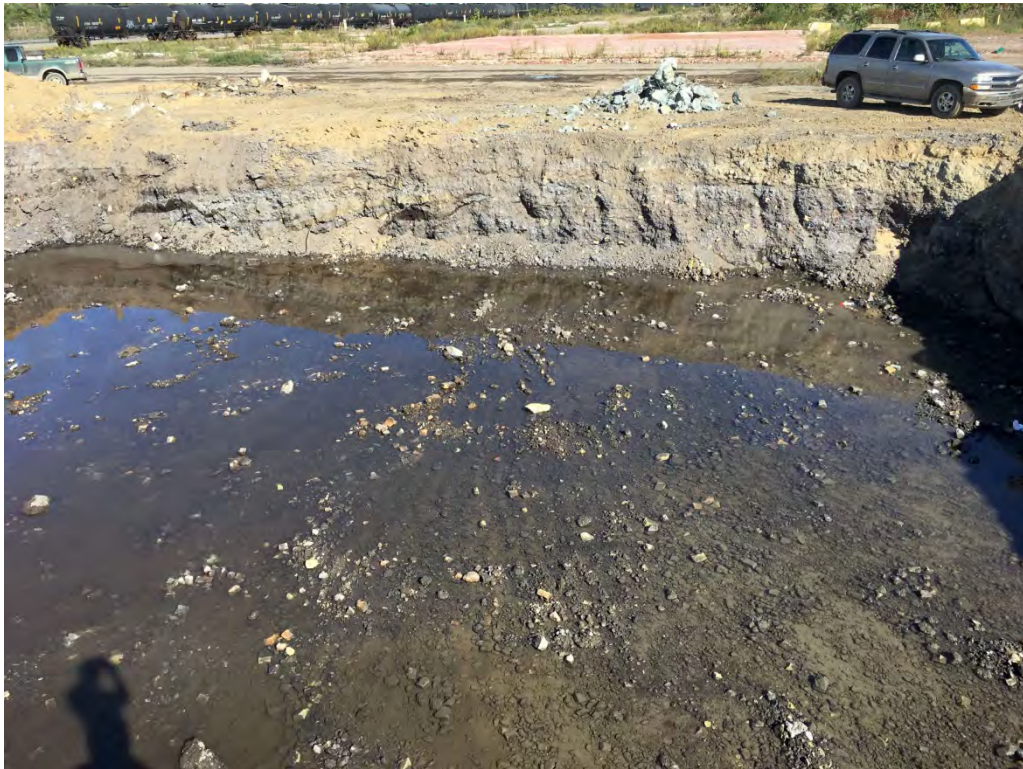
View of the east wall of the completed excavation facing east.
