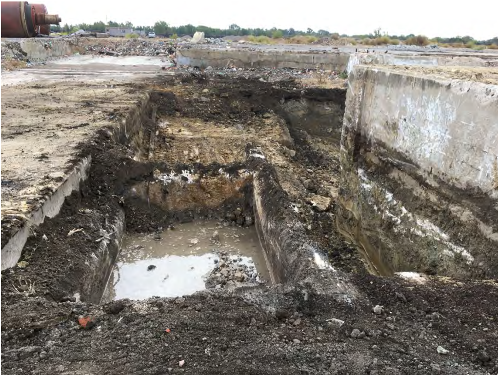
View of concrete box located in the northwest corner of the main excavated area. The benched area, approximately three feet below grade, is seen beyond the end of the concrete box.
