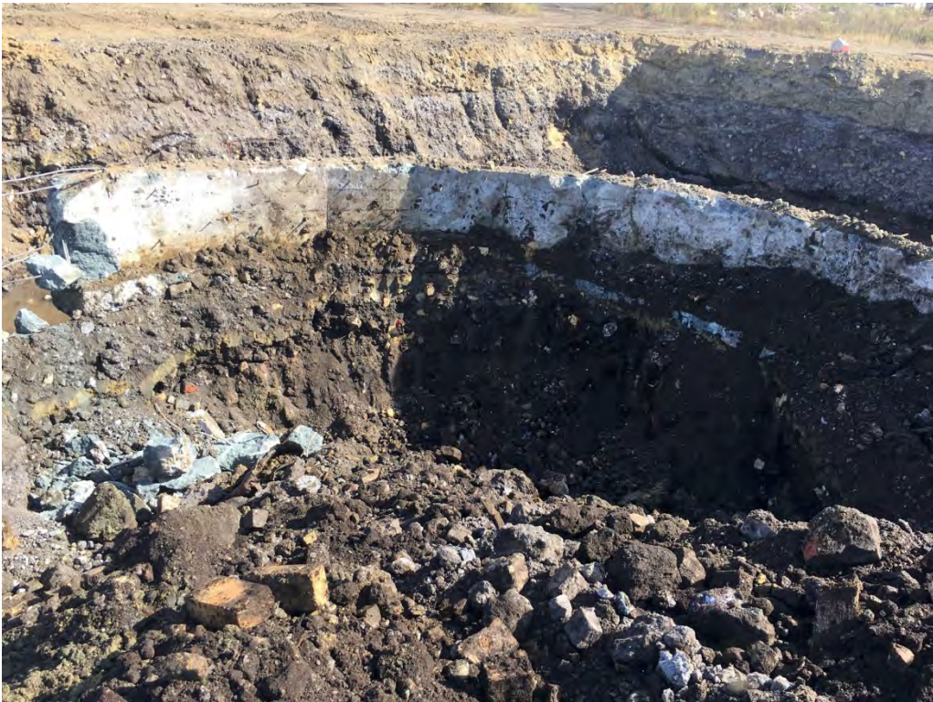
View of the material under the tank pad slag. Minor impacts were observed in this area. No impacts were observed on the tank's concrete pad and support ring.
