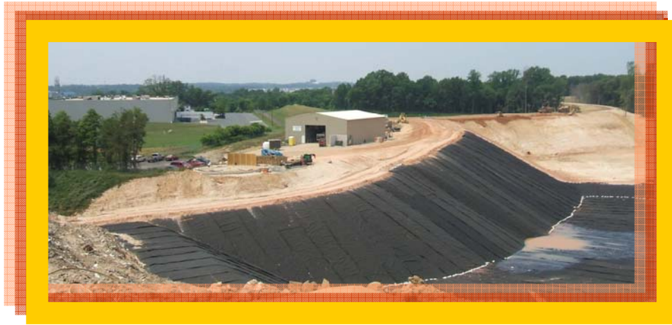
Rubble Landfill Liner Installation.
