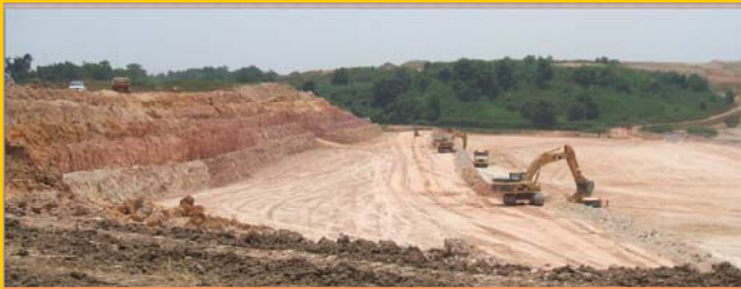
New cell under construction at Quarantine Road Landfill, Baltimore City
