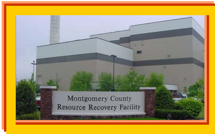
Montgomery County Resource Recovery Facility
