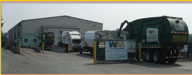
The largest processing and transferring facility in operation, Annapolis Junction Transfer Station, Jessup
