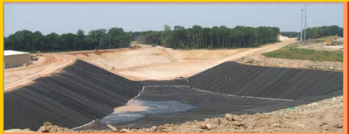
The construction of a new lined cell at Honeygo Rubble Landfill in White Marsh, Baltimore County
