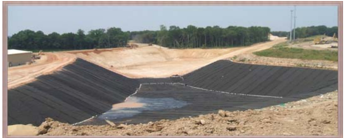
The construction of a new lined cell at Honeygo Rubble Landfill in White Marsh, Baltimore County
