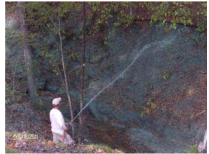
Ravine 3 - During Restoration
