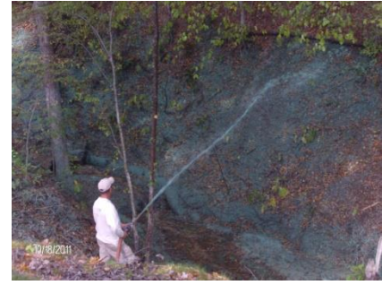
Ravine 3 - During Restoration
