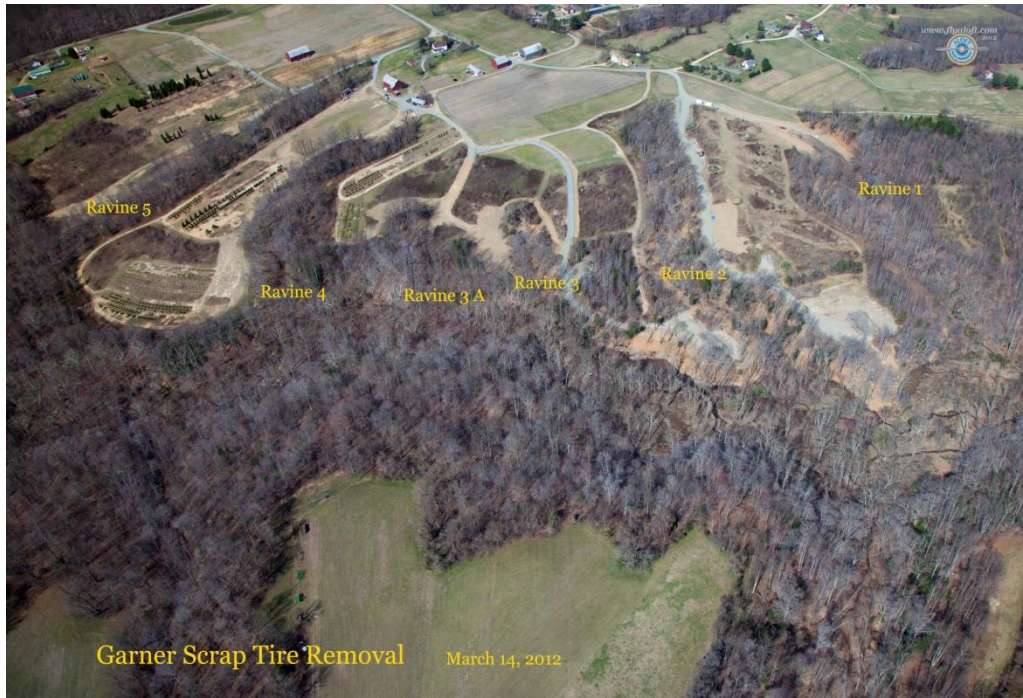
Aerial Photo of Entire Site During Cleanup
