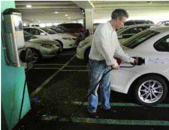
IMAGE 4. PARAMUS, NJ BY MOUNTING THE EVSE ON AN EXISTING POST BETWEEN SPACES, PARKING SPACE SIZES ARE MAINTAINED AND WHEEL STOPS OR BOLLARDS DO NOT NEED TO BE INSTALLED
