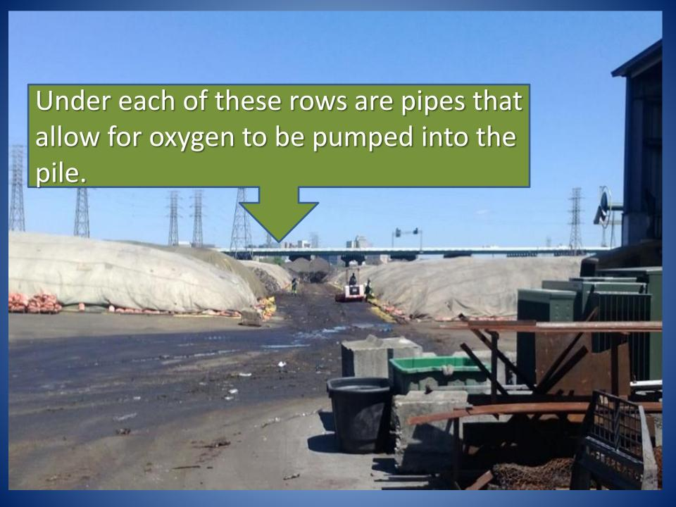
The Gore cover optimizes the breakdown process by trapping moisture and heat, while keeping out rain water
